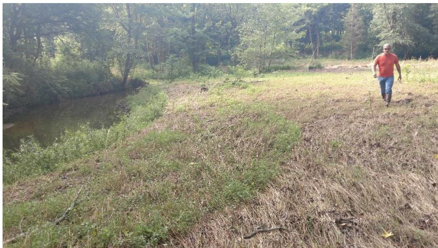
Evidence floodplain access in the form of preferential flow over grasses Mt. Pleasant Creek Restoration Project-Bowman Property
