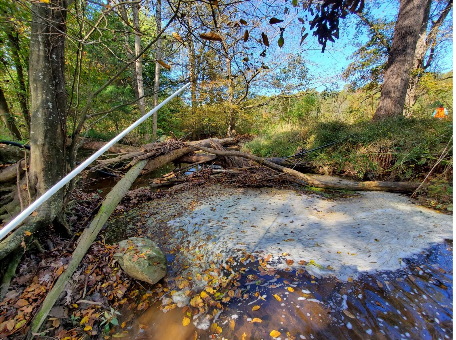
10/22/2020. Bankfull debris deposited in stream.
