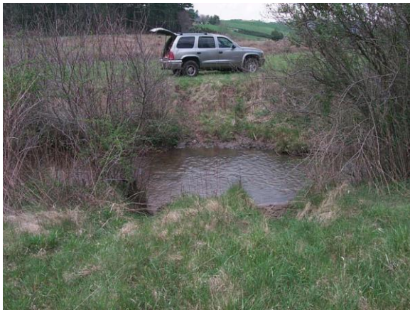
PS-9, bearing 310°: Pre-construction view of low water crossing at station 15+25; 17 Apr 02.
