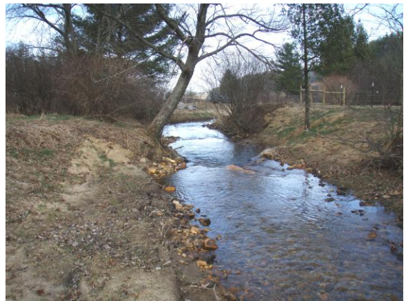
PS-4, bearing 335°: Post-construction view of cross-section 2 at station 6+39; 01 Jan 08.
