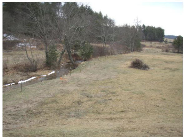
PS-2, bearing 315°: Post-construction view of station 3+00 to station 8+50; 29 Jan 08.
