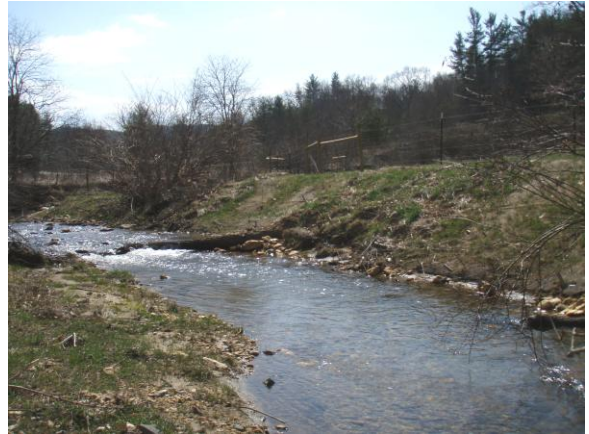
PS-1, bearing 230°: Post-construction view of station 1+75 to station 2+48; 26 Mar 08.
