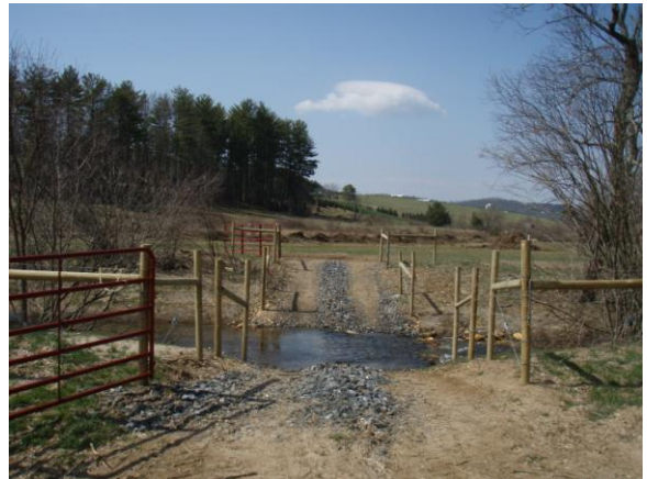
PS-9, bearing 310°: Post-construction view of low water crossing at station 15+25; 26 Mar 08.
