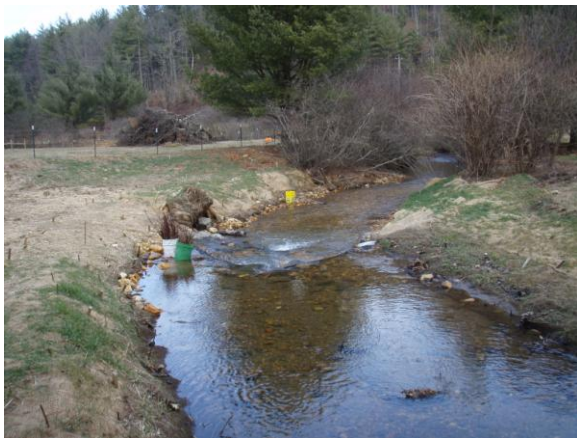
PS-6, bearing 18°: Post-construction view of cross-section 3 at station 7+62; 08 Jan 08.
