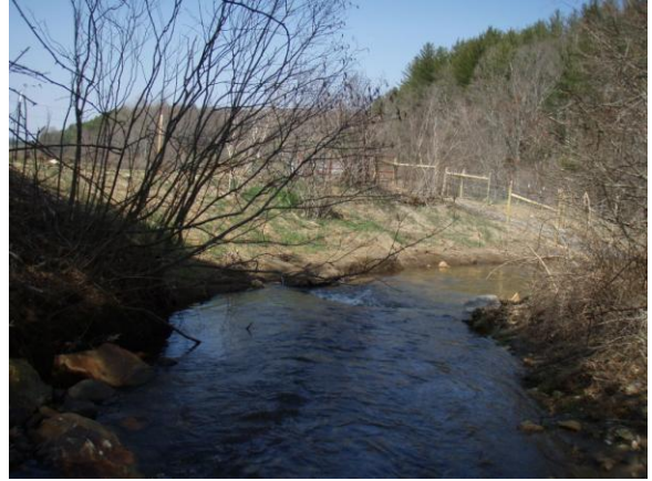
PS-8, bearing 350°: Post-construction view of cross-section 5 at station 14+80; 26 Mar 08.
