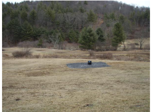
PS-15, bearing 80°: Post-construction view of station 16+50 to station 12+50; 29 Jan 08.
