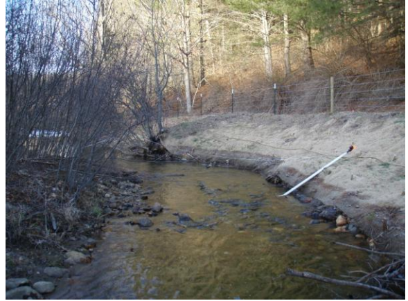
PS-11, bearing 20°: Post-construction view of cross-section 6 at station 20+90; 08 Jan 08.
