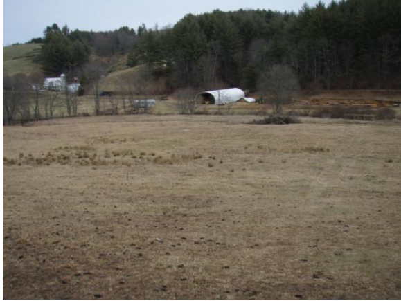
PS-14, bearing 50°: Post-construction view of station 23+00 to station 27+00; 29 Jan 08.
