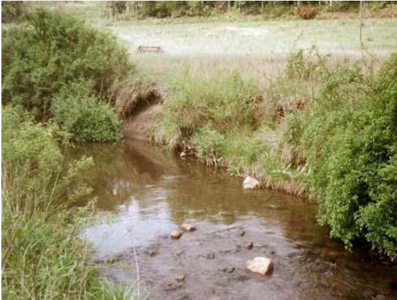
PS-1, bearing 230°: Pre-construction view of station 1+75 to station 2+48; 17 Apr 02.
