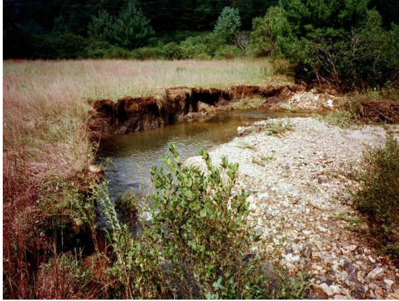
PS-5, bearing 35°: Pre-construction view of station 7+25 to station 8+50; 24 Sep 02.
