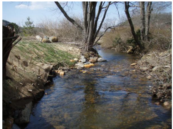
PS-13, bearing 330°: Post-construction view of station 21+50 to station 22+00; 26 Mar 08.
