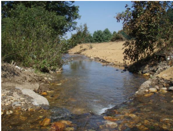
PS-3, bearing 330°: Post-construction view of cross-section 1 at station 3+56; 25 Sep 07.
