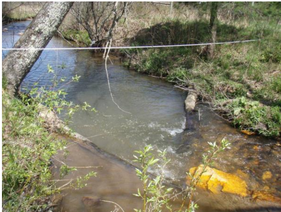
SPA MY5-1, piping under right vane arm, 9 Apr 12.
