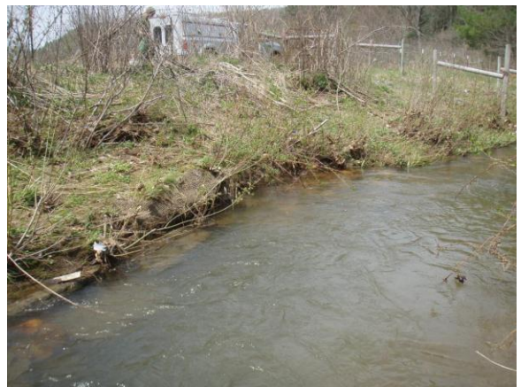
SPA MY4-5, repair of eroding left bank, 19 Apr 11.
