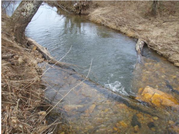
SPA MY4-2, piping under right vane arm, 3 Feb 11
