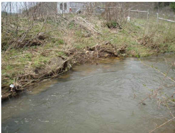
SPA MY4-5, eroding left bank, 19 Apr 11.
