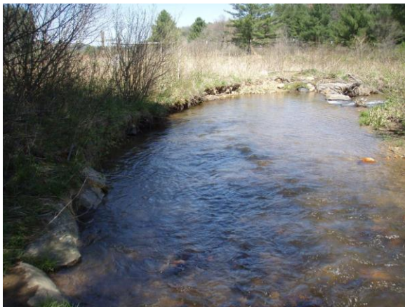
SPA MY5-2, eroding left bank, 9 Apr 12.
