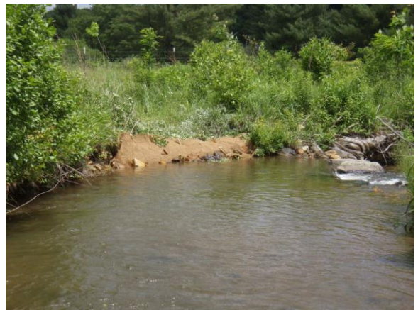
SPA MY5-2, repair of eroding left bank, 29 May 12
