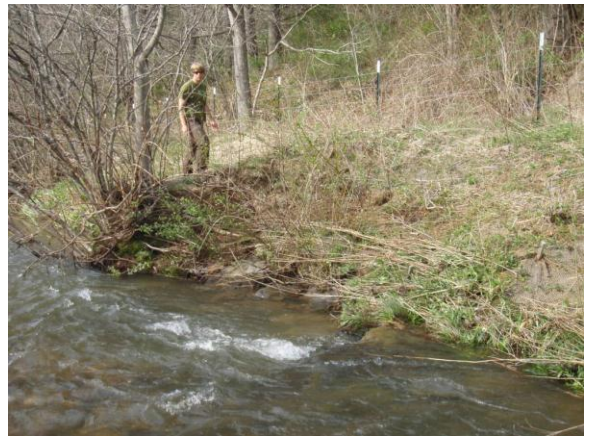
SPA MY4-6, repair of eroding right bank, 19 Apr 11.
