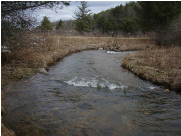
SPA MY3&4-3, eroding left bank: 14 Mar 10.
