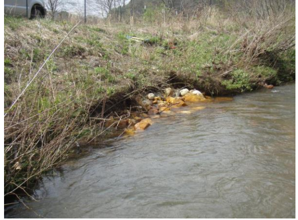
SPA MY4-7, repair of eroding left bank, 19 Apr 11.
