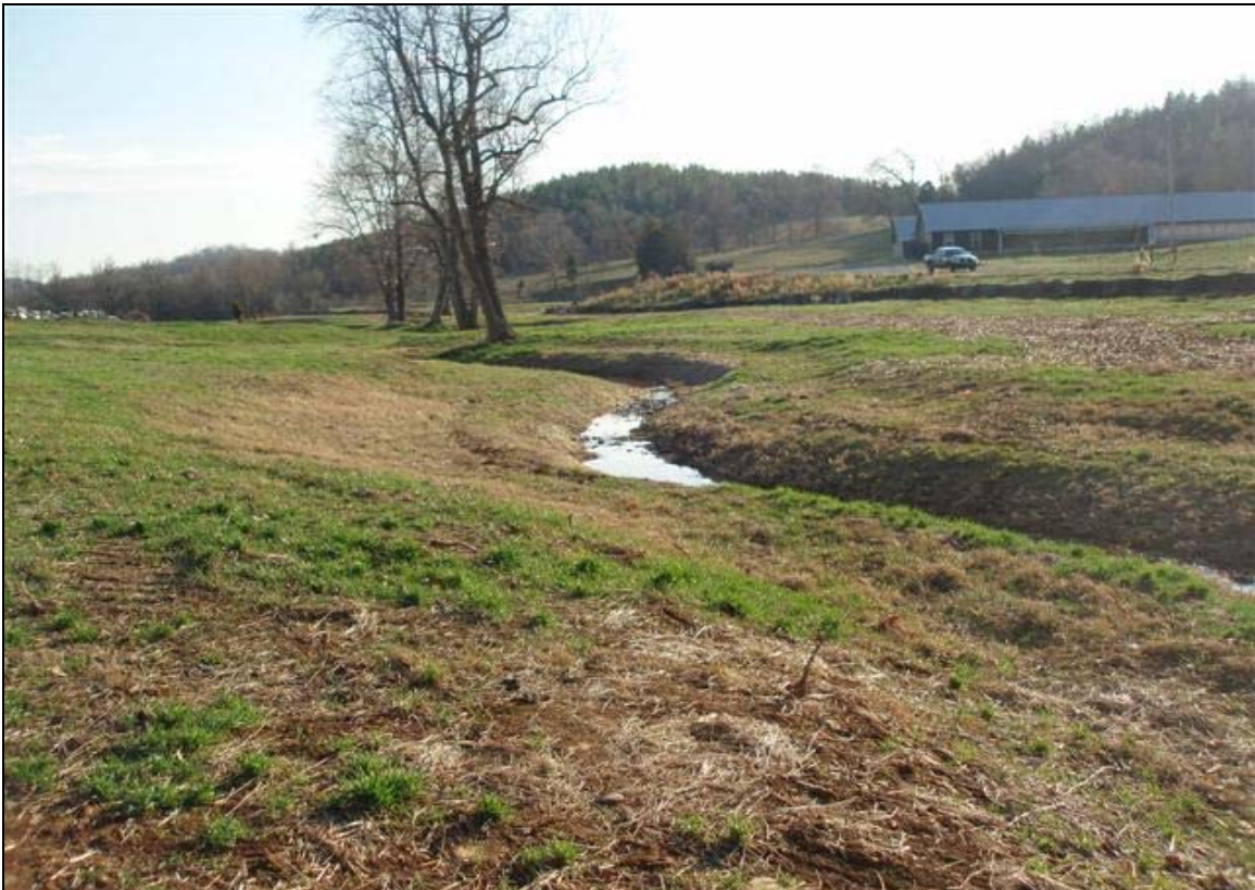
Photo Point 1b: View looking downstream near Station 11+50. 12/19/07 – As-Built
