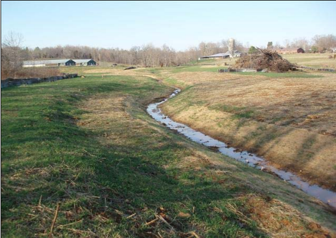
Photo Point 7a: View looking upstream near Station 27+25. 12/19/07 – As-Built
