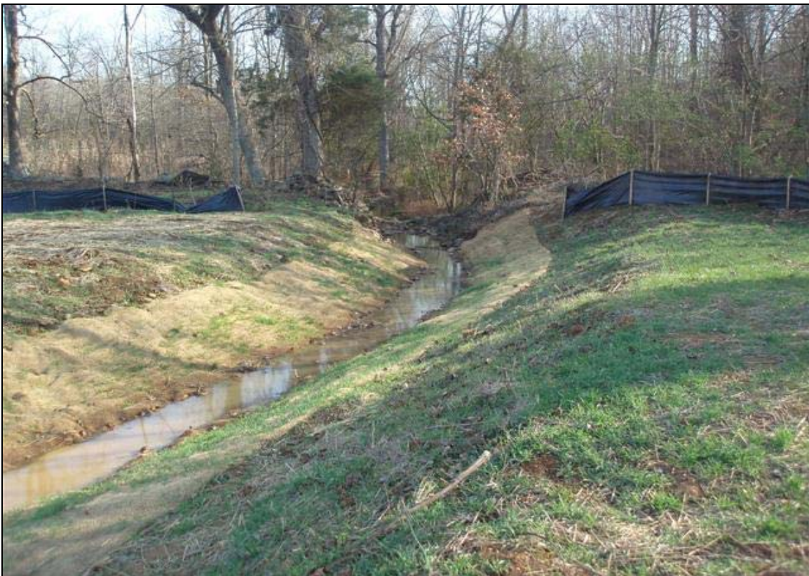
Photo Point 7b: View looking downstream towards end of project. 12/19/07 – As-Built
