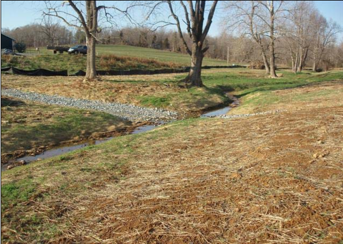
Photo Point 4a: View looking upstream near Station 18+00. 12/19/07 – As-Built
