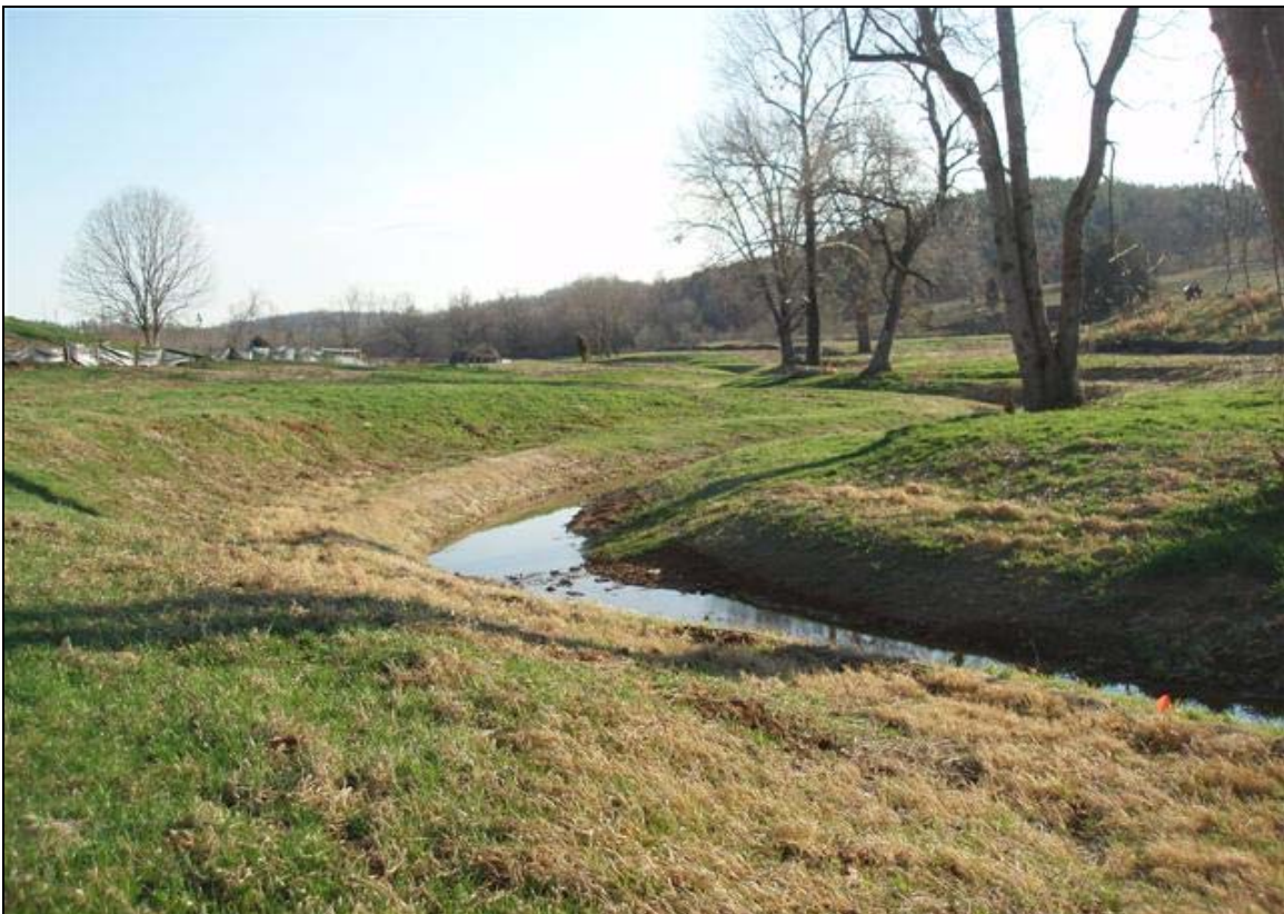
Photo Point 2b: View looking downstream taken near Station 13+10. 12/19/07 – As-Built
