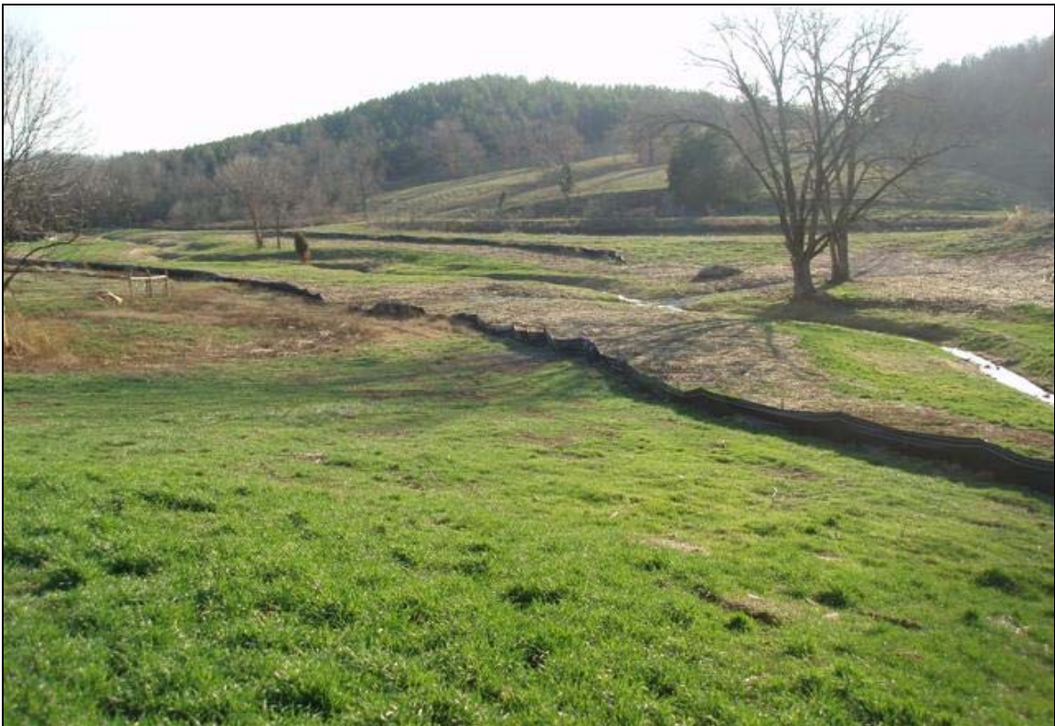
Photo Point 3b: View looking downstream from eastern side slope near Station 15+00. 12/19/07 – As-Built
