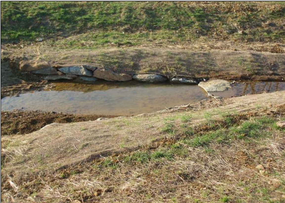
Photo Point 5b: View looking at cross vane near Station 21+00. 12/19/07 – As-Built
