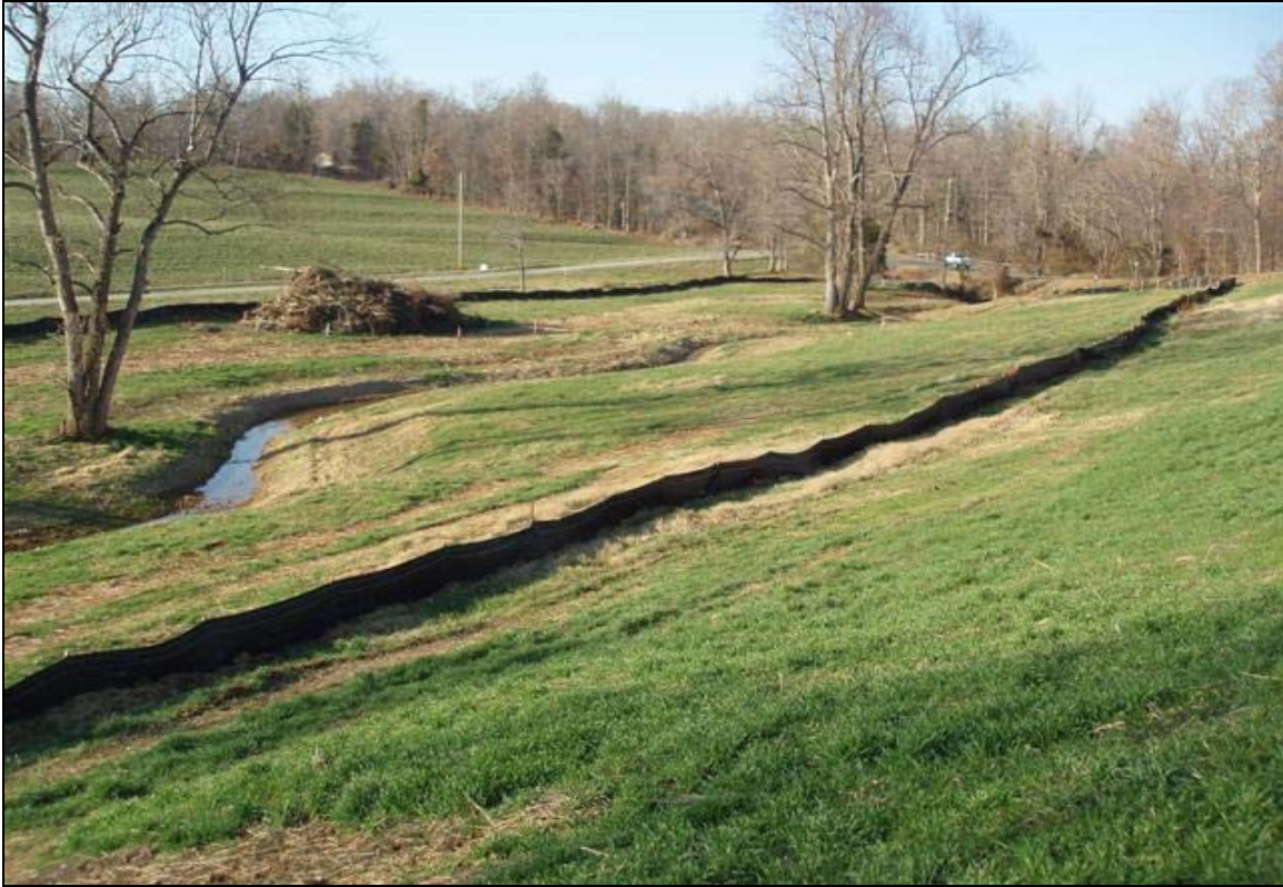
Photo Point 3a: View looking upstream from eastern side slope near Station 15+00. 12/19/07 – As-Built
