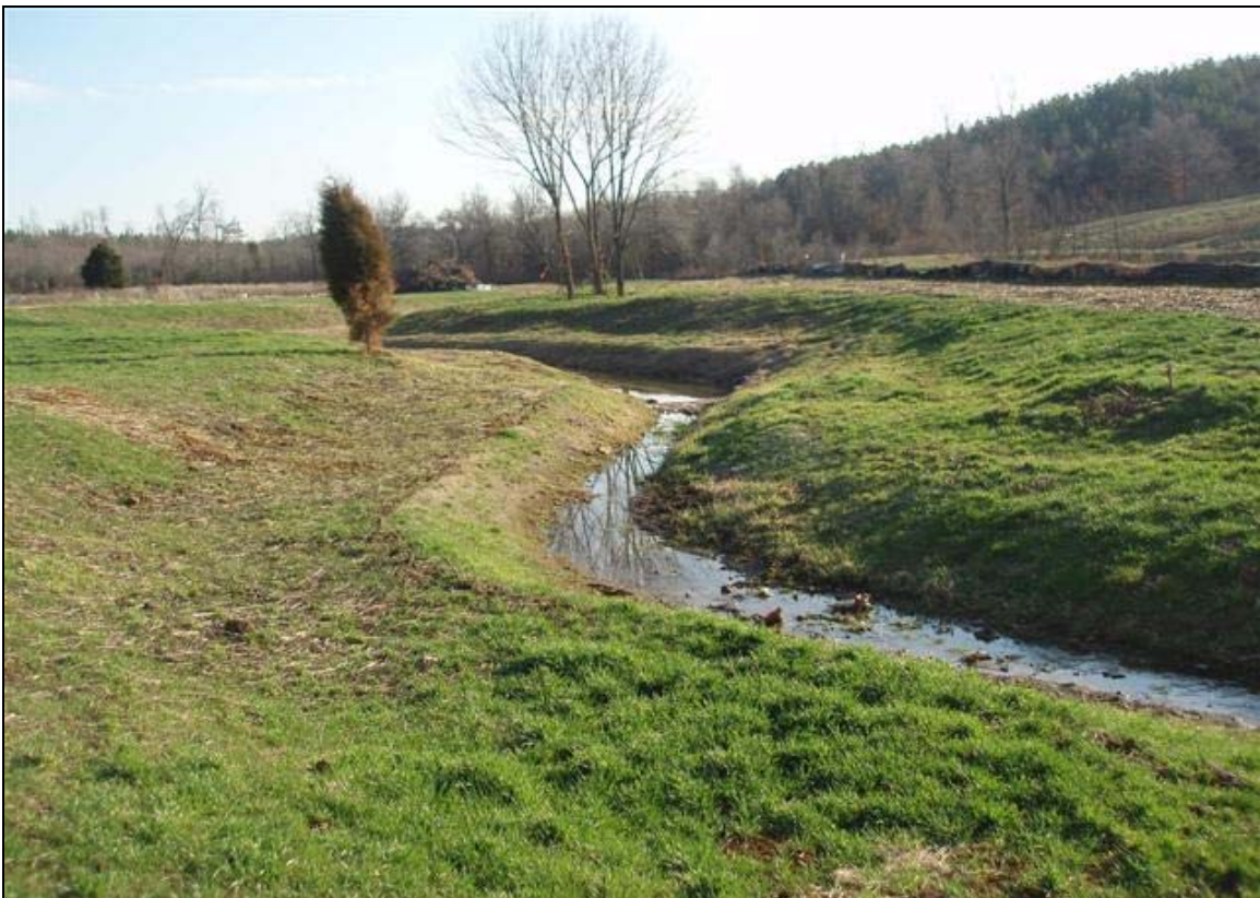
Photo Point 4b: View looking downstream near Station 18+00. 12/19/07 – As-Built
