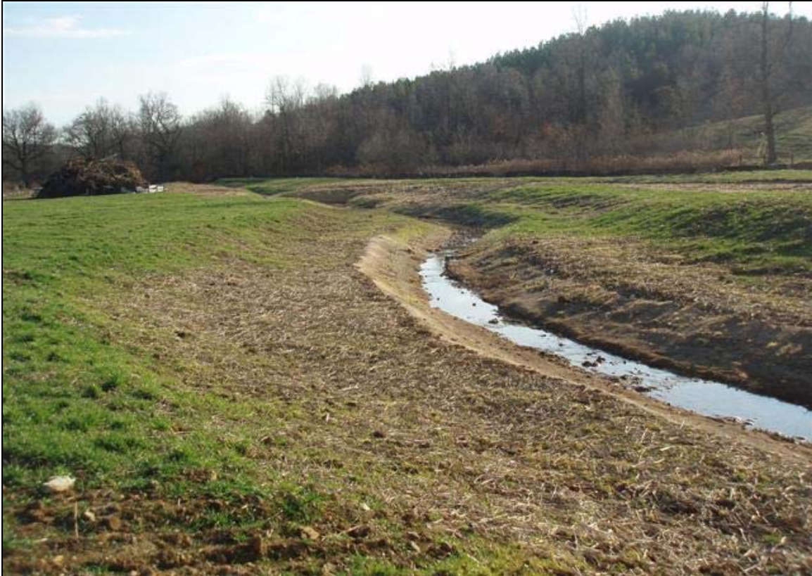
Photo Point 5c: View looking downstream near Station 21+00. 12/19/07 – As-Built
