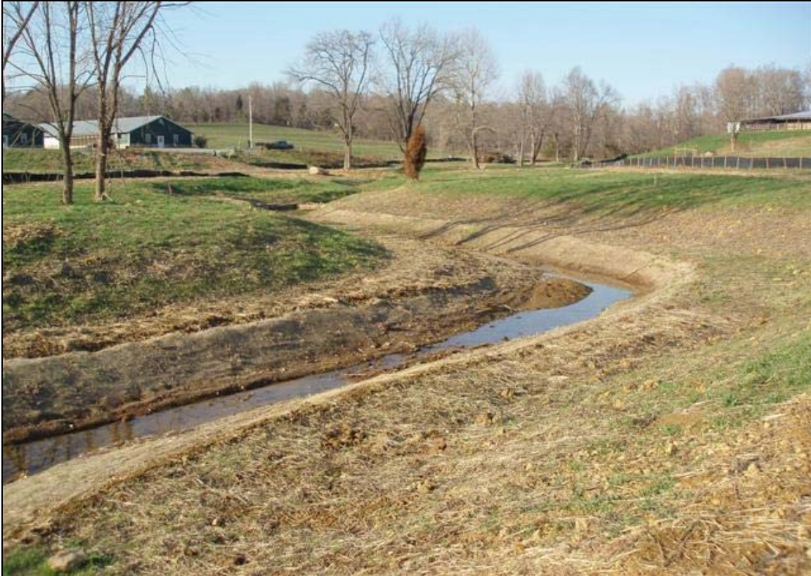
Photo Point 5a: View looking upstream near Station 21+00. 12/19/07 – As-Built
