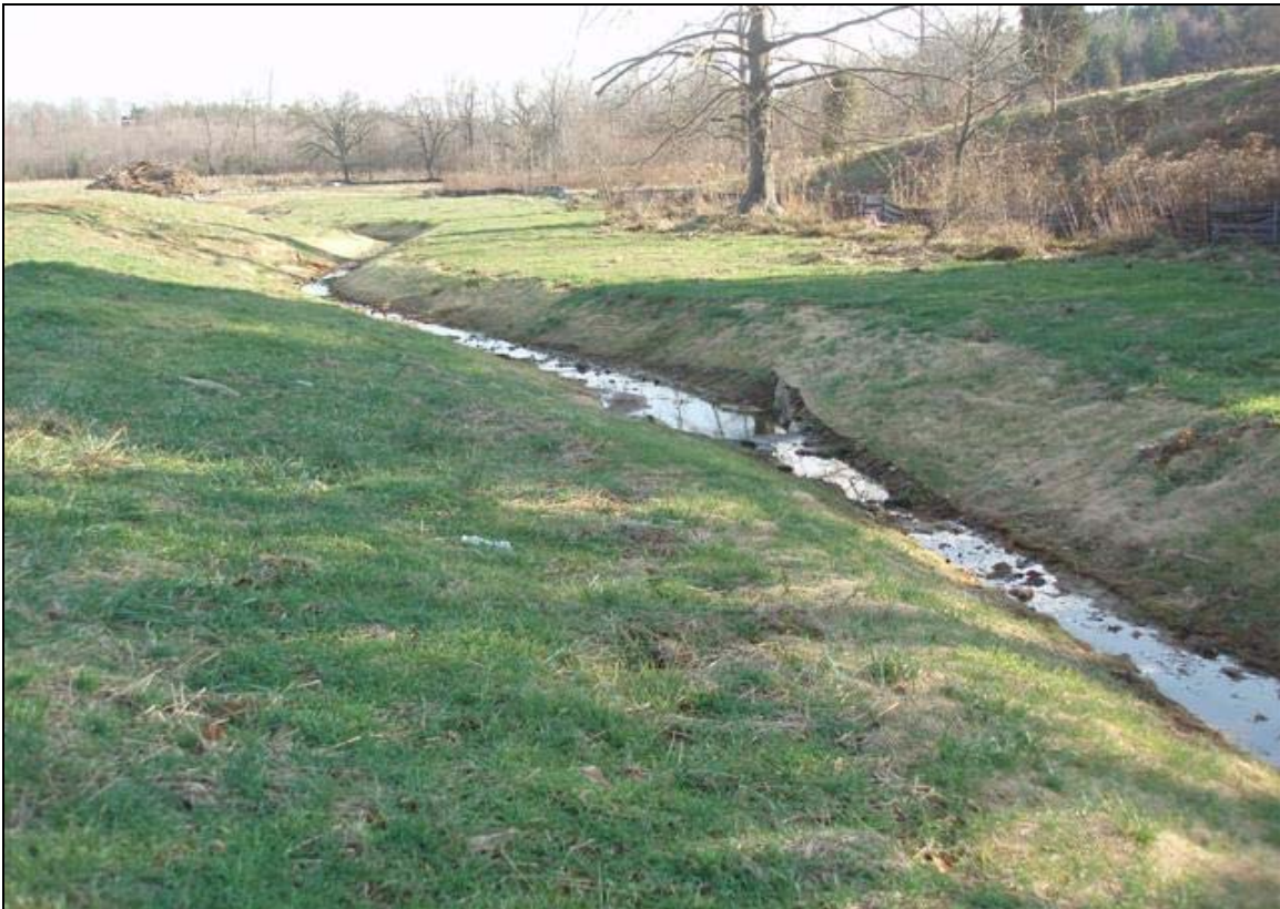
Photo Point 9b: View looking downstream on tributary near Station 53+15. 12/19/07 – As-Built
