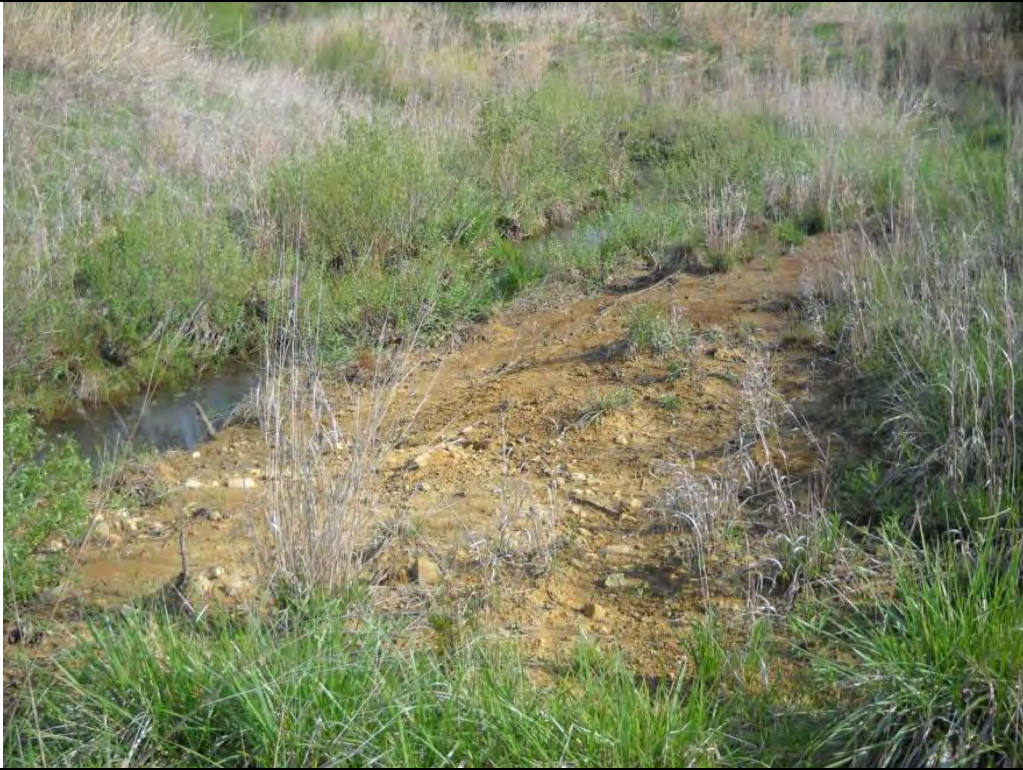
VP3: Bare bench on Reach UTJC1 (STA 20+00) Taken: April 2011
