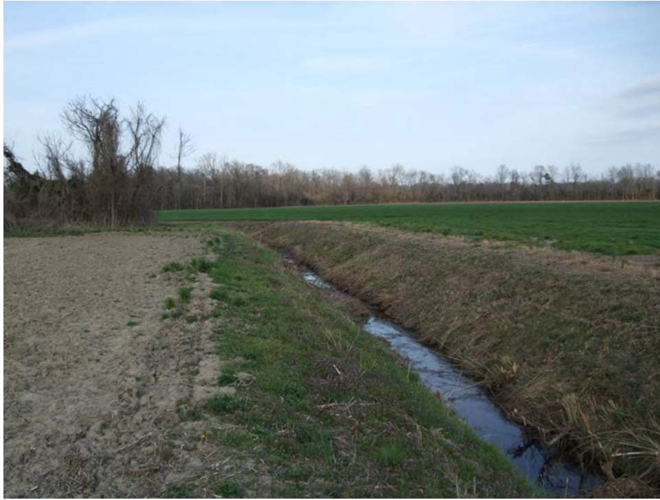
Photo B1 – Pre-construction stream channel looking downstream near station 14+00 (3/10/09)
