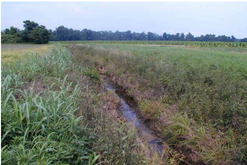
Photo 4. Existing Channel; Middle Reach Facing North Looking Downstream Showing Mowed Buffer
