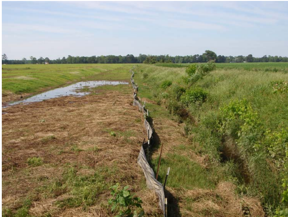
Photo B8 – Evidence of bankfull flow (wrack lines of straw and sediment on plants). Lower end of stream enhancement looking upstream (5/13/2009 Year 0)
