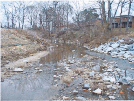
Reach 1 Downstream of Culvert at W. Meadowview
