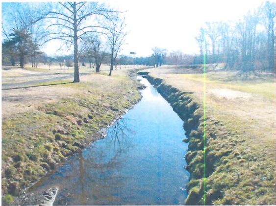
Upstream Section on Golf Course
