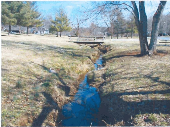
Upstream of Foot Bridge
