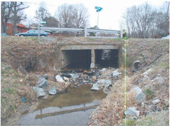
Culvert Downstream of S. Benbow Rd.
