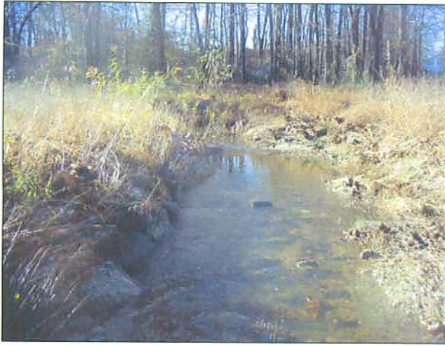
PP#31B R2 Constructed Riffle #3, Rock Vane #4, and Cross Section #4
