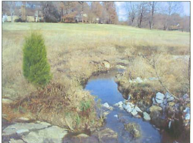
PP26 Root Wad Cluster #5 with toe protection
