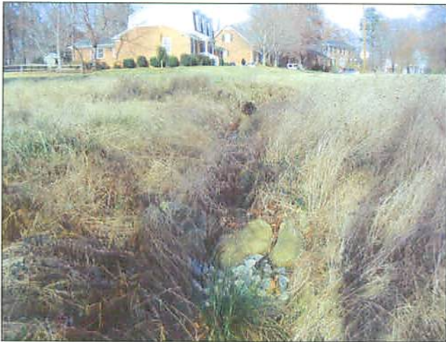
PP20B Swale into Step Pool #2
