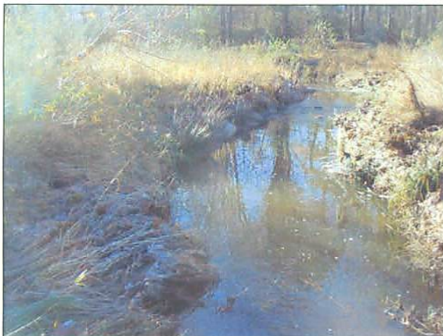
PP#30 R2 Rock Vane #4 and Constructed Riffle #3
