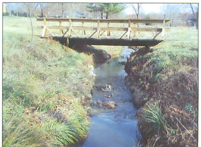
PP18 Riffle #8 and Pedestrian Footbridge
