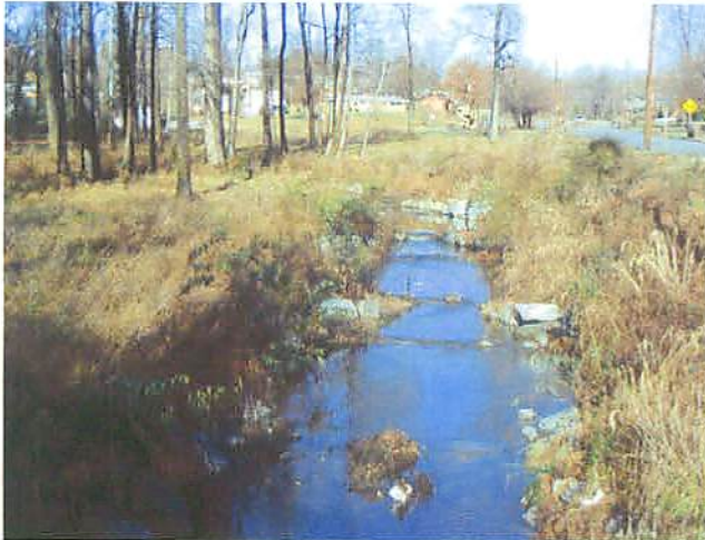
PP#44 R2 Upstream view from Belcrest Road at end of R2
