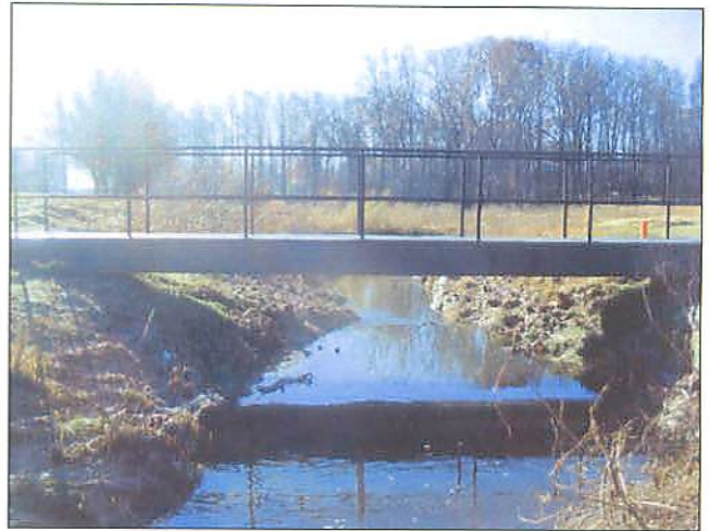
PP#22 R2 Newly Installed Pedestrian Bridge
