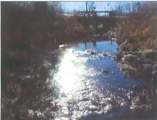
PP#14 R1 Constructed Riffle #4
