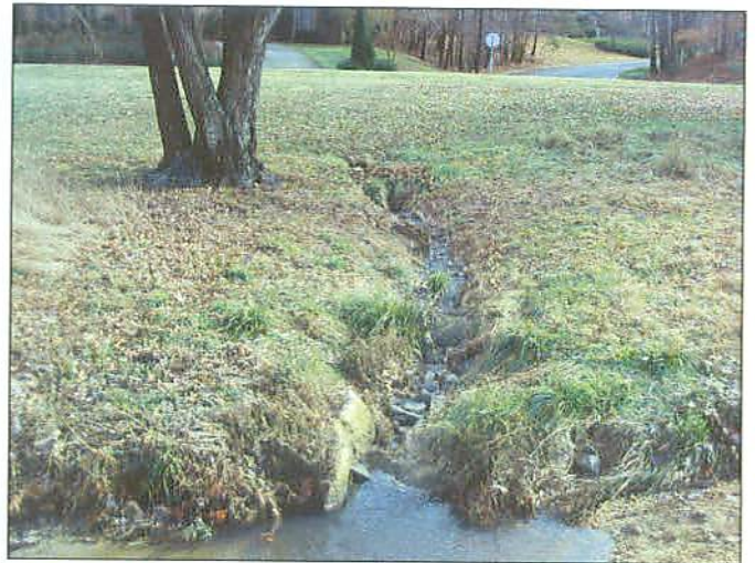
PP#31 Swale into Step Pool #7
