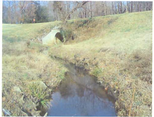
PP#41 Root Wad Cluster #16 into Culvert at Reach End
