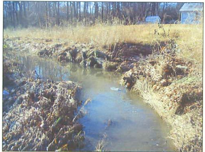
PP#27 R2 Rock Vane #3, Step pool #2, and Root Wad Cluster #2
