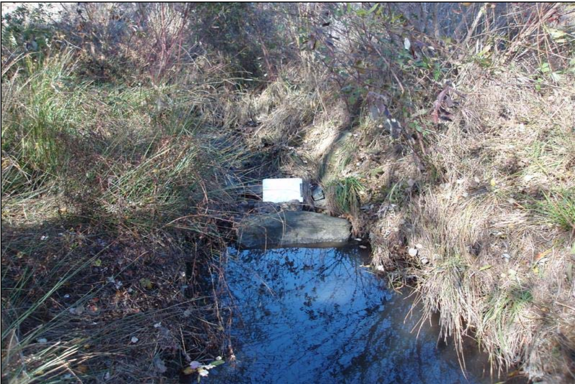
SP2 – Base flow going around a header stone in cross vane. Photo taken near Station 19+20. 11/19/07 - MY 03
