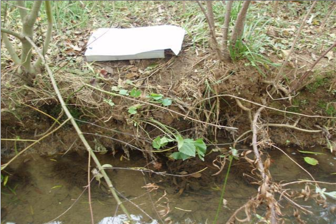
SP3 – Bank erosion. Photo taken near Station 31+50. 10/29/08 - MY 04
