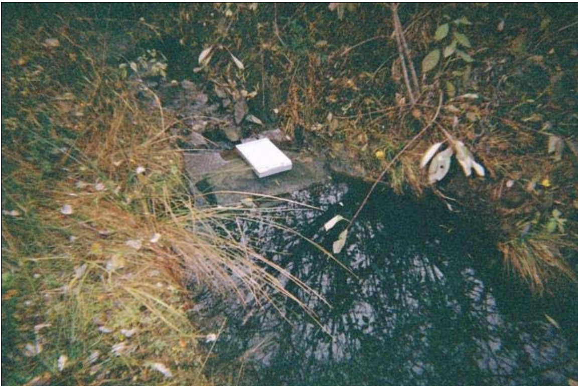
SP2 – Base flow going around a header stone in cross vane. Photo taken near Station 19+20. 11/5/08 - MY 04
