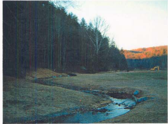
Photo Station #16. Looking downstream from as-built Station ~14+25.
