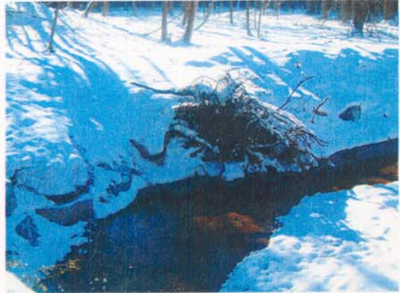
Photograph NM-8. Looking downstream at rootwad and rock toe protection from pedestrian bridge at as-built Station ~44+60.
