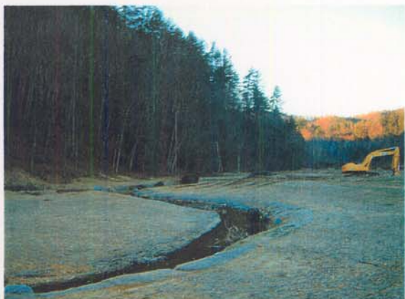
Photo Station #19. Looking downstream from as-built Station ~8+30.
