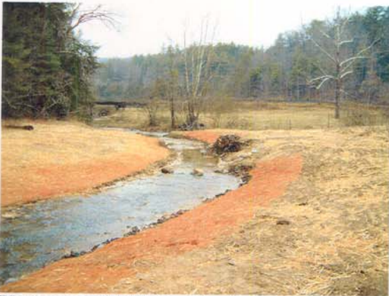
Photograph NM-73. Looking downstream at rock "J" vane and rootwad from as-built Station ~1+00.
