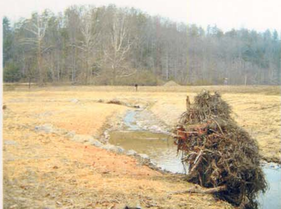
Photograph NM-61. Looking downstream at rootwads and rock toe protection from as-built Station ~6+50.
