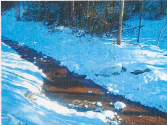
Photograph NM-7. Looking upstream at cross vane from as-built Station ~44+80.
