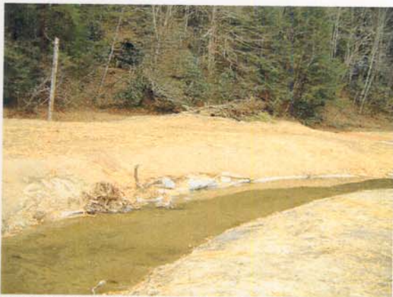
Photograph NM-67. Looking downstream at rootwad from as-built Station ~4+00.
