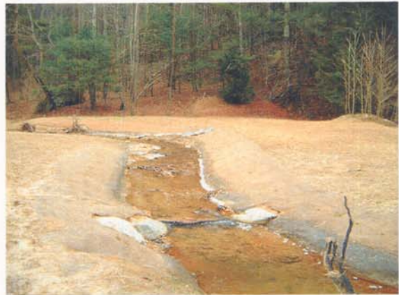
Photograph NM-52. Looking upstream at rock vane and rootwads from as-built Station ~8+75.
