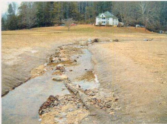
Photograph NM-57. Looking upstream at log vane from as-built Station ~7+00.
