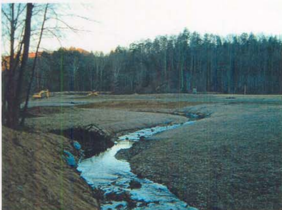
Photo Station #17. Looking downstream from as-built Station ~12+50. Tributary confluence to left.
