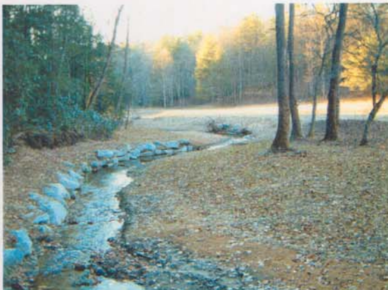
Photo Station #5. Looking downstream from as-built Station ~41+25.
