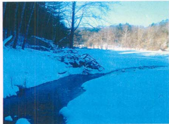
Photograph NM-46. Looking downstream at rootwads from as-built Station ~12+25.
