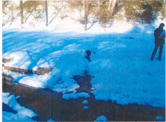
Photograph NM-26. Looking downstream at log toe protection from as-built Station ~30+85.
