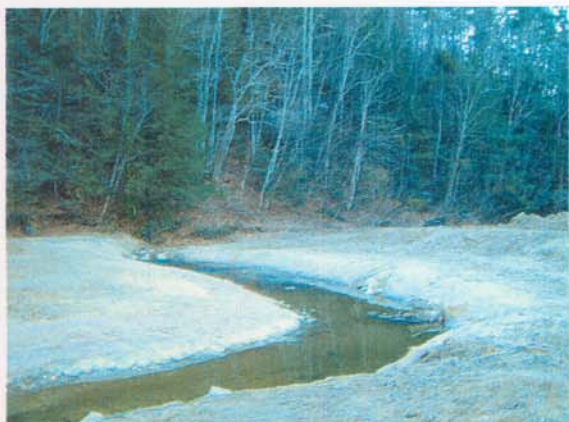
Photo Station #21. Looking downstream from as-built Station ~3+25.
