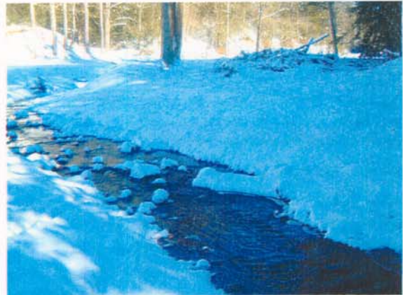
Photograph NM-32. Looking downstream at log vane from as-built Station ~23+30.
