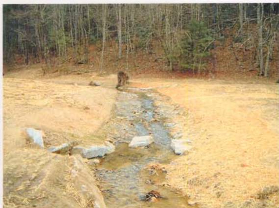
Photograph NM-63. Looking upstream at rock "J" vane from as-built Station ~5+25.
