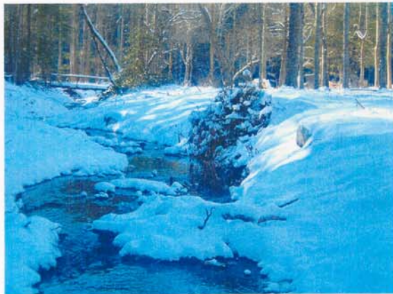
Photograph NM-6. Looking downstream at log vane from as-built Station ~47+25.
