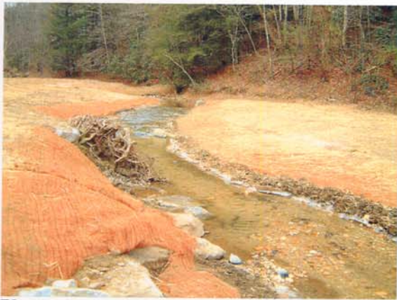
Photograph NM-75. Looking upstream at rock vane and rootwad from as-built Station ~0+65.
