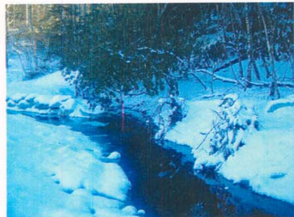
Photograph NM-36. Looking upstream at rootwads and rock toe protection from as-built Station ~20+00.
