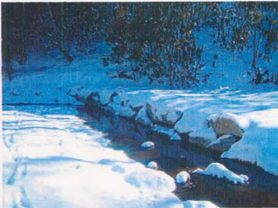
Photograph NM-33. Looking upstream at rock toe protection from as-built Station ~23+00.
