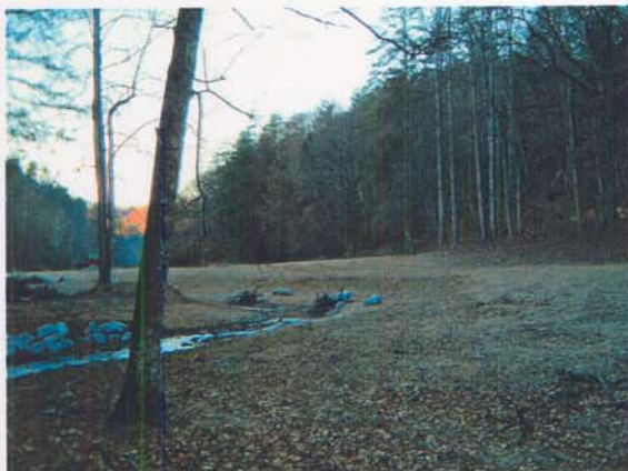
Photo Station #11. Looking downstream from as-built Station ~25+85.
