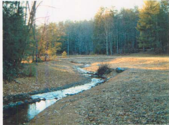
Photo Station #6. Looking downstream from as-built Station ~38+00.
