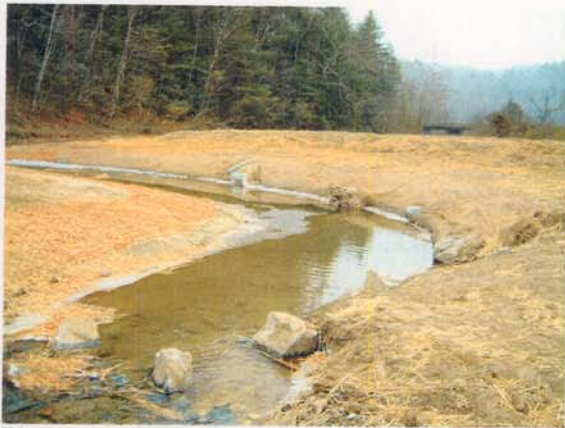
Photograph NM-69. Looking downstream at rock "J" vane from as-built Station ~3+25.
