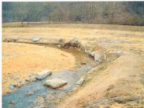
Photograph NM-62. Looking downstream at rock "J" vane, rock toe protection, and rootwad from as-built Station ~5+50.
