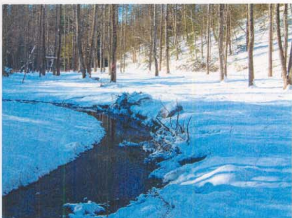
Photograph NM-3. Looking downstream at rootwads and log toe protection from as-built Station ~49+25.
