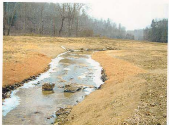
Photograph NM-72. Looking upstream at rock "J" vane from as-built Station ~2+00.
