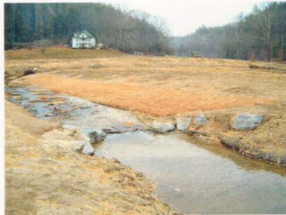
Photograph NM-66. Looking upstream at cross vane from as-built Station ~4+00.
