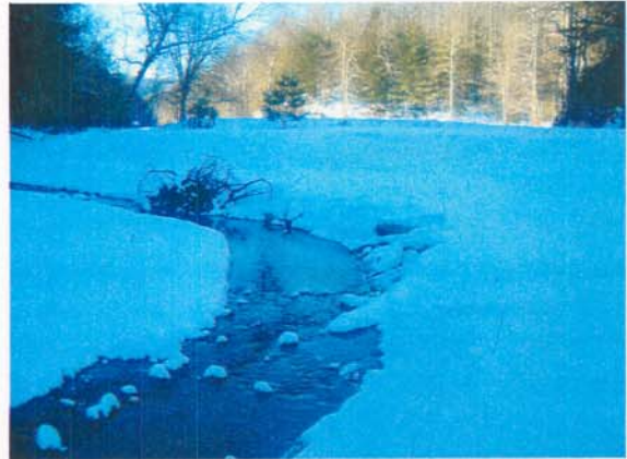
Photograph NM-20. Looking downstream at log vane, rootwad, and log toe protection from as-built Station ~36+25.
