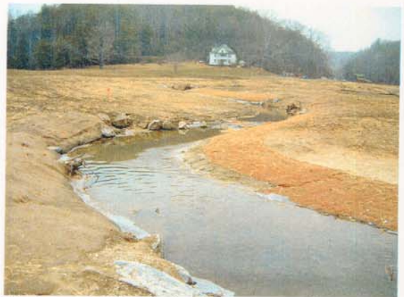
Photograph NM-70. Looking upstream from as-built Station ~2+75.
