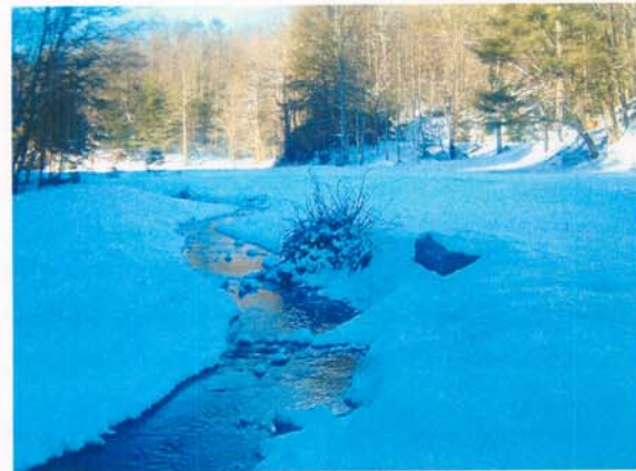
Photograph NM-18. Looking downstream at log vane and rootwads from as-built Station 37+75.
