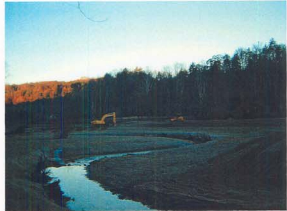
Photo Station #18. Looking downstream from as-built Station ~10+05.
