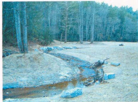
Photo Station #12. Looking downstream from as-built Station ~24+50.
