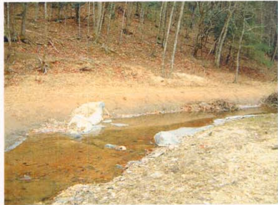
Photograph NM-58. Looking downstream at rock "J" vane from as-built Station ~6+80.
