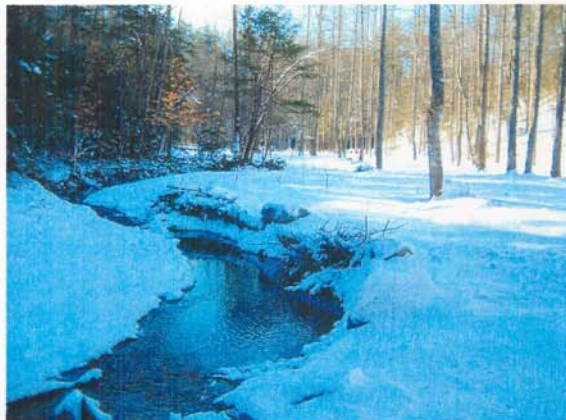
Photograph NM-2. Looking downstream at rootwads and log toe protection from as-built Station ~51+00.
