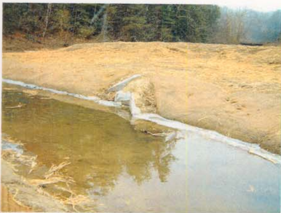
Photograph NM-71. Looking downstream at rock vane from as-built Station ~2+75.
