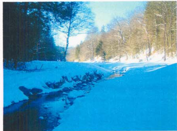
Photograph NM-24. Looking downstream at rock toe protection from as-built Station ~32+00.
