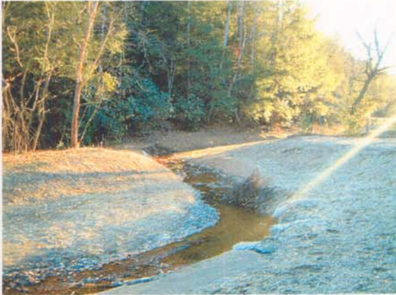
Photo Station #7. Looking downstream from as-built Station ~36+10.
