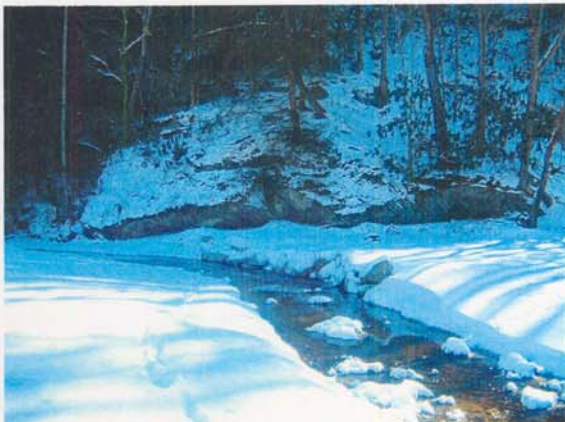
Photograph NM-41. Looking upstream at rock toe protection from as-built Station ~14+50.
