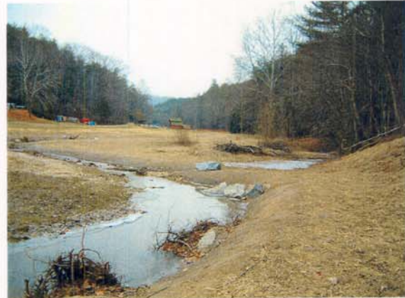
Photograph NM-60. Looking upstream at rock "J" vane and wetland from as-built Station ~ 6+50.
