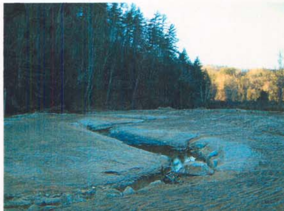
Photo Station #20. Looking downstream from as-built Station ~5+05.
