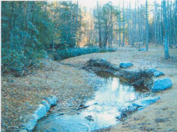
Photo Station #1. Looking downstream from as-built Station ~51+00.
