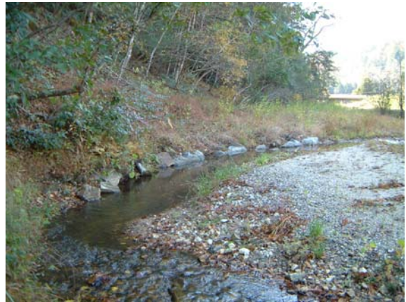
Looking downstream at rock wall at as-built Station ~1+50.
