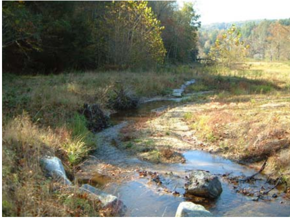
Photograph NM-49. Looking downstream at rootwads and rock vane from as-built Station ~10+00.
