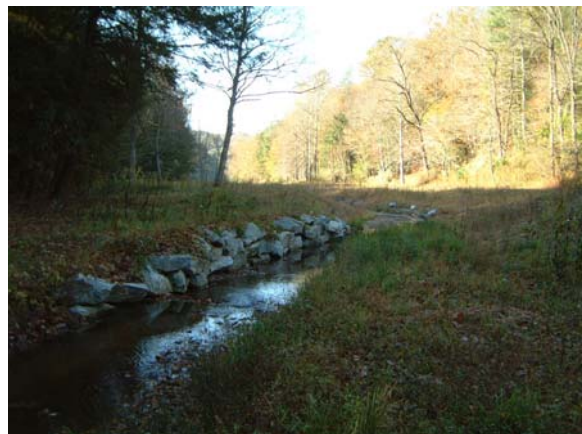
Photograph NM-24. Looking downstream at channel plug protection from as-built Station ~32+00.
