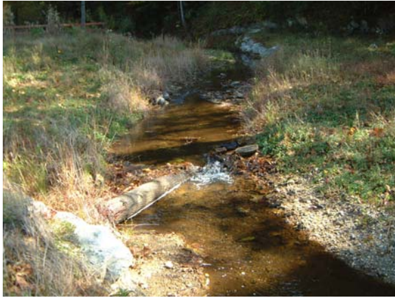
Photograph NM-43. Looking upstream at log vane from as-built Station ~14+00.
