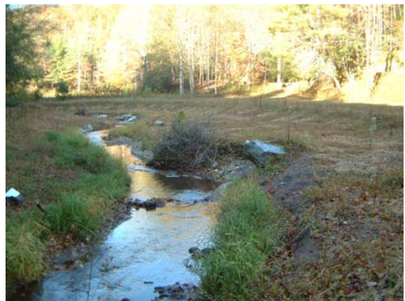
Photograph NM-18. Looking downstream at log vane and rootwads from as-built Station 37+75.
