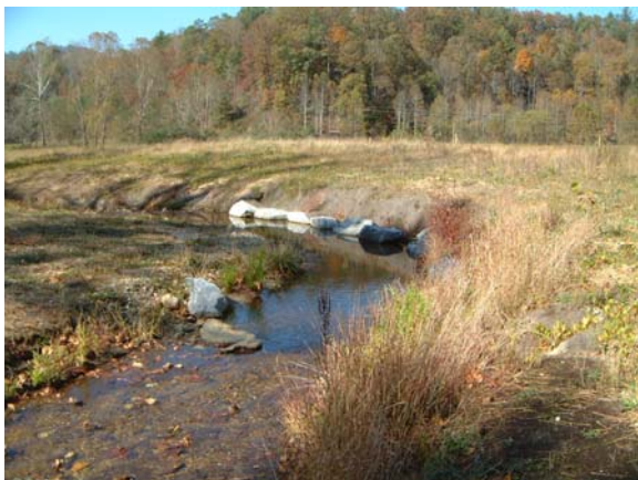
Photograph NM-47. Looking downstream at rock cross vane from as-built Station ~11+30.
