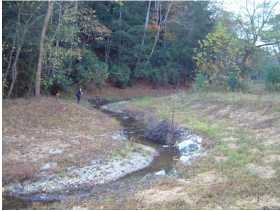
Photo Station #7. Looking downstream from as-built Station ~36+10.
