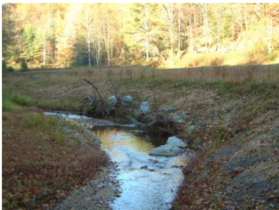
Photograph NM-17. Looking downstream at rock vane, rootwads, and log toe protection from as-built Station ~39+75.
