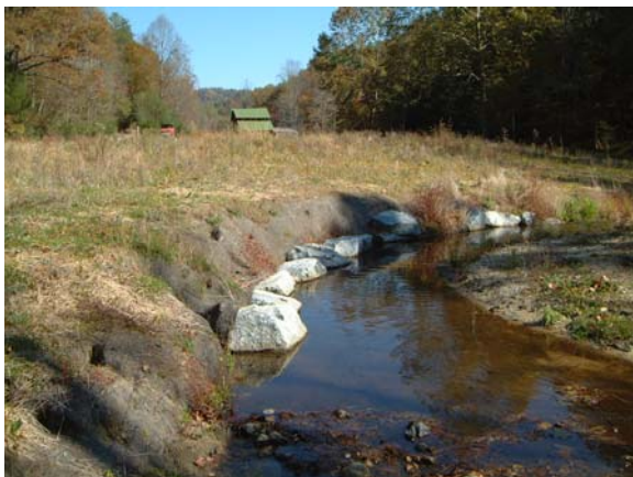
Looking upstream at rolled rocks at as-built Station ~11+00.
