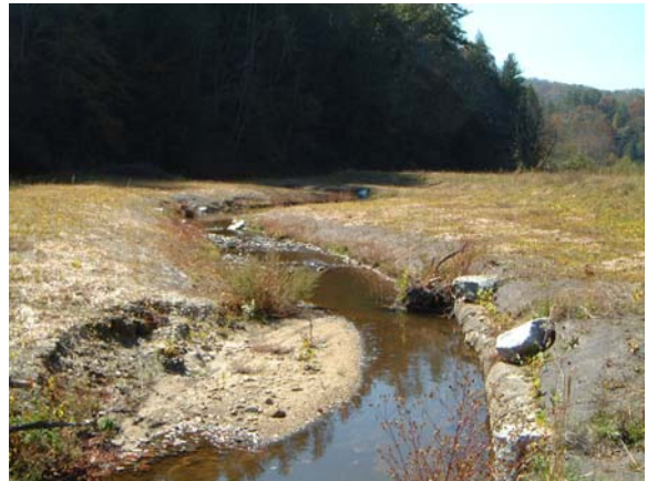
Photograph NM-64. Looking downstream at log toe protection and rootwad from as-built Station ~5+25.
