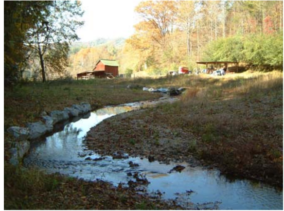
Photograph NM-38. Looking downstream at channel plug protection from as-built Station ~19+00.
