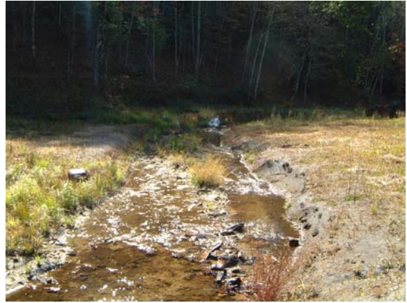
Photograph NM-56. Looking downstream along riffle from as-built Station ~8+00.
