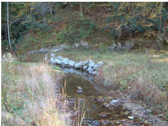
Photograph NM-41. Looking upstream at channel plug protection from as-built Station ~14+50.
