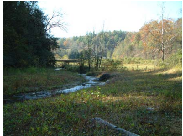
Photo Station #22. Looking downstream from as-built Station 1+60.
