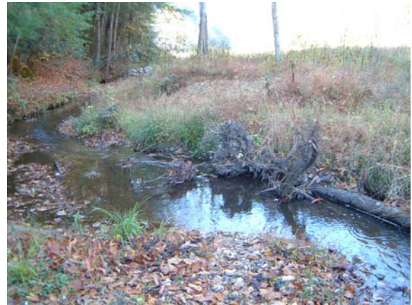
Looking downstream at good pool and rootwad from as-built Station ~26+50.
