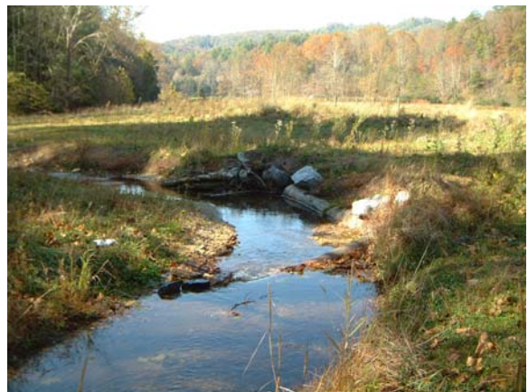
Photograph NM-42. Looking downstream at log vane from as-built Station ~14+25.
