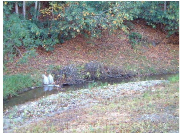
Looking downstream at rootwads from as-built Station ~35+00.
