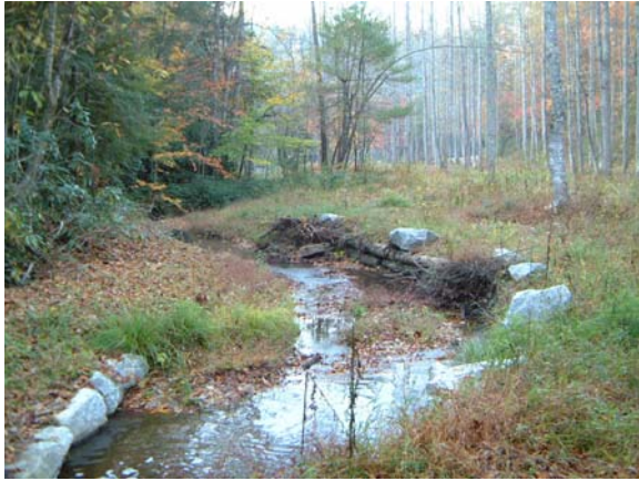
Photo Station #1. Looking downstream from as-built Station ~51+00.
