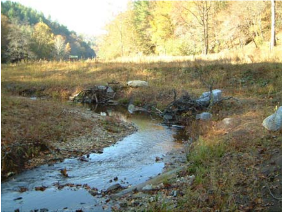
Photograph NM-31. Looking downstream at log vane and rootwads from as-built Station 24+60.
