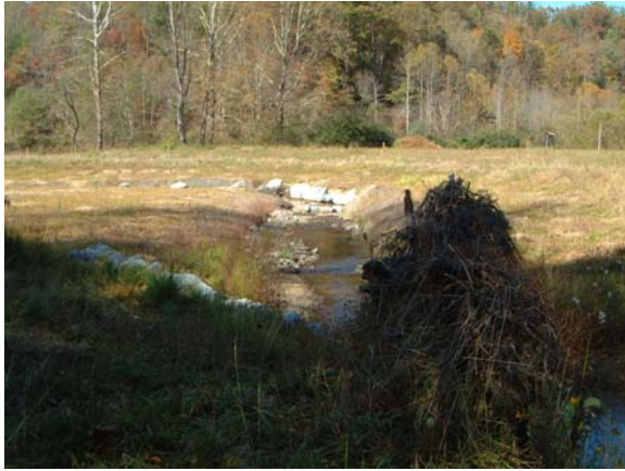
Photograph NM-61. Looking downstream at rootwads and rock toe protection from as-built Station ~6+50.
