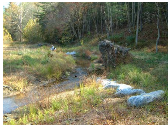
Looking upstream at rock vane and root wads from as-built Station ~6+50.
