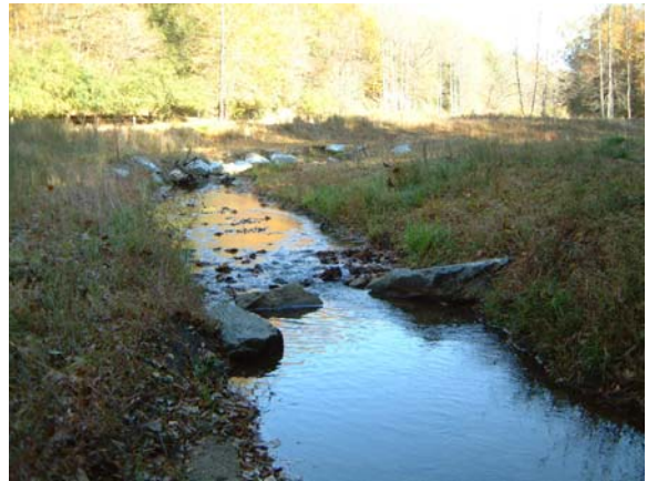
Photograph NM-40. Looking upstream at rock "J" vane from as-built Station ~16+00.
