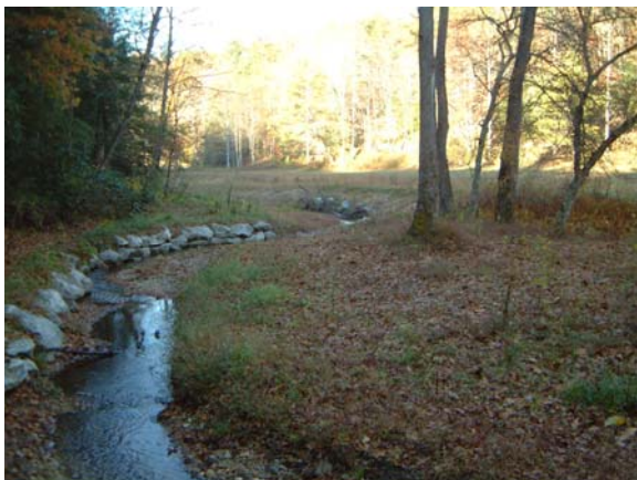
Photo Station #5. Looking downstream at channel plug protection from as-built Station ~41+25.
