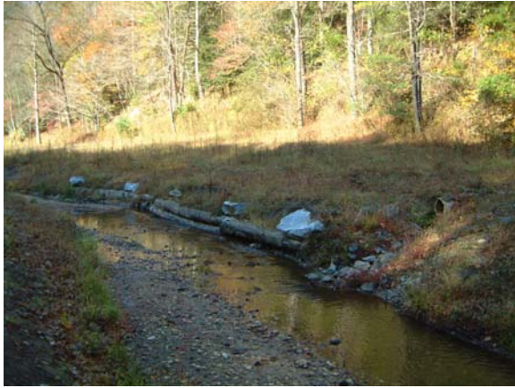
Photograph NM-25. Looking downstream at log toe protection from as-built Station ~31+00.
