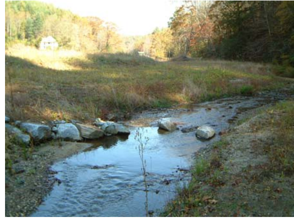
Photograph NM-74. Looking upstream at rock “J” vane from as-built Station ~0+85.
