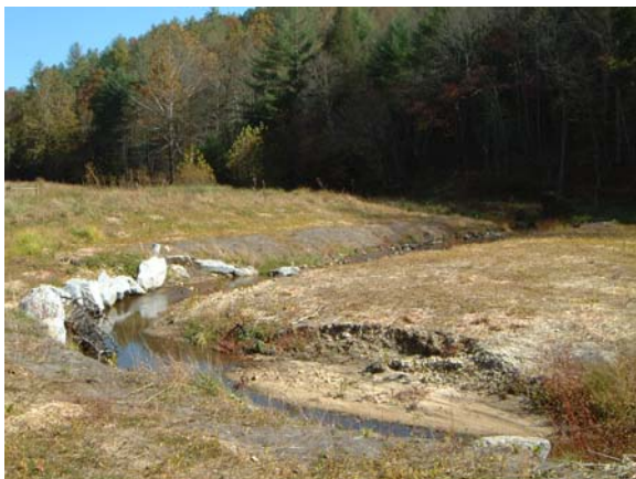
Photograph NM-65. Looking upstream at log toe protection, rootwad, and rock vane from as-built Station ~4+50.
