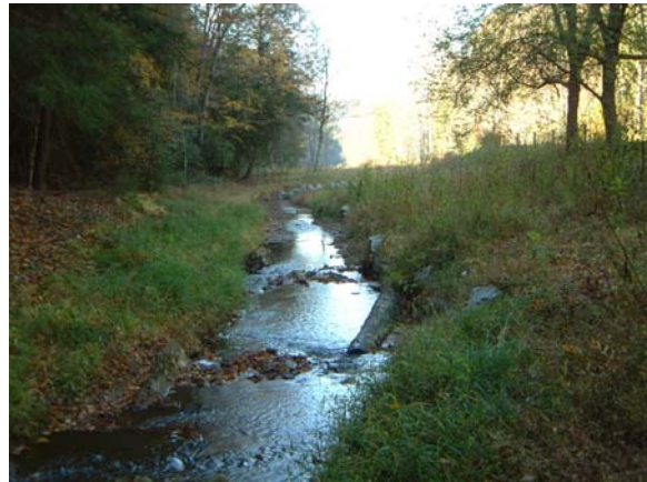
Photograph NM-22. Looking downstream at log vane and log toe protection from as-built Station ~34+00.
