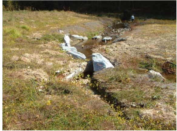
Looking upstream at gully erosion at as-built Station ~5+25.
