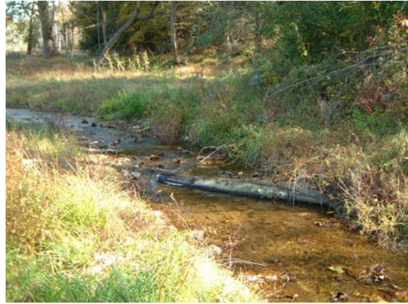
Photograph NM-44. Looking upstream at log vane from as-built Station ~12+75.
