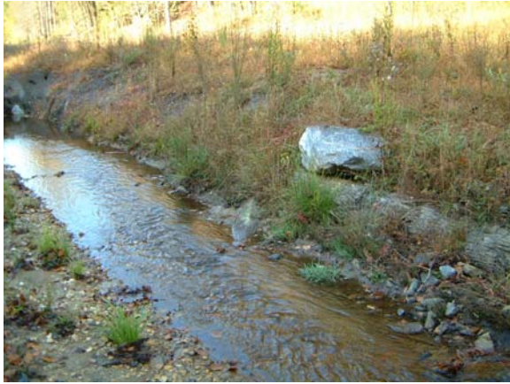
Looking downstream at log vane from as-built Station ~30+25.
