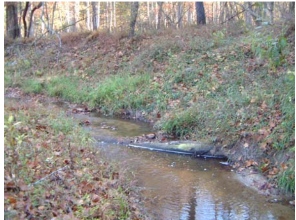
Looking upstream at log vane at as-built Station ~41+50.
