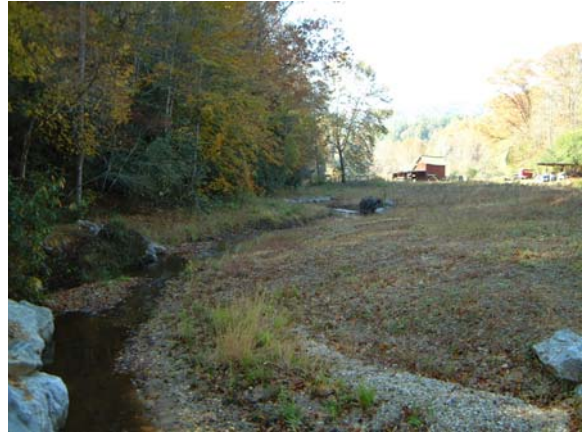
Photo Station #14. Looking downstream from as-built Station ~20+70. Small tributary confluence to left.
