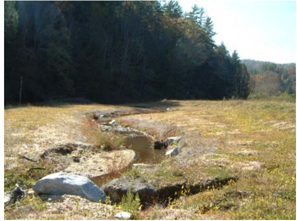
Photo Station #20. Looking downstream from as-built Station ~5+05.
