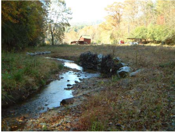
Photograph NM-37. Looking downstream at log toe protection and log vane from Station ~19+70.
