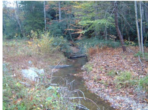
Photograph NM-4. Looking upstream at buried log vane from as-built Station ~49+25.
