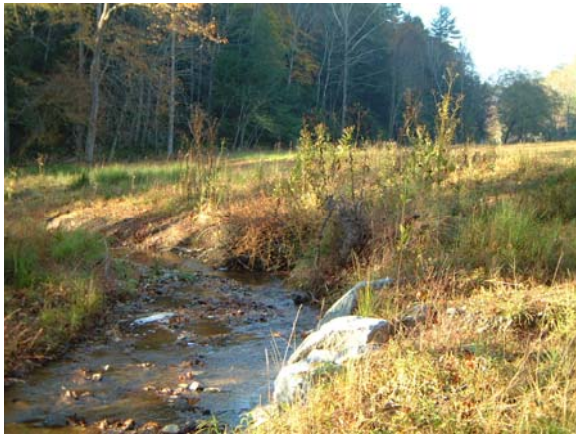
Photograph NM-9. Looking downstream at rootwads and rock toe protection from as-built Station ~43+80.
