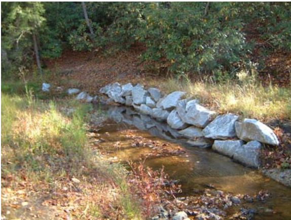
Photograph NM-33. Looking upstream at channel plug protection from as-built Station ~23+00.
