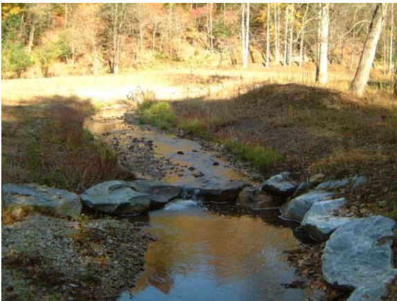
Photograph NM-35. Looking upstream at cross vane from as-built Station ~20+50.
