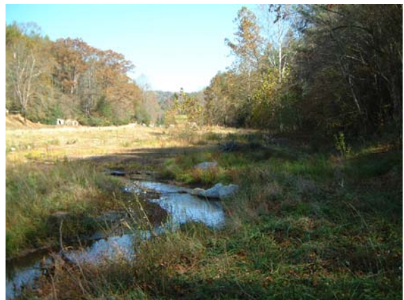
Photograph NM-60. Looking upstream at rock "J" vane and wetland from as-built Station ~ 6+50.
