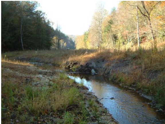
Photograph NM-27. Looking downstream at rootwad and log toe protection from as-built Station ~30+50.
