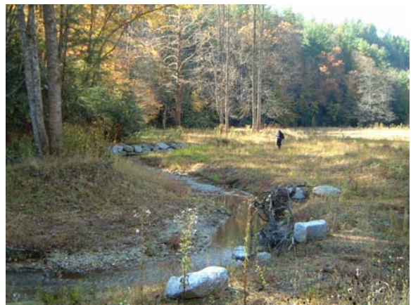
Photo Station #12. Looking downstream from as-built Station ~24+50.
