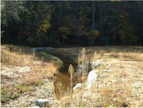
Photo Station #13. Looking downstream from as-built Station ~22+20.
