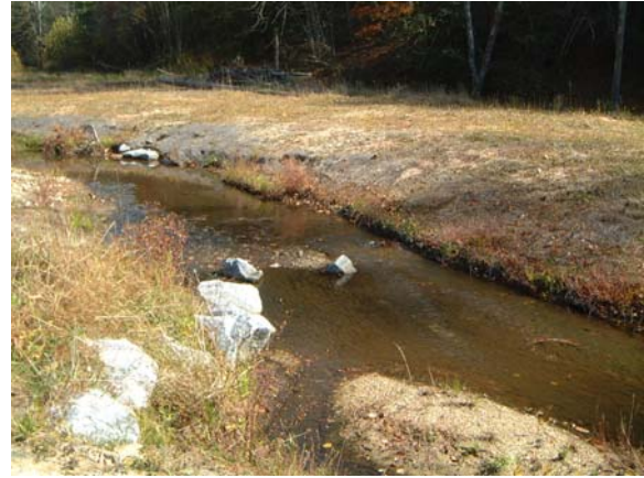
Photograph NM-68. Looking upstream at rock "J" vane from as-built Station ~3+25.
