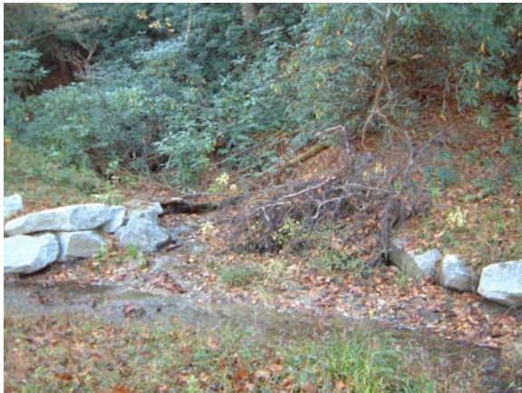
Photograph NM-15. Looking up tributary at confluence with Brown Branch, as-built Station ~41+00.
