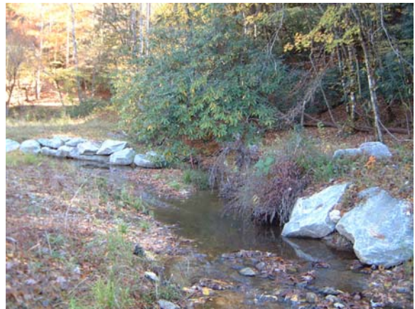
Photograph NM-36. Looking upstream at rootwads and rock toe protection from as-built Station ~20+00.
