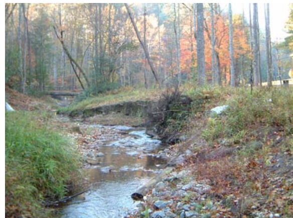
Photograph NM-6. Looking downstream at log vane from as-built Station ~47+25. Severe erosion along right bank.
