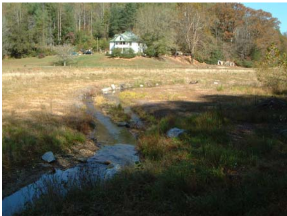
Photograph NM-59. Looking upstream at rock "J" vane from as-built Station ~6+80.
