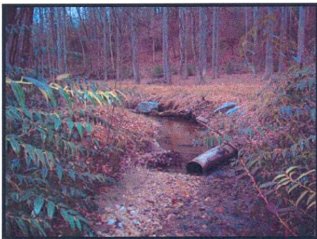
STA 1+25 Down-cut Streambed at a Single Vane Looking Downstream
