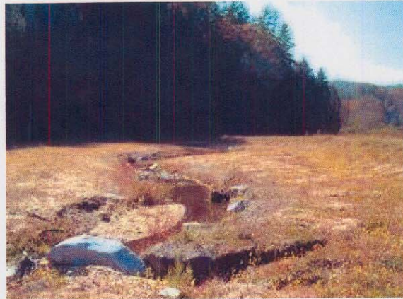
Photo Station #20. Looking downstream from as-built Station ~5+05.
