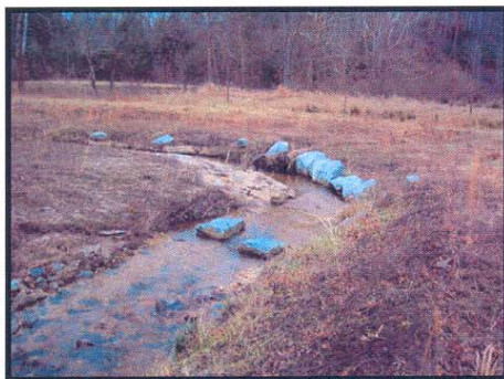
STA 45+40 Looking Downstream @J-Hook and Boulder toe
