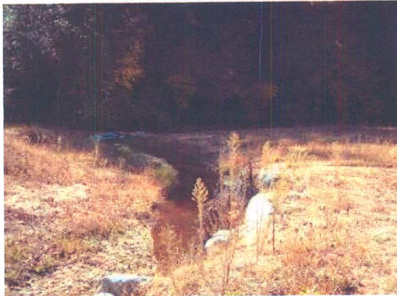
Photo Station #13. Looking downstream from as-built Station ~22+20.
