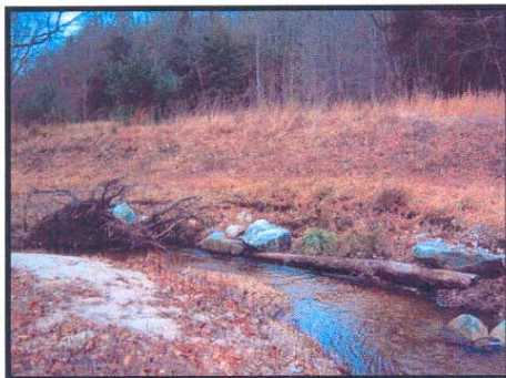
STA 14+75 Looking Downstream @BankErosion
