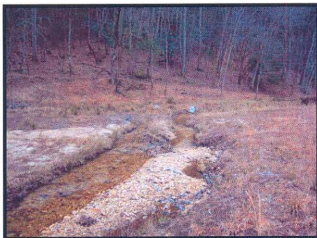
STA 43+10 Looking Downstream @Severe Mid-Channel Bar
