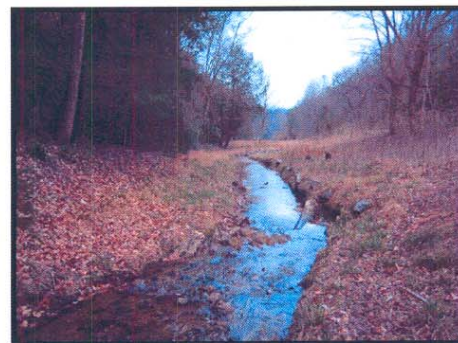
STA 16+50 Looking Downstream @ Single Log Vane and Bank Scour
