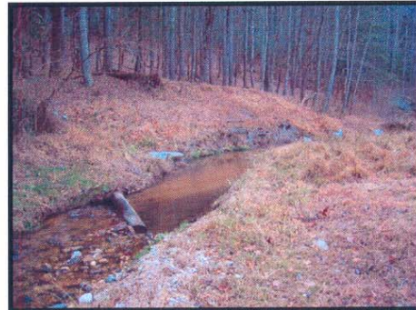
STA 37+40 Downstream @ Down-cut Log Vane
