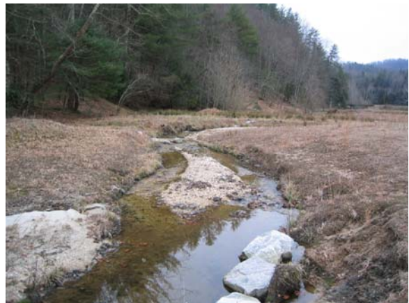
Issue Photo 2. Mid-Channel Bar STA: 40+20
