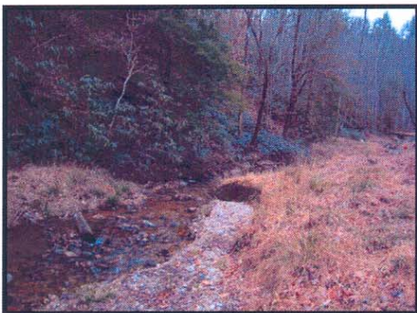
STA 2+90 Bank Blowout and Forming Bench Looking Downstream
