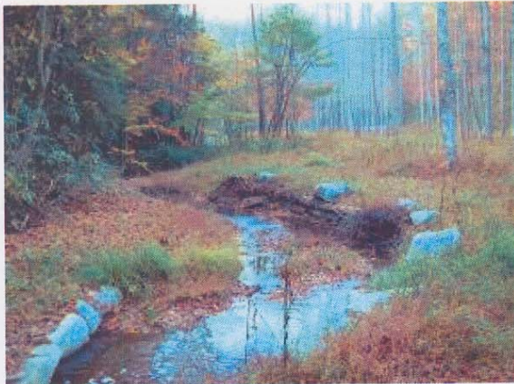
Photo Station #1. Looking downstream from as-built Station ~51+00.
