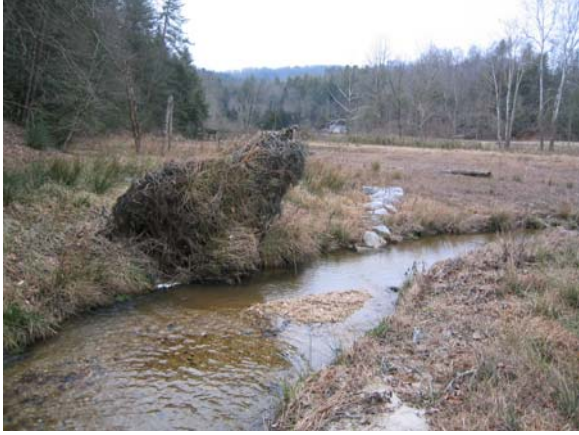
Issue Photo 3 Pool Filling with Sediment At STA: 44+50
