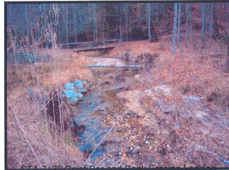
STA 7+70 Point Bar and Bank Erosion Looking Upstream
