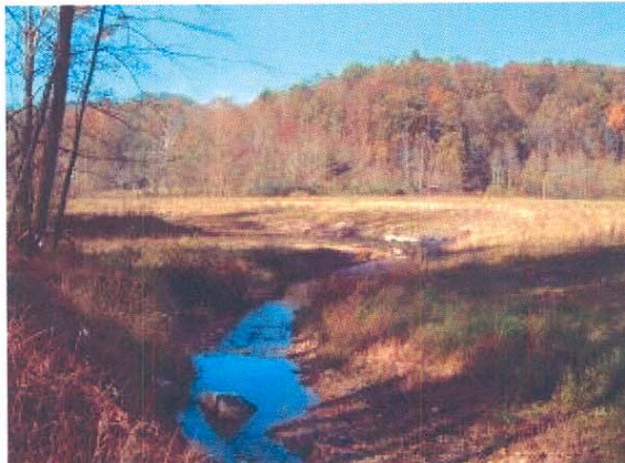
Photo Station #17. Looking downstream from as-built Station ~12+50. Tributary confluence to left. Rock has rolled from bank into channel from left.
