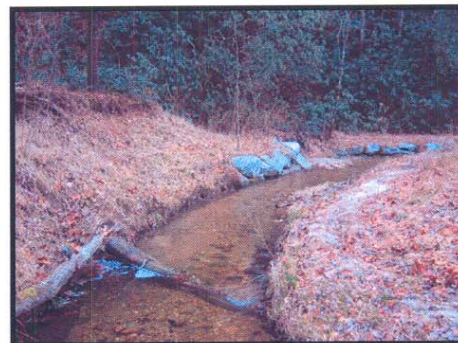
STA 9+70 Down-cut Log Sill Looking Downstream
