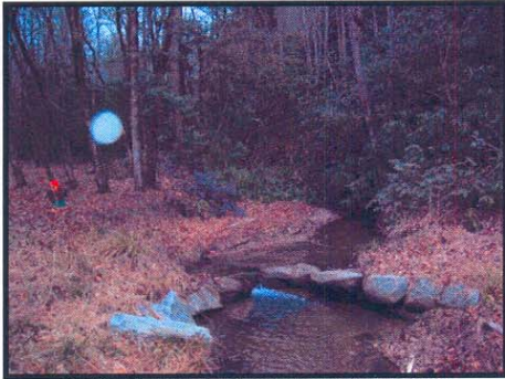
STA 0+25 Looking Upstream at Beginning of Project
