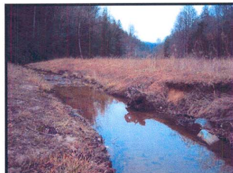
STA 21+30 Looking Downstream @ Bank Erosion Tight Radius of Curvature
