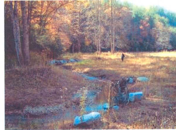
Photo Station #12. Looking downstream from as-built Station ~24+50.
