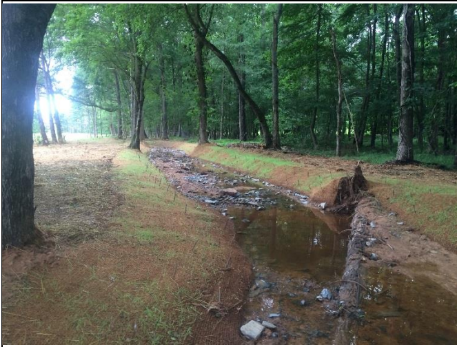
UT4 Reach 2, view downstream at Station 21+50
