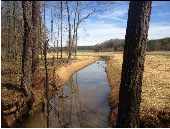
Hurricane Creek Reach 1, view downstream at Station 10+00
