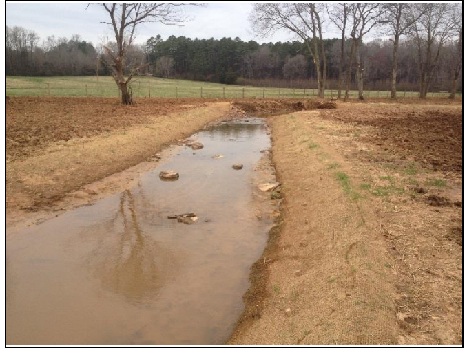
Hurricane Creek Reach 2, view downstream at Station 36+00
