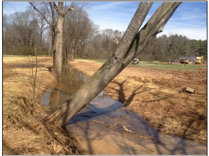
Hurricane Creek Reach 2, view downstream at Station 40+75
