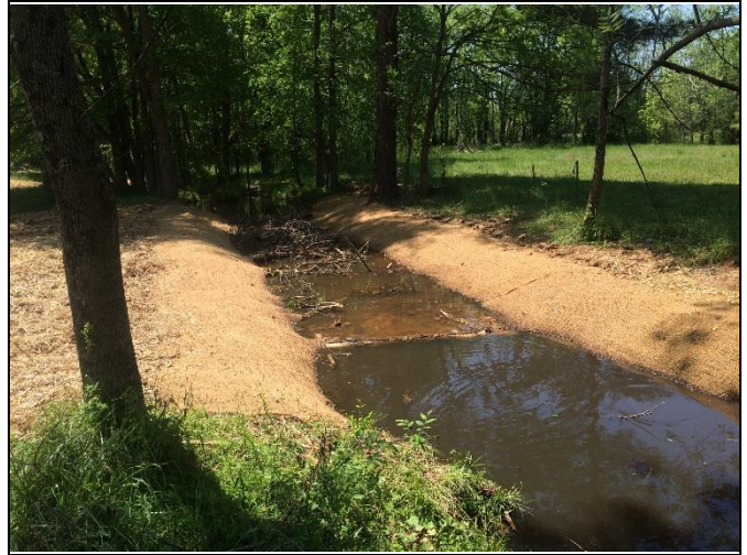
UT4 Reach 4, view upstream at Station 13+40
