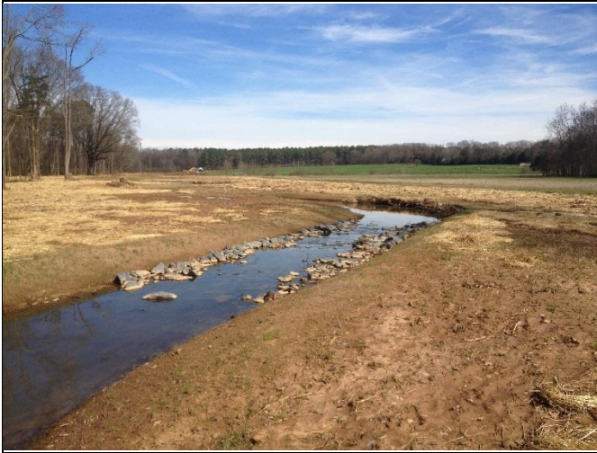
Hurricane Creek Reach 1, view downstream at Station 19+75
