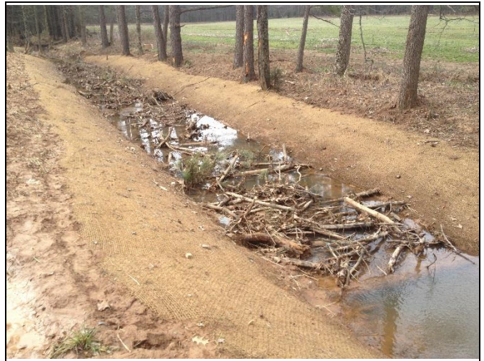
UT4 Reach 5, view upstream at Station 23+75
