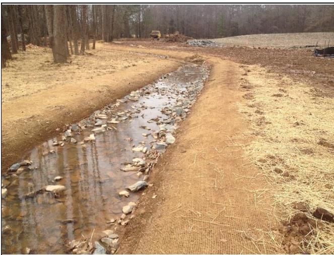
UT4 Reach 1, view downstream at Station 15+40
