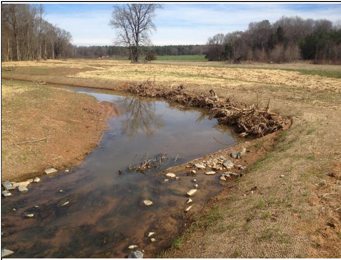
Hurricane Creek Reach 1, view downstream at Station 14+50
