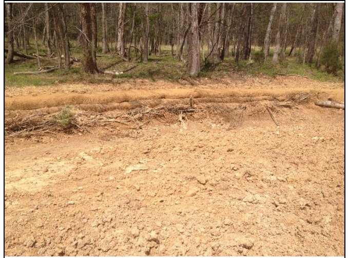
UT4 Reach 2, view at Station 26+00
