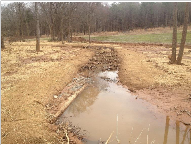
UT4 Reach 1, view upstream at Station 14+15
