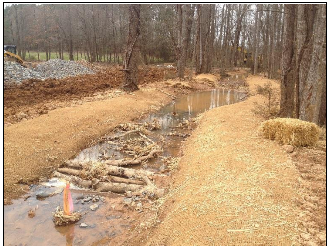
UT4 Reach 1, view downstream at Station 17+20
