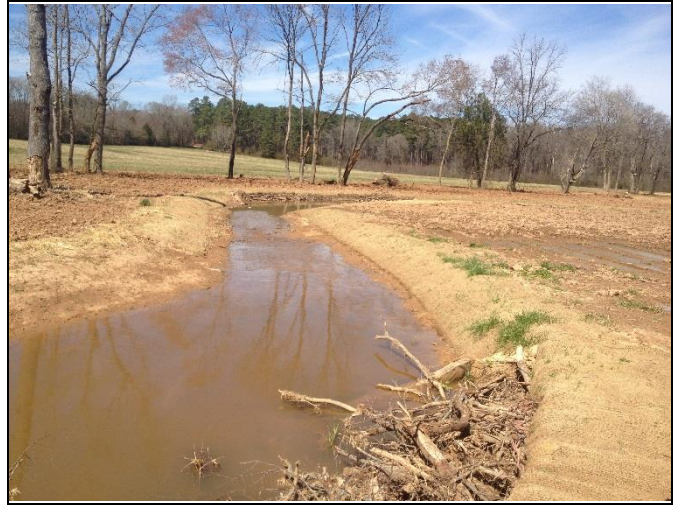
Hurricane Creek Reach 2, view downstream at Station 33+00
