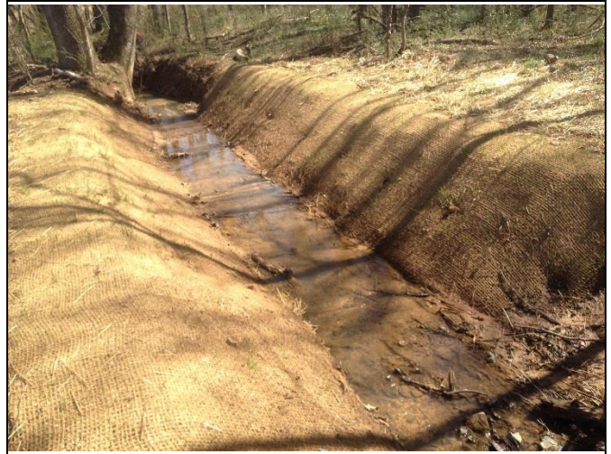
Hurricane Creek Reach 3, view downstream at Station 14+00
