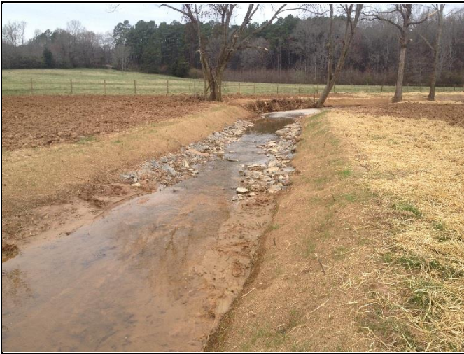
Hurricane Creek Reach 2, view downstream at Station 39+10
