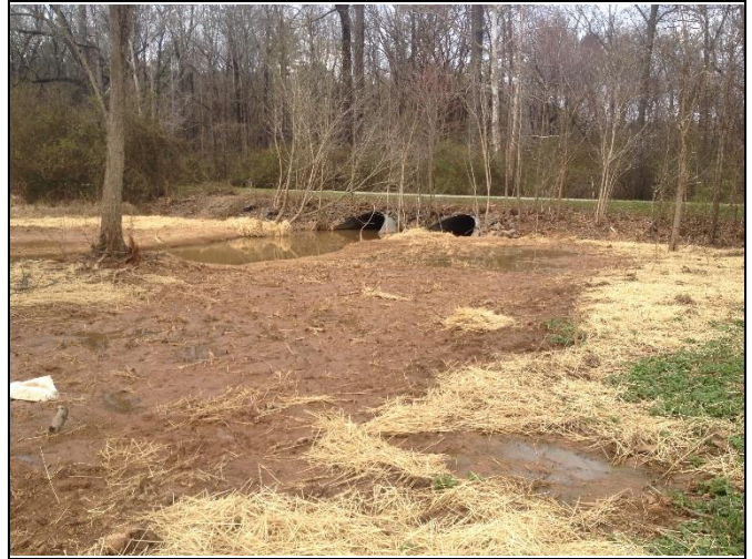
Hurricane Creek Reach 2, view downstream at Station 44+25
