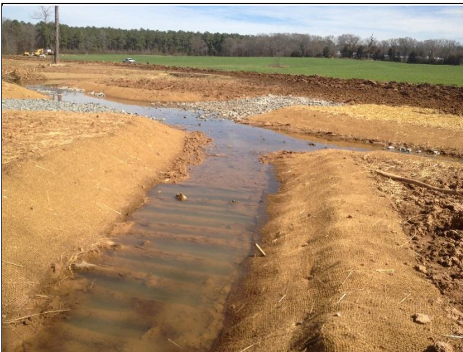
Hurricane Creek Reach 3, view downstream at Station 15+50
