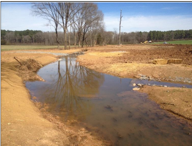
Hurricane Creek Reach 1, view downstream at Station 29+30
