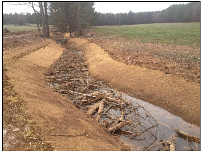
UT4 Reach 5, view upstream at Station 28+25
