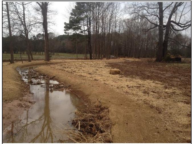
UT4 Reach 1, view downstream at Station 14+25
