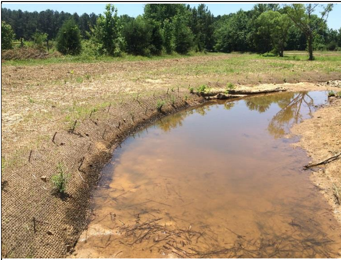
UT4 Reach 4, view upstream at Station 18+20
