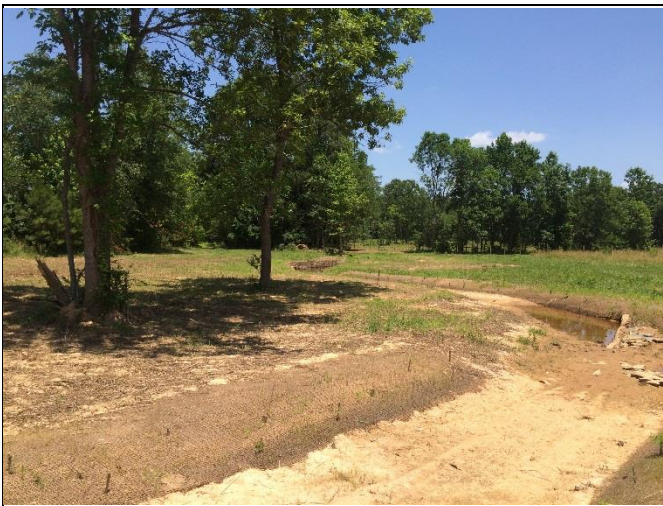
UT4 Reach 4, view downstream at Station 21+25
