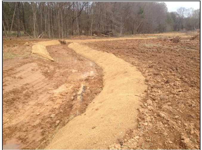
UT4 Reach 2, view upstream at Station 31+75
