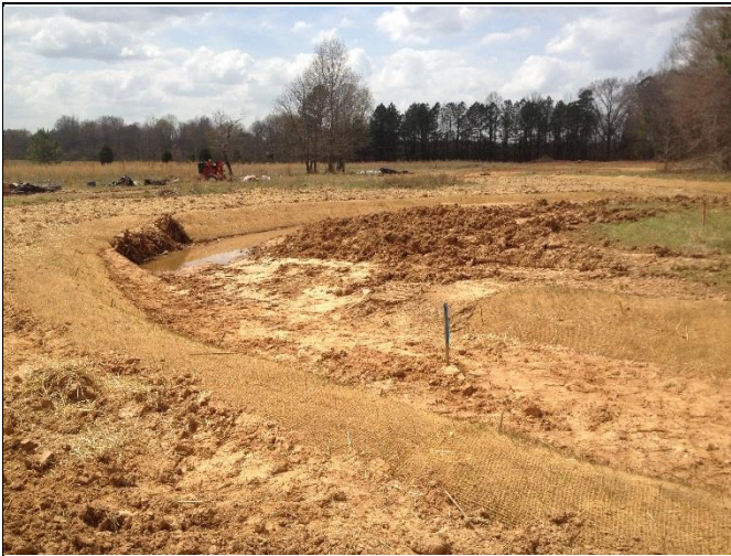
UT4 Reach 2, view downstream at Station 28+75
