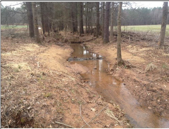
UT4 Reach 5, view upstream at Station 22+20
