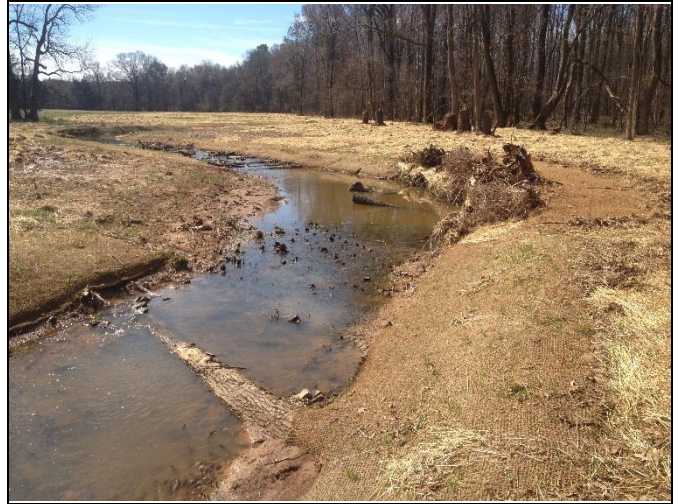
Hurricane Creek Reach 1, view downstream at Station 22+40
