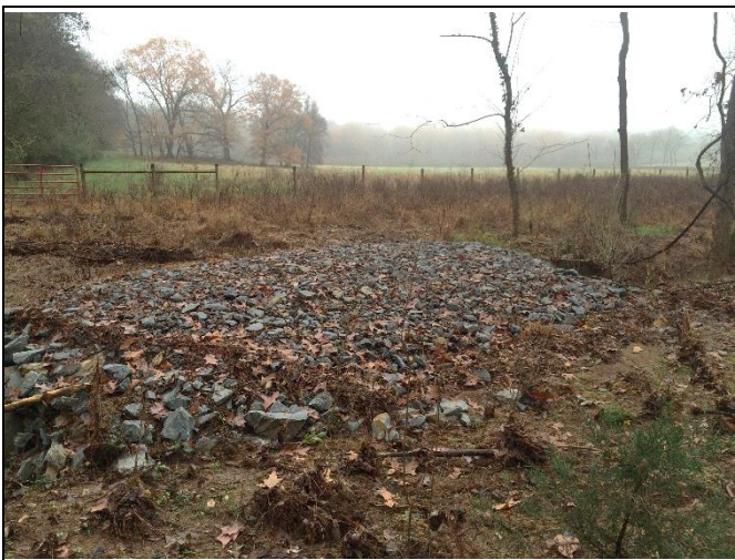
Reach HC-R3 – View of crossing at Station 10+20
