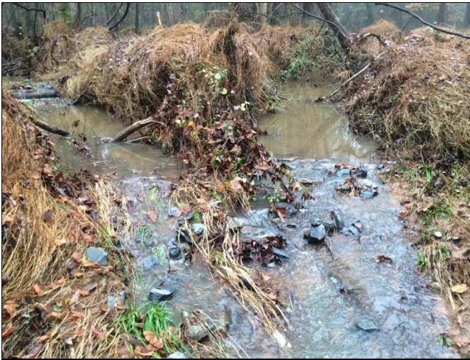
Reach UT4-R5a – View upstream, Station 11+75
