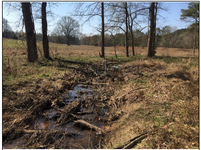
Reach UT4-R1b – View downstream, Station 14+50
