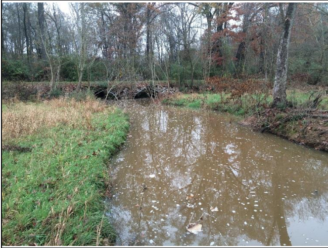
Reach HC-R2 – View downstream to culvert, Station 43+75
