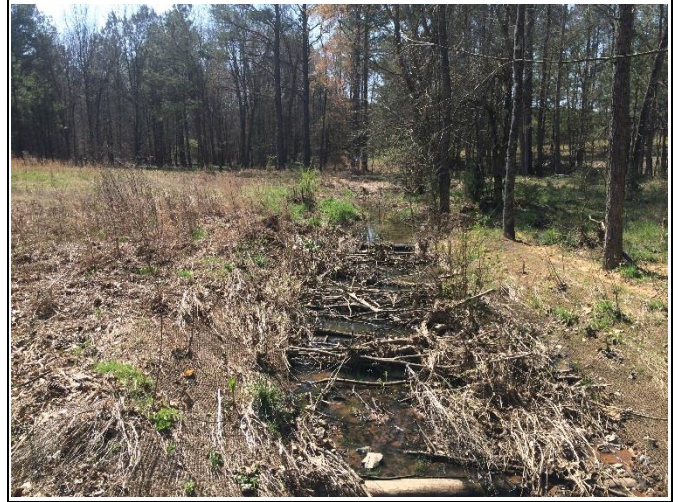
Reach UT4-R4a – View upstream, Station 12+10
