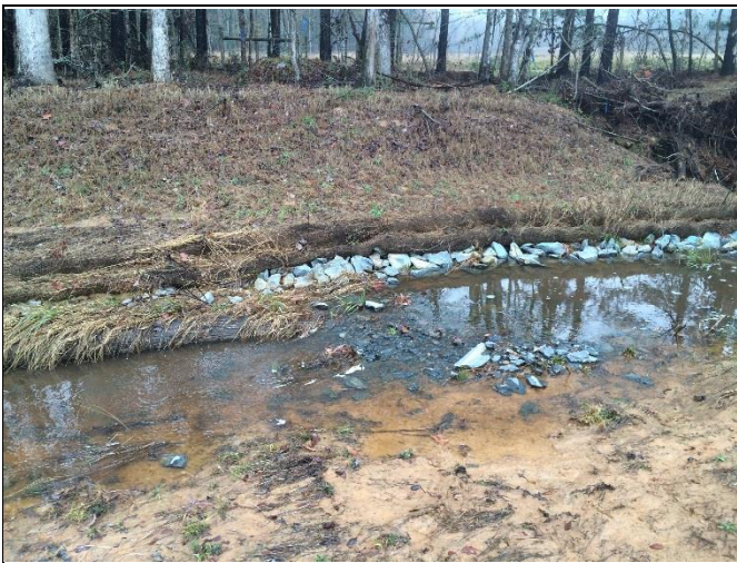
Reach UT4-R4b – View at Station 27+00
