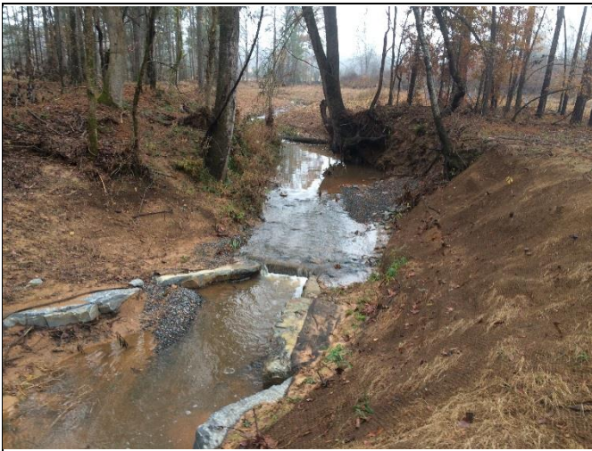
Reach UT4-R3 – View upstream, Station 29+90
