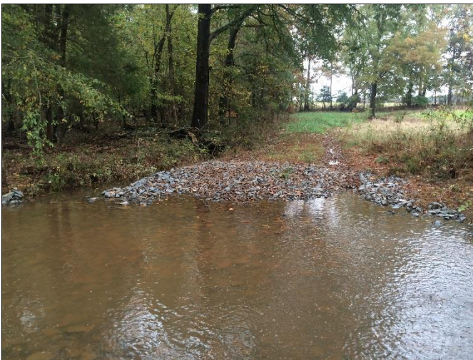
Reach UT4-R2 – View of crossing at Station 21+25
