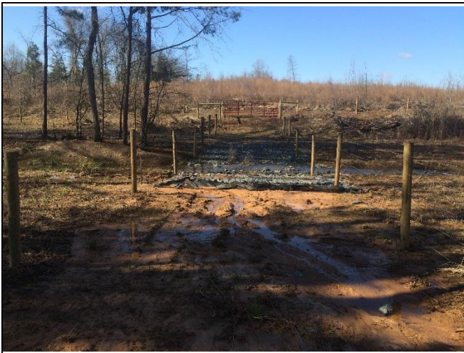
3) Reach UT4-R4b – Crossing erosion at Station 25+30
