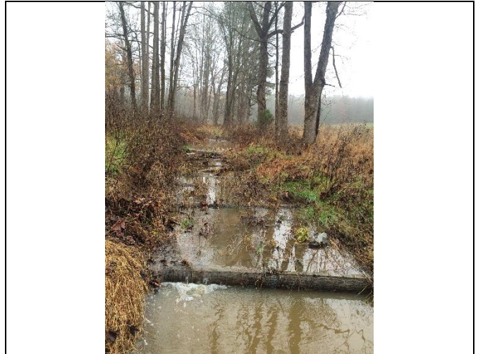
Reach UT4-R1b – View upstream, Station 19+00
