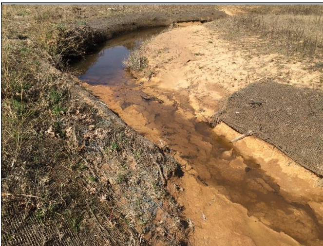
5) Reach UT4-R2 – Riffle scour at Station 28+75
