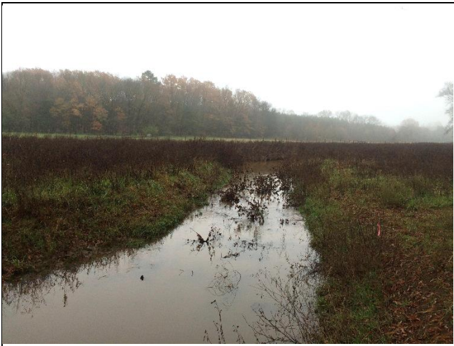
Reach HC-R1 – View upstream, Station 27+00
