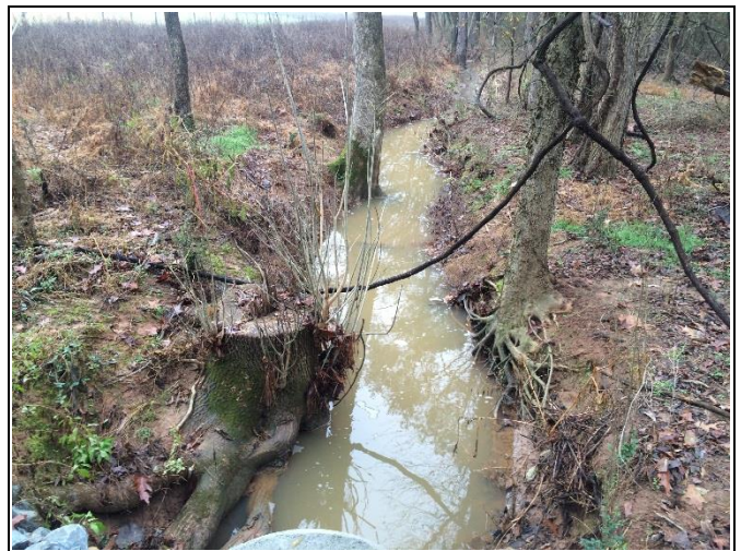
Reach HC-R3 – View downstream from culvert, Station 10+30
