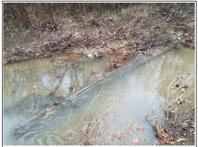
Reach HC-R1 – Log vane at Station 13+50
