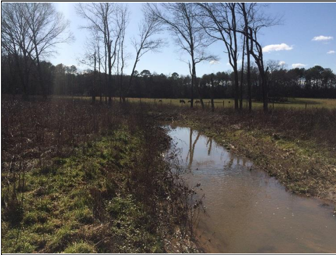
Reach HC-R2 – View upstream, Station 35+25
