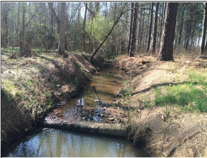
Reach UT4-R5a – View upstream, Station 10+60
