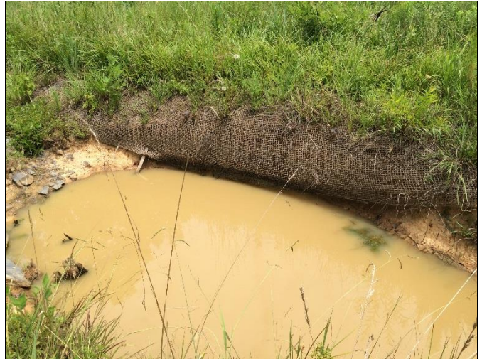
2) Reach UT4-R4b – Bank erosion at Station 23+20
