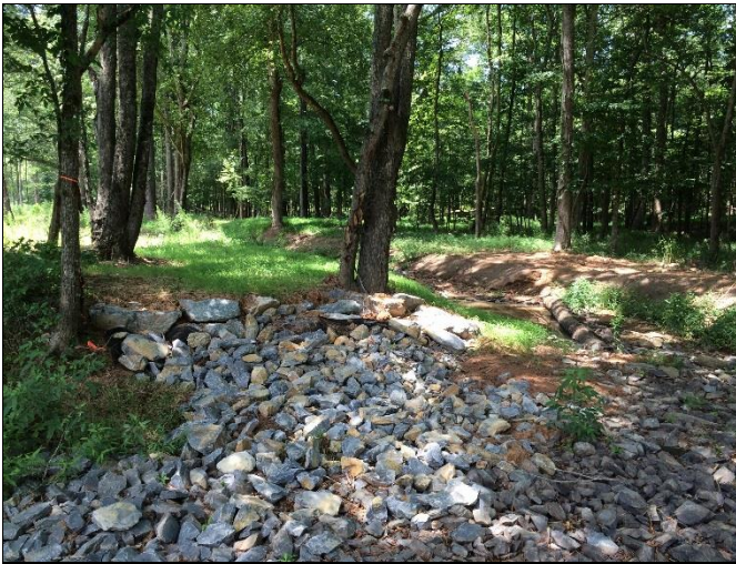
9) Reach UT4-R2: Rock crossing repaired and stabilized at Station 21+40
