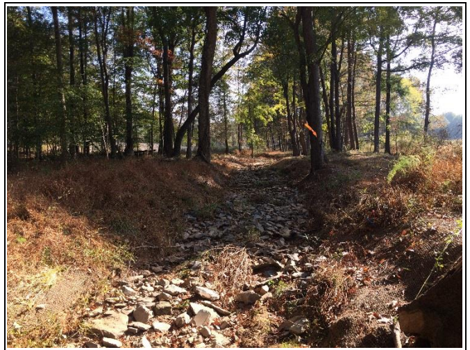
Reach UT4-R2 – View upstream, Station 23+00
