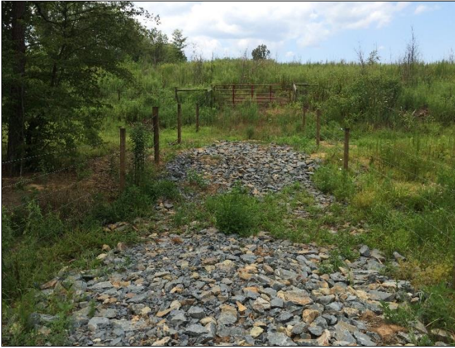
1) Reach UT4-R4b: Rock crossing repaired at Station 25+30
