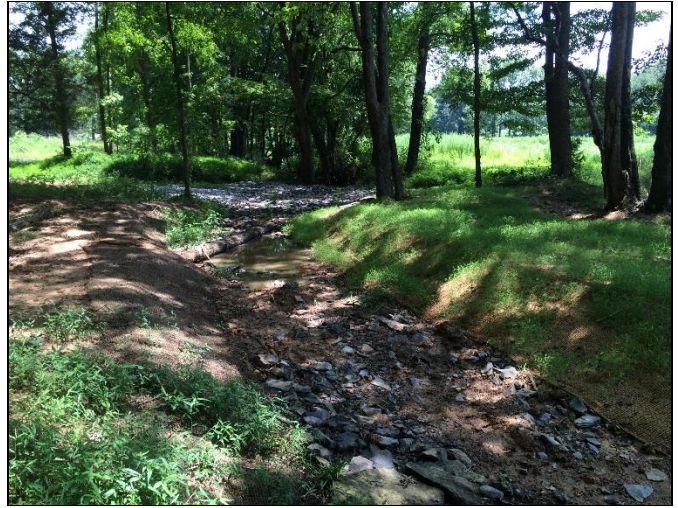
8) Reach UT4-R2: Banks regraded and seeded/matted at Station 22+00
