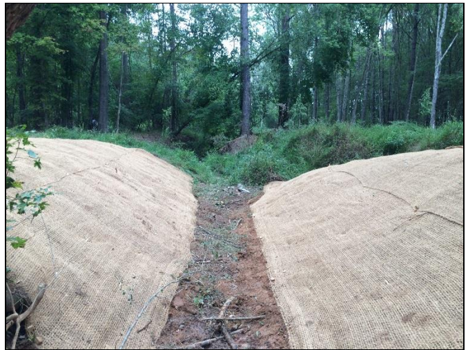
12) Reach UT4-R5a: Banks regraded and seeded/matted at Station 11+00
