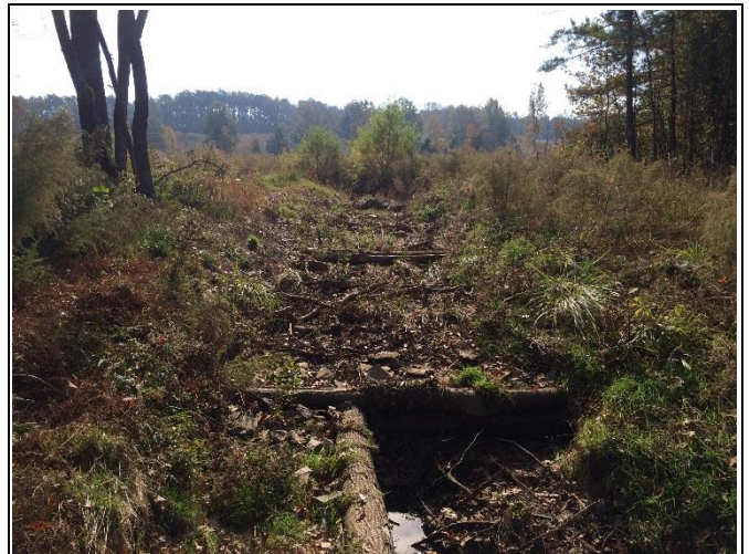
Reach UT4-R2 – View upstream, Station 37+00
