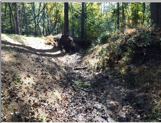
Reach UT4-R5a – View upstream, Station 12+75
