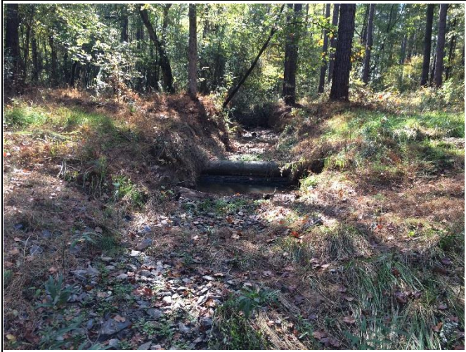
Reach UT4-R5a – View upstream, Station 10+75
