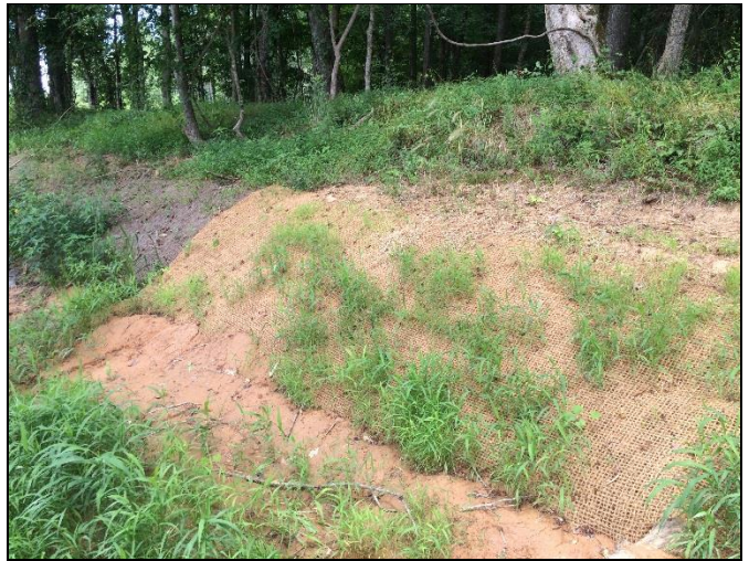
4) Reach UT4-R2: Slopes regraded and seeded/matted at Station 37+40
