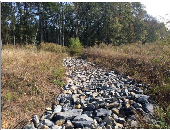
Reach UT4-R2 – View upstream, Station 31+50
