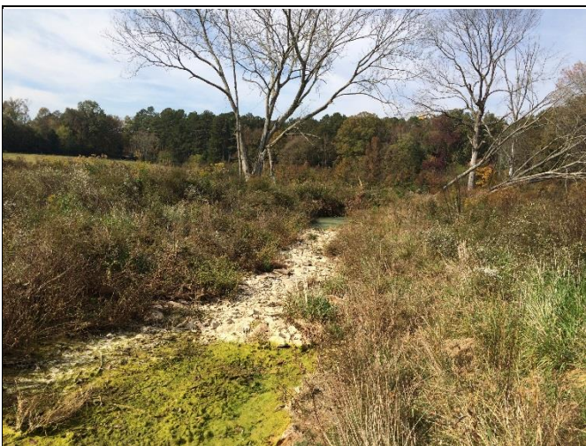
HC Reach 2, view downstream at Station 39+10
