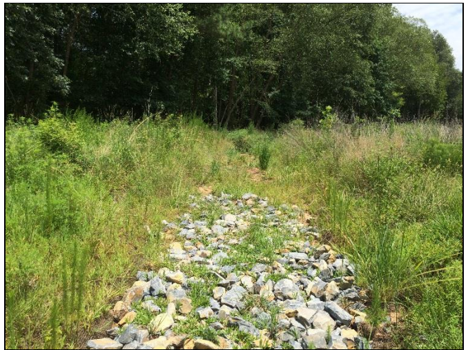
6) Reach UT4-R2: Riffle regraded and stabilized with rock at Station 28+75
