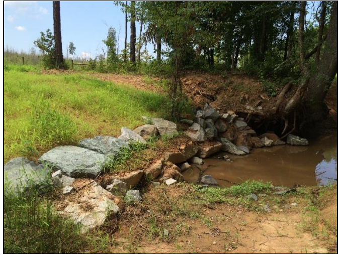
2) Reach UT4-R3: Boulder revetment replaced J-hook at Station 29+00
