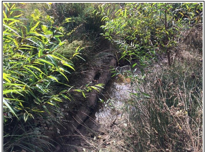
Reach UT4-R1b – View downstream, Station 13+25
