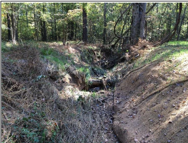
Reach UT4-R5a – View of side tributary at Station 11+75
