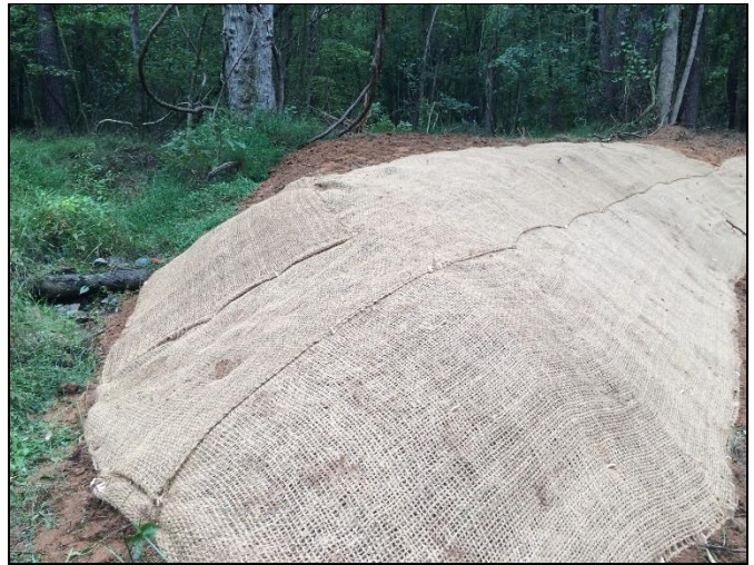
10) Reach UT4-R5a: Banks regraded and seeded/matted at Station 11+75
