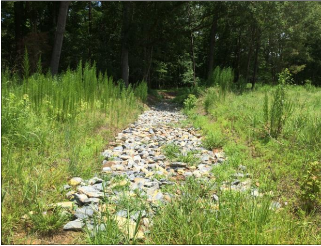
7) Reach UT4-R2: Riffle regraded and stabilized with rock at Station 24+00
