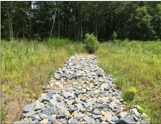
5) Reach UT4-R2: Riffle regraded and stabilized with rock at Station 31+00
