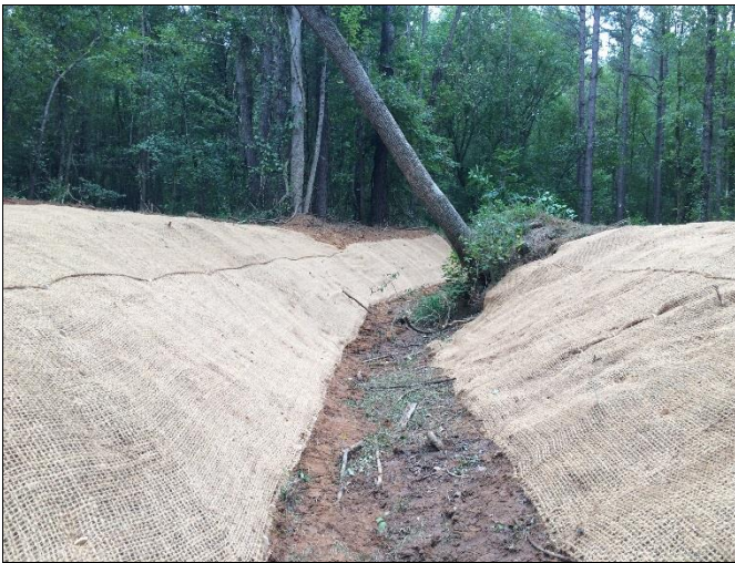
11) Reach UT4-R5a: Banks regraded and seeded/matted at Station 11+50
