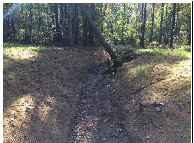
Reach UT4-R5a – View upstream, Station 11+50
