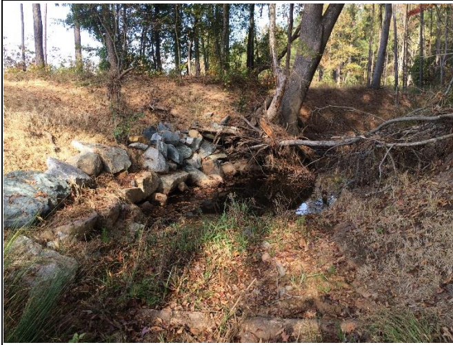
Reach UT4-R3 – View downstream, Station 29+00
