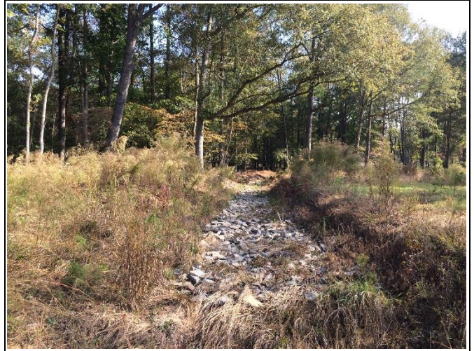
Reach UT4-R2 – View upstream, Station 24+50
