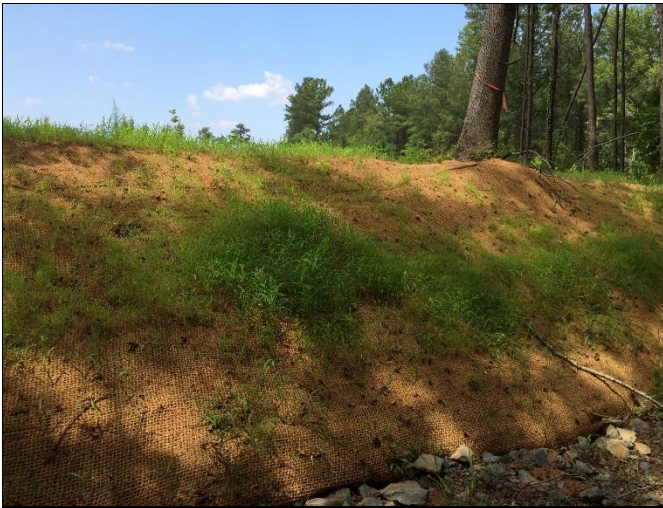
3) Reach UT4-R3: Slopes regraded and seeded/matted at Station 31+00
