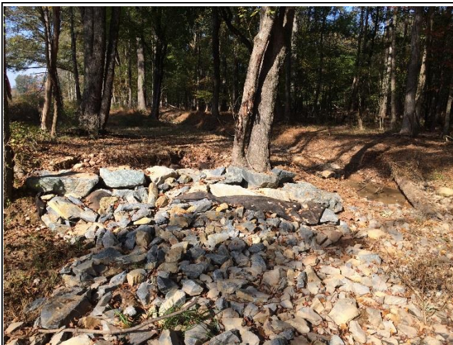
Reach UT4-R2 – View downstream, Station 20+40
