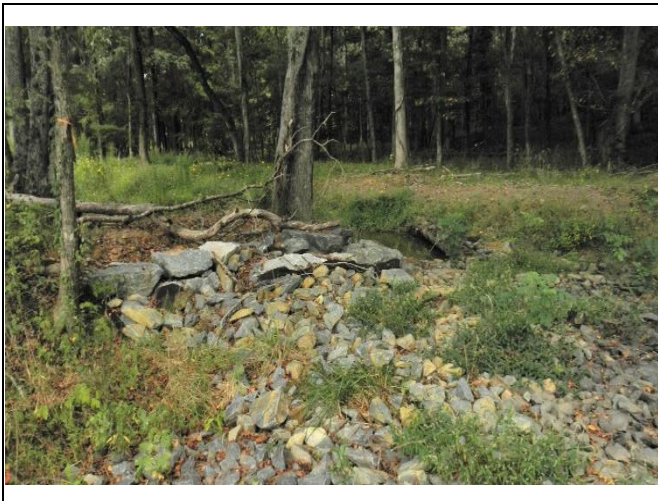
Reach UT4-R2 – View downstream, Station 20+40
