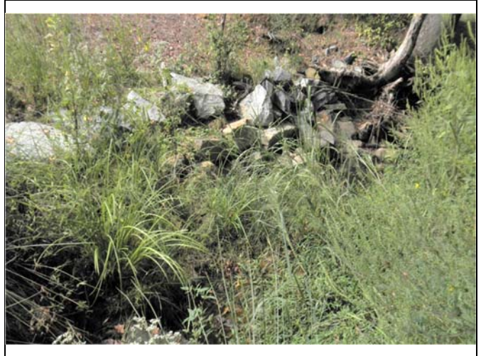
2) Reach UT4-R3: Boulder revetment, Station 29+00
