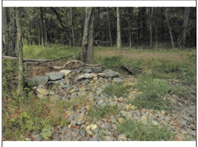
8) Reach UT4-R2: Bank at crossing stabilized with rock, Station 21+40
