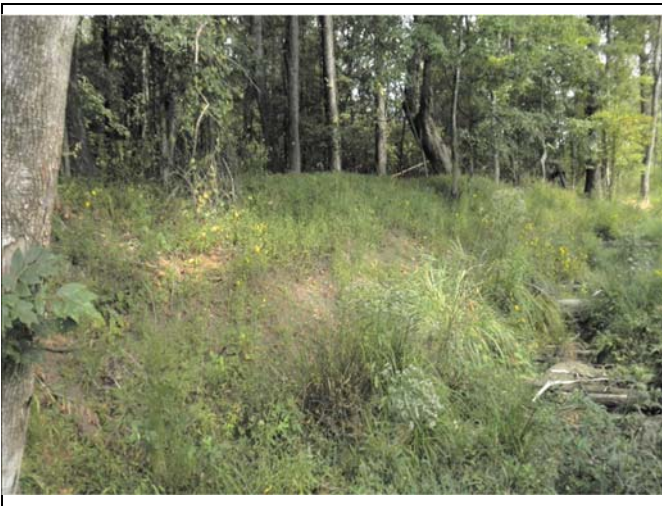
3) Reach UT4-R2: Bank regraded, Station 37+40
