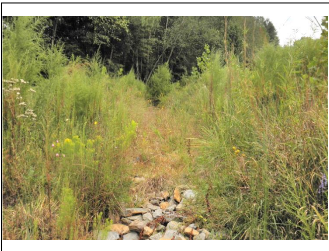
Reach UT4-R2 – View upstream at Station 29+00
