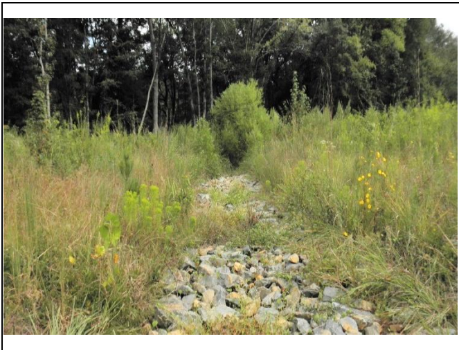
Reach UT4-R2 – View upstream, Station 31+50
