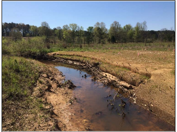
2) Reach UT4-R2: Geolift Installed March 2017 (AFTER)
