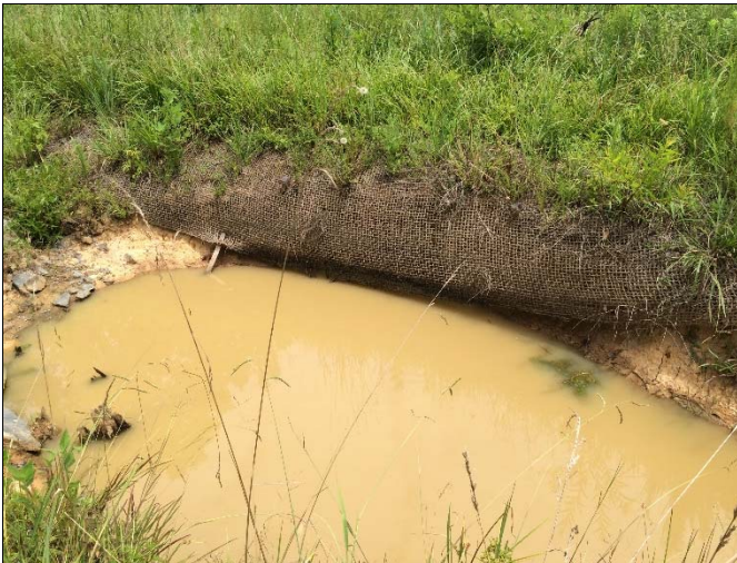
3) Reach UT4-R4b: Bank Erosion, Station 23+30 (BEFORE)
