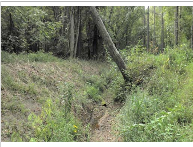
9) Reach UT4-R5a: Banks regraded, Station 11+50
