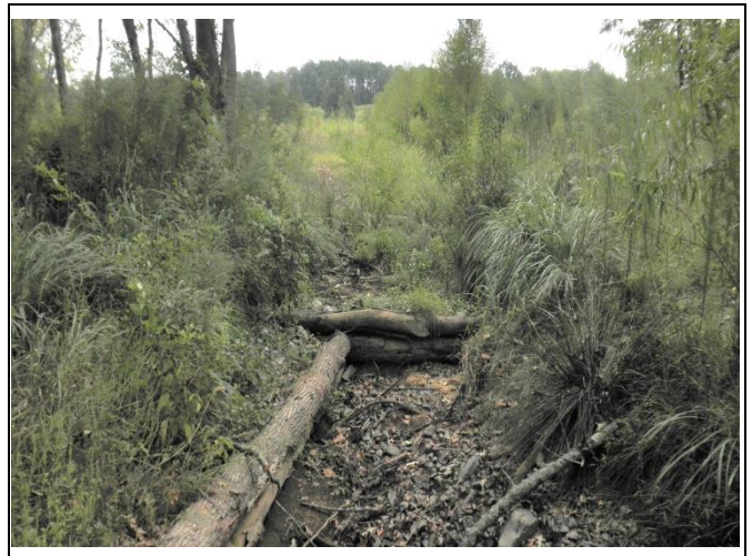
Reach UT4-R2 – View upstream, Station 37+00
