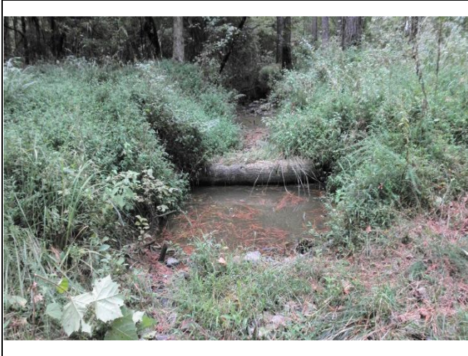
Reach UT4-R5a – View upstream, Station 10+75
