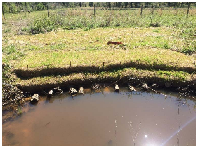
4) Reach UT4-R4b: Geolift Installed March 2017 (AFTER)
