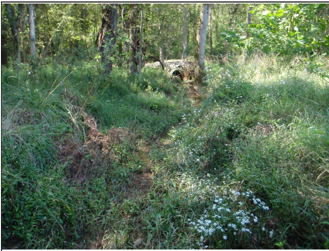
HC Reach 3, view upstream at Station 11+40
