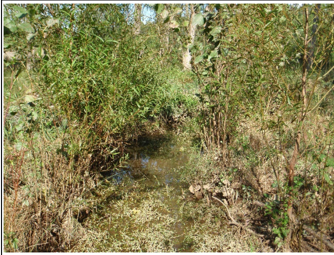
Reach UT4-R1b – View upstream, Station 14+25
