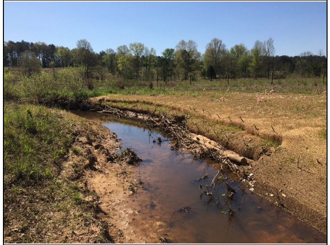
Reach UT4-R2: Stream bank repair, Station 31+75 (post-repair in March 2017)
