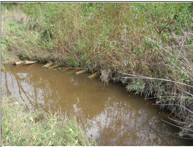
Reach UT4-R4b, Stream bank repair in Oct. 2018
