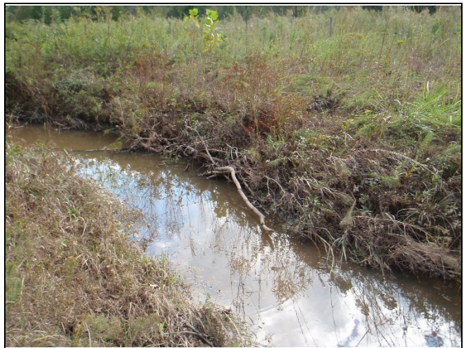
Reach UT4-R2, Stream bank repair in Oct. 2018
