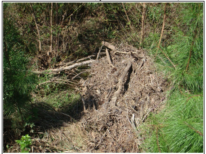
Reach HC-R1: Wrack lines and debris in floodplain
