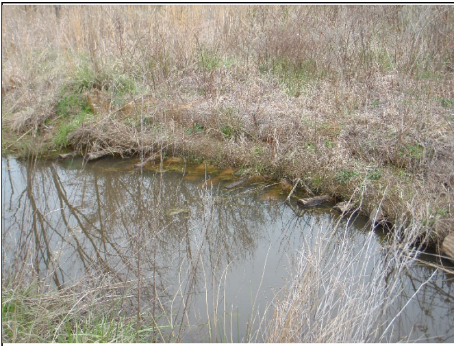
Reach UT4-R4b, Stream bank repair in March 2018
