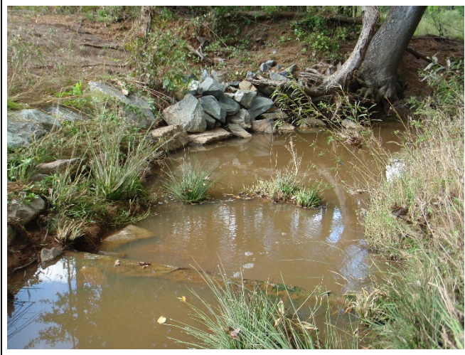
Reach UT4-R3 – View downstream, Station 29+00
