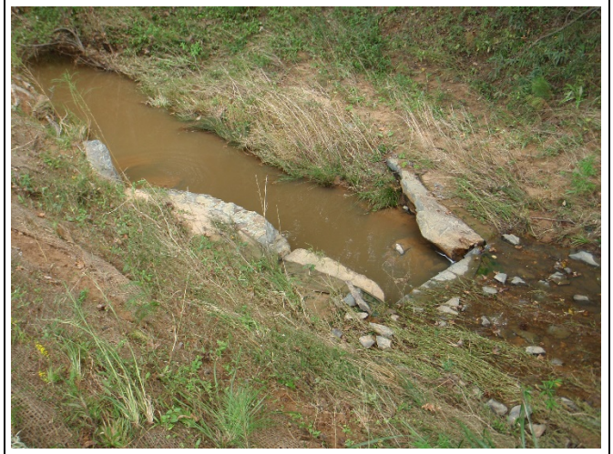
Reach UT4-R3 – View downstream, Station 29+50
