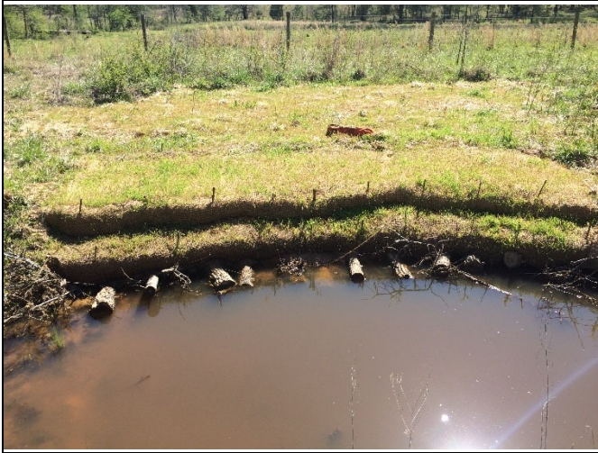
Reach UT4-R4b: Stream bank repair, Station 23+30 (post-repair in March 2017)
