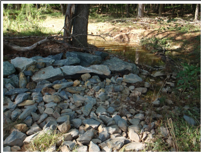
Reach UT4-R2 – View downstream, Station 20+40
