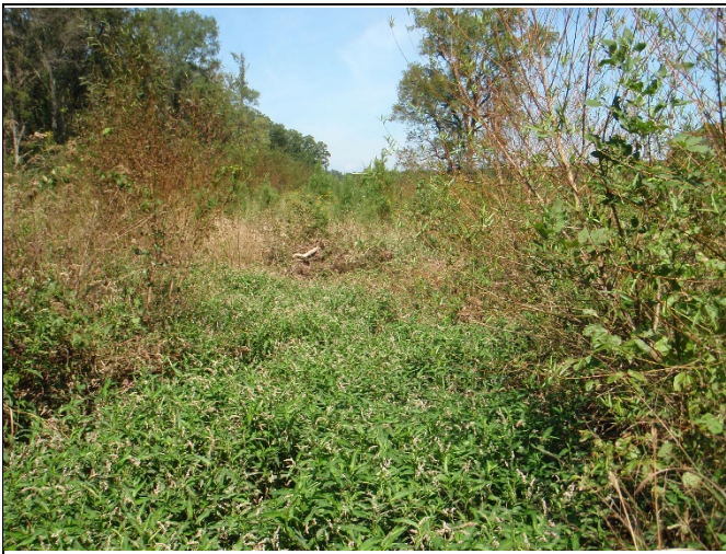
HC Reach 1, view downstream at Station 14+50
