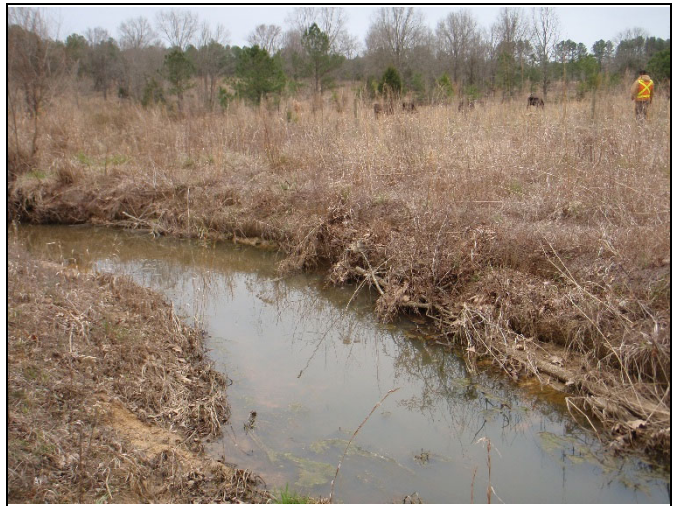
Reach UT4-R2, Stream bank repair in March 2018
