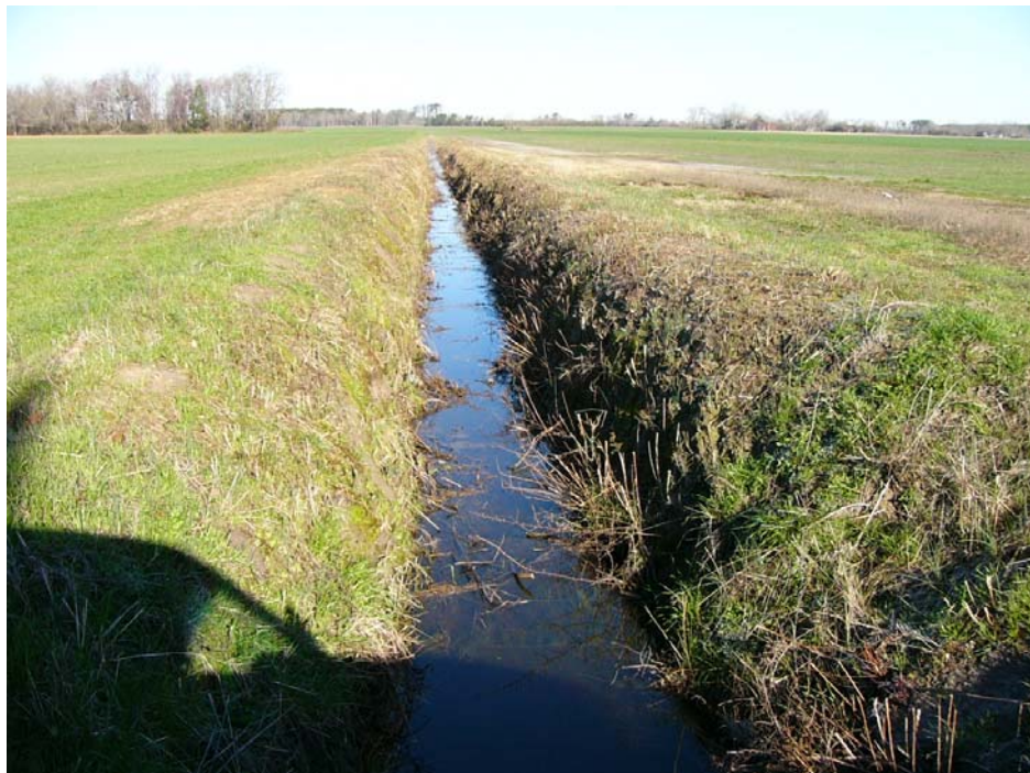
Southern UT looking upstream. Notice stream has been channelized and regularly maintained.
