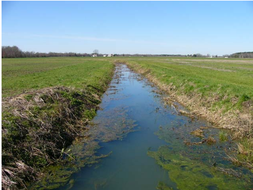
Northern UT looking downstream from crossing
