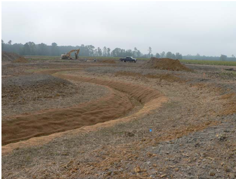
Construction of Northern UT Channel and Floodplain
