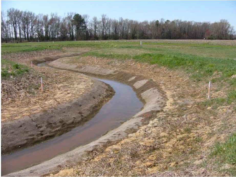
Permanent Photo Station – Cross Section 13
