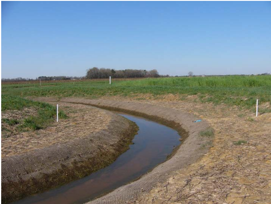
Permanent Photo Station – Cross Section 4
