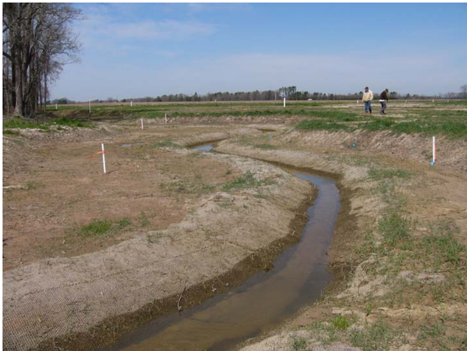
Permanent Photo Station – Cross Section 18
