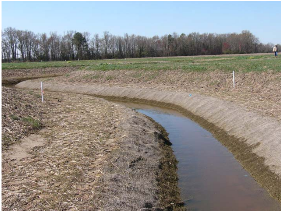
Permanent Photo Station – Cross Section 10
