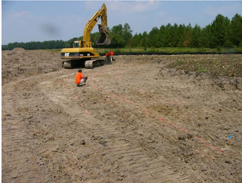
Construction of Northern UT Floodplain
