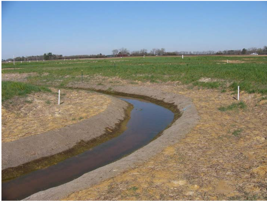
Permanent Photo Station – Cross Section 7
