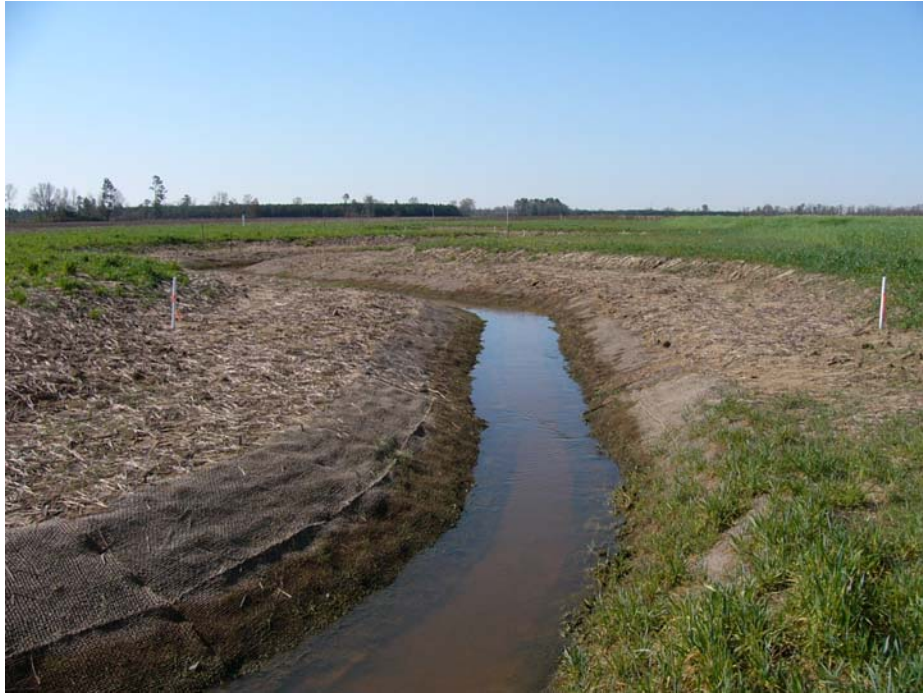
Permanent Photo Station – Cross Section 1
