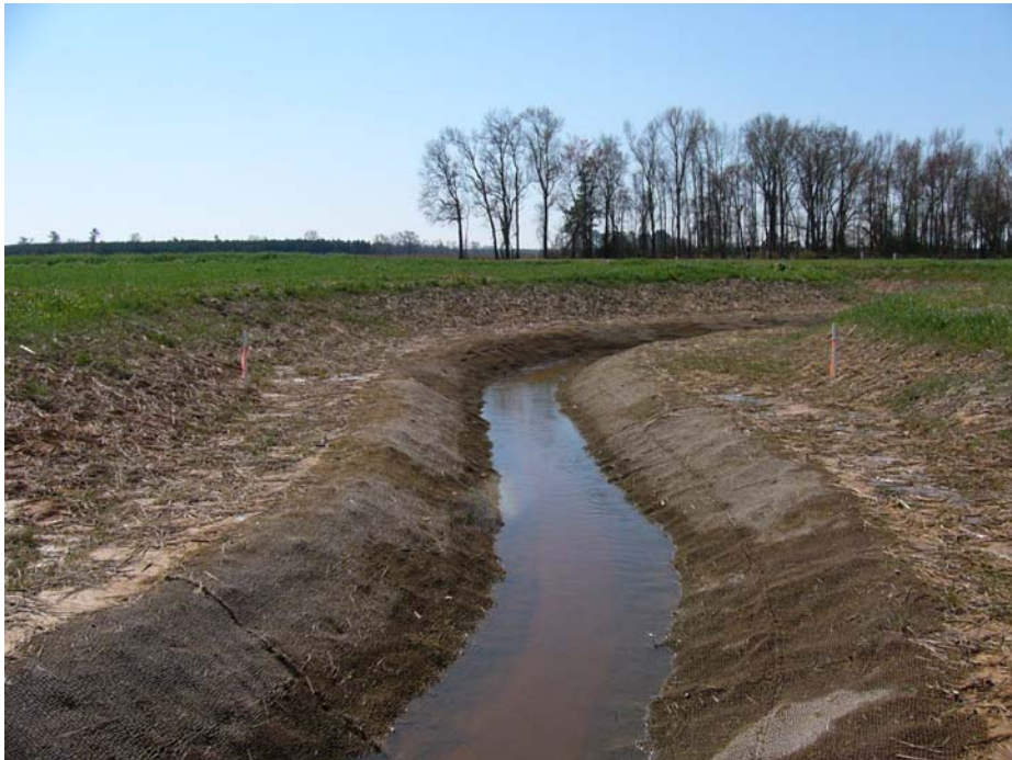
Permanent Photo Station – Cross Section 14
