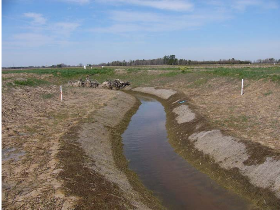
Permanent Photo Station – Cross Section 11
