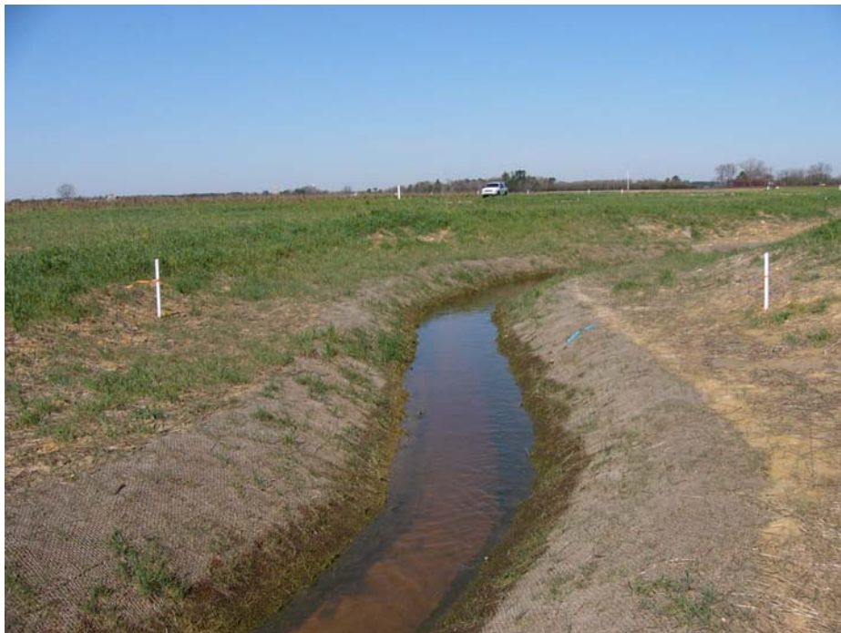
Permanent Photo Station – Cross Section 6
