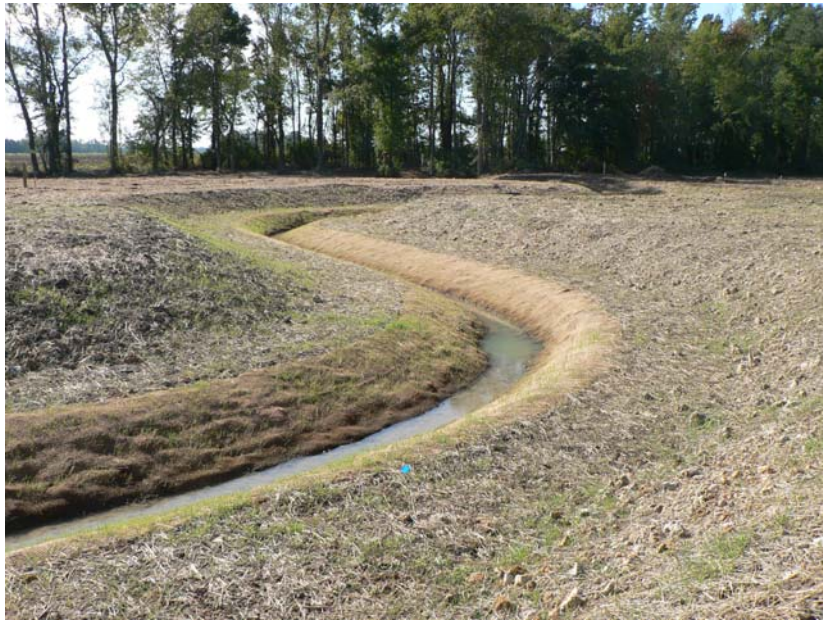
Northern UT looking downstream towards confluence with Lower Reach
