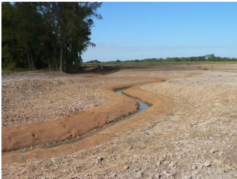
Southern UT looking downstream towards confluence with Upper Reach
