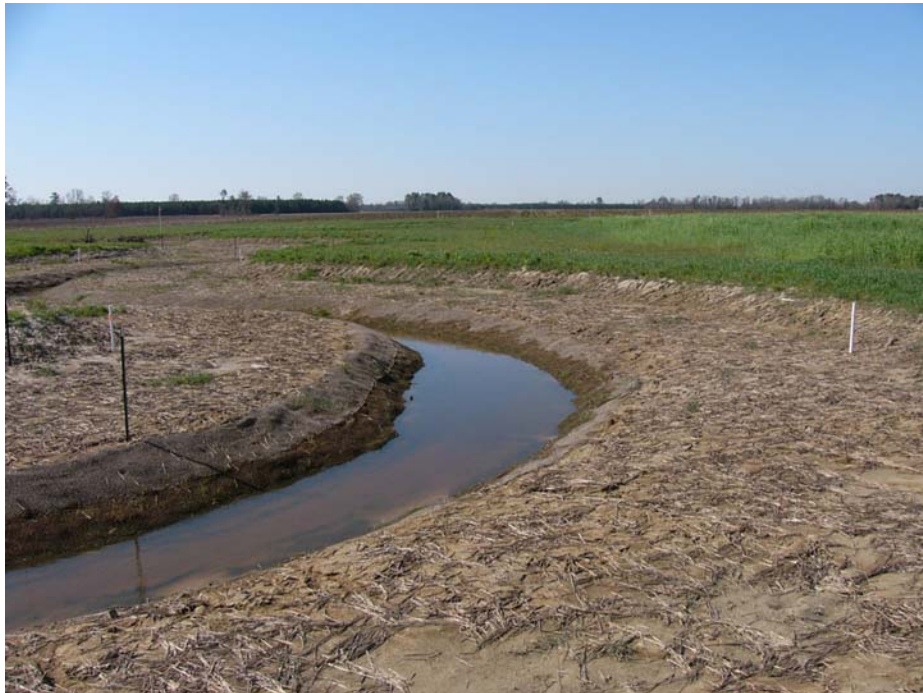
Permanent Photo Station – Cross Section 2
