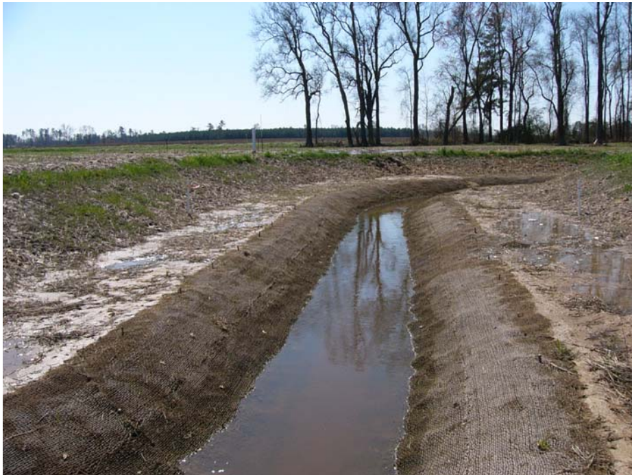
Permanent Photo Station – Cross Section 16
