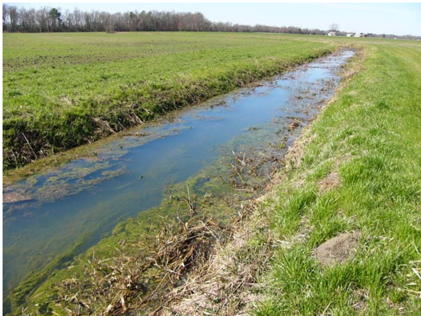
Northern UT looking downstream at maintained banks
