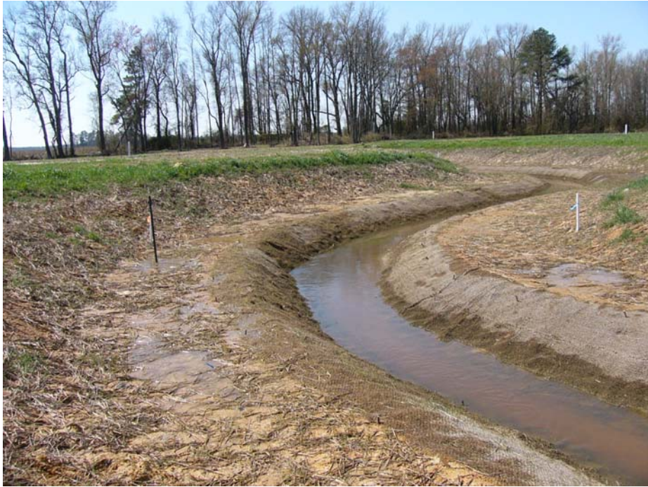
Permanent Photo Station – Cross Section 15
