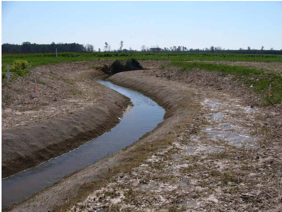
Permanent Photo Station – Cross Section 12
