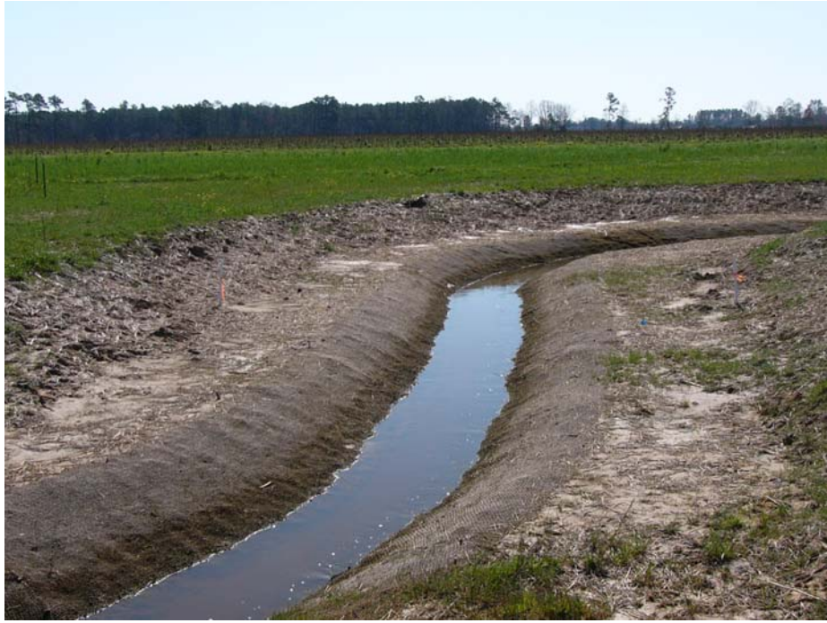
Permanent Photo Station – Cross Section 9
