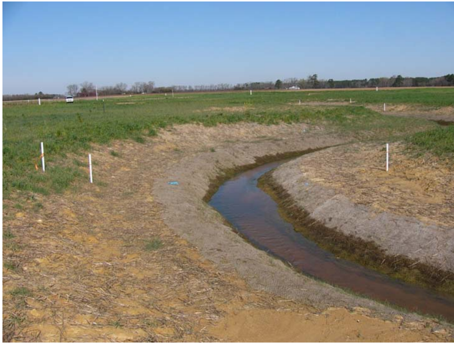
Permanent Photo Station – Cross Section 5
