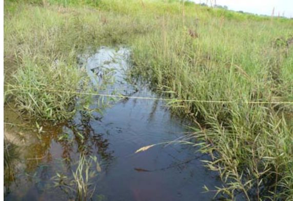
Photo of Cross-Section R3-12 - Looking Downstream @ STA 45+05
