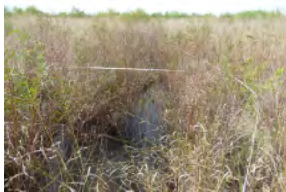
Photo of Cross-Section R5-4 - Looking Downstream @ STA 17+40
