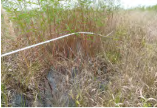
Photo of Cross-Section R4-7 - Looking Downstream @ STA 22+95
