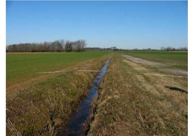
Southern UT looking downstream at recently mowed banks.
