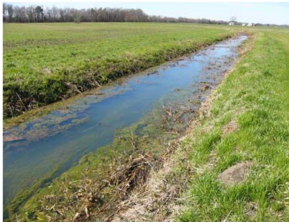
Northern UT looking downstream at maintained banks, algal blooms, and agricultural practices adjacent to stream banks
