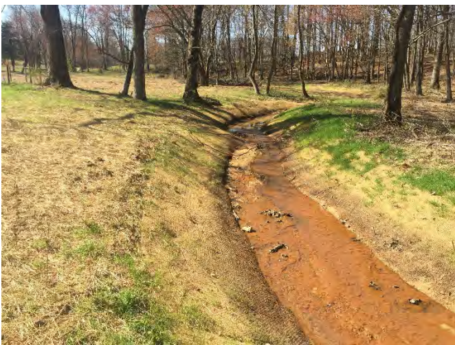
Reach 2 Upper enhancement 1 (Asbuilt)
