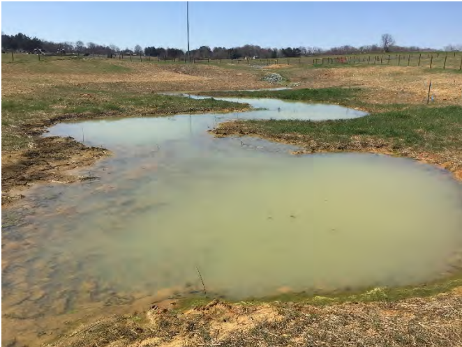
BMP on Reach 6 (Asbuilt)
