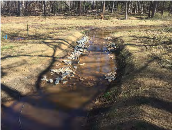
Reach 1 riffle with adjacent wetlands (Asbuilt)
