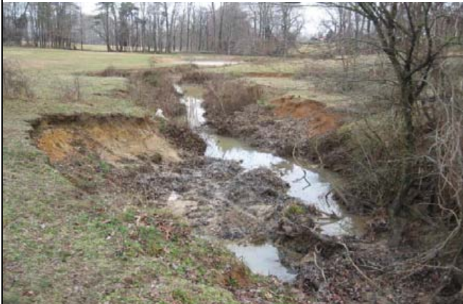
Downstream view along lower Reach R4. Reach T3 enters in background on right, marking the beginning of R3. (2/27/12)
