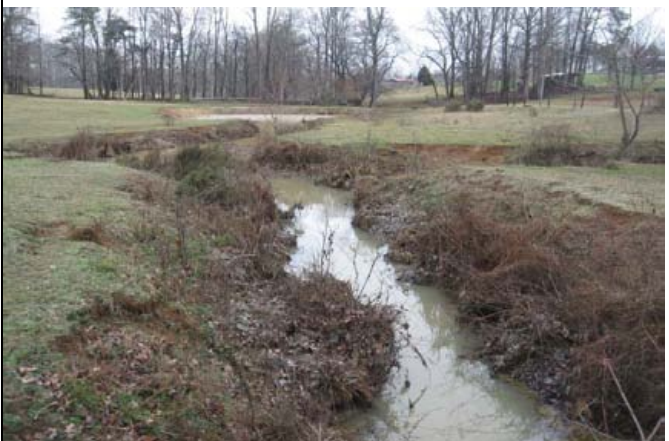
Reach T3 can be seen entering the right bank in the middle of this photo. A headcut from the mainstem has migrated through lower T3. (2/27/12)
