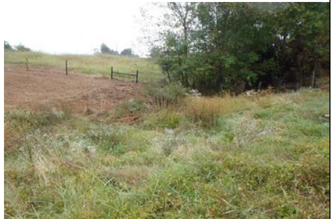
View looking upstream at the dam above Reach T2. (10/10/13)
