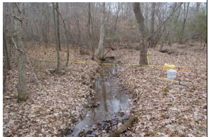
View looking upstream along reference reach cross section in Haw River State Park. (12/8/14)
