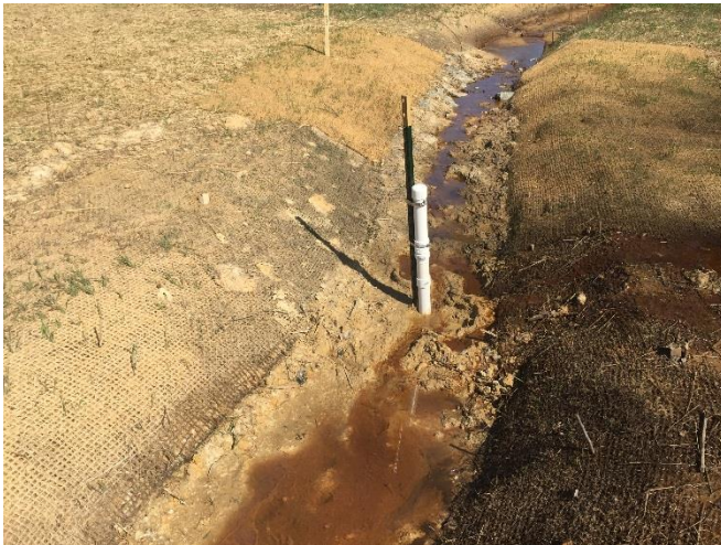
Automated Flow Gauge 2 – Reach T3
