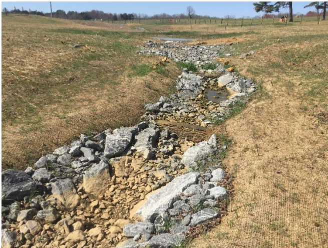
Photo Point 35 – Station 15+00, Reach 6, BMP
