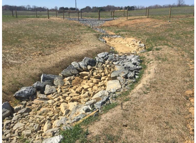
Photo Point 38 – Station 10+50, Reach 6, BMP
