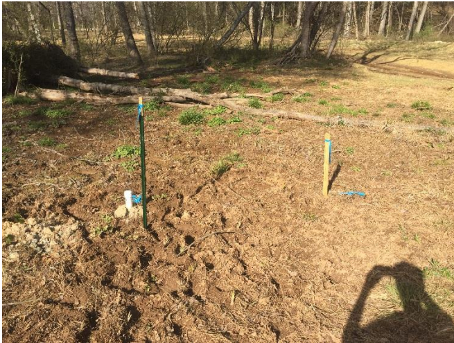
Wetland Well 3 – Reach 1, Station 52+00
