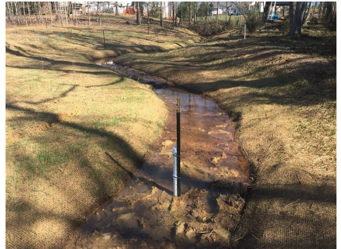
Automated Flow Gauge 3 – Reach T1
