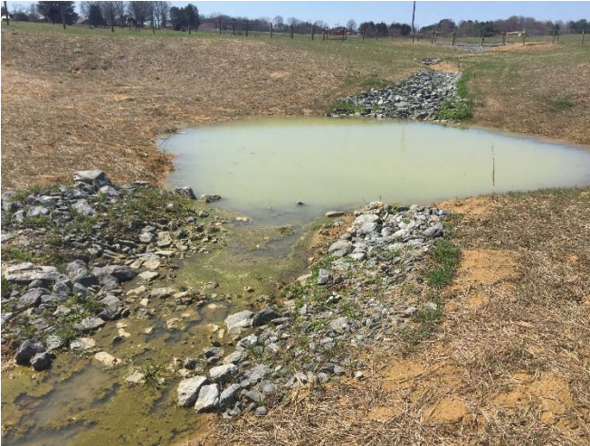
Photo Point 37 – Station 11+90, Reach 6, BMP
