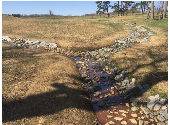
Photo Point 34 – Sta. 15+75, Reaches 4, 5 and 6
