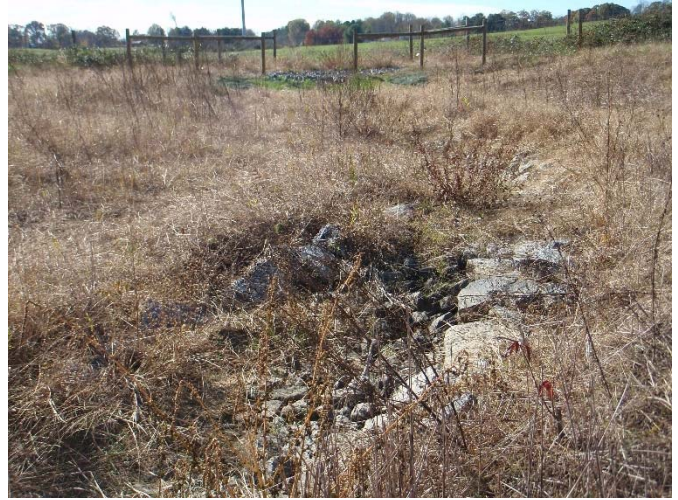
Photo Point 38 – Station 10+50, Reach 6, Step Pools
