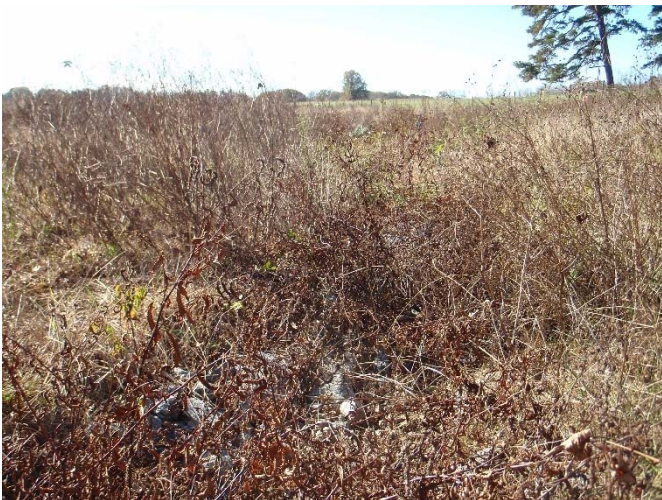
Photo Point 35 – Station 15+00, Reach 6, Step Pools
