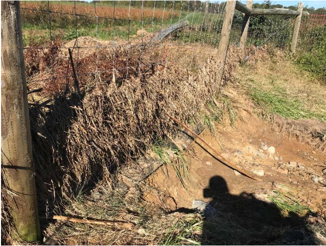
SPA 1 – Reach 6, Station 10+25
