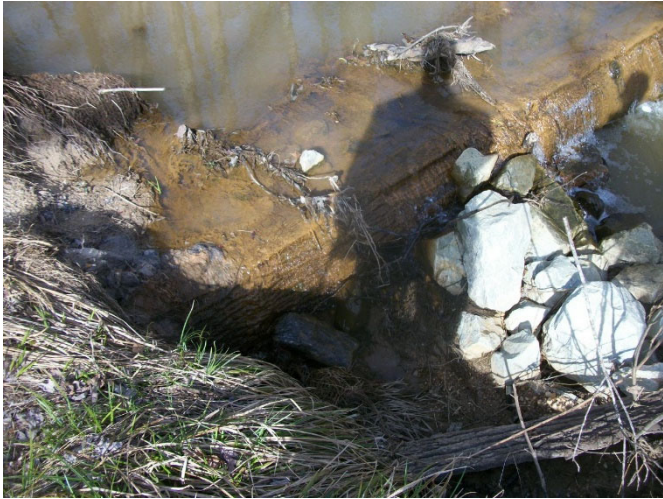
SPA 3-1 – Reach 2, Station 47+50 (March 12, 2019)
