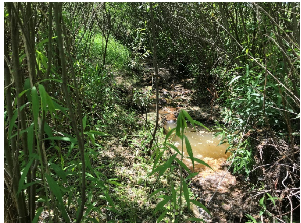
Photo Point 22 – Station 28+75, Reach 3/T3
