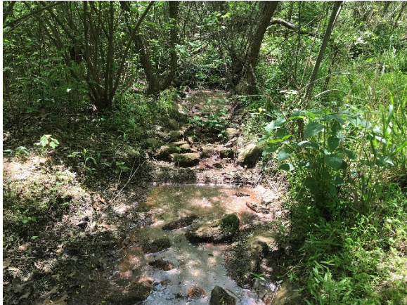
Photo Point 29 – Station 11+00, Reach T4
