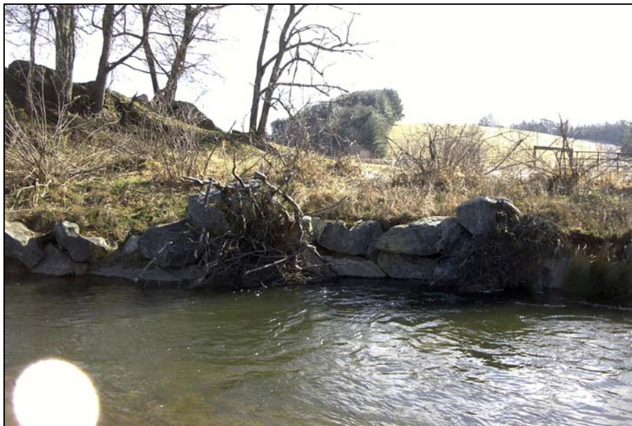
Brush Creek Photograph Station 3 120° from North
