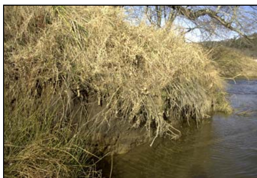
Undercut left stream bank at the confluence with Brush Creek
