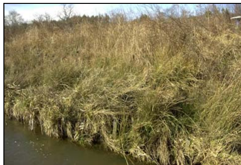
Tunneling in left bank near cross-section 3
