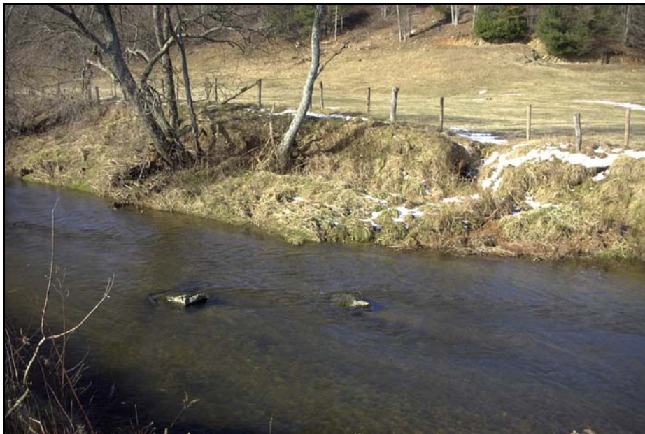
Brush Creek Photograph Station 1 275° from North
