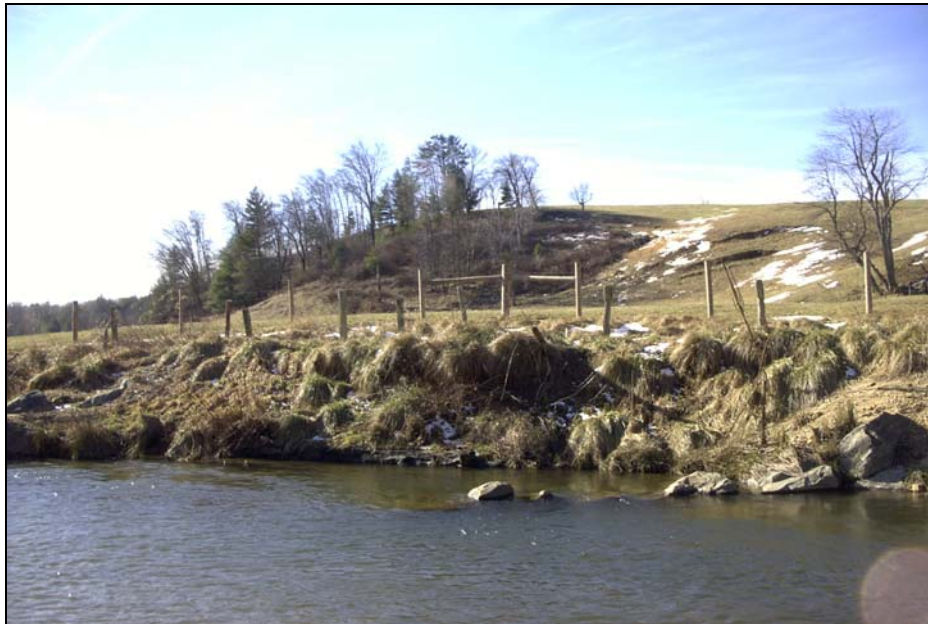
Brush Creek Photograph Station 9 230° from North
