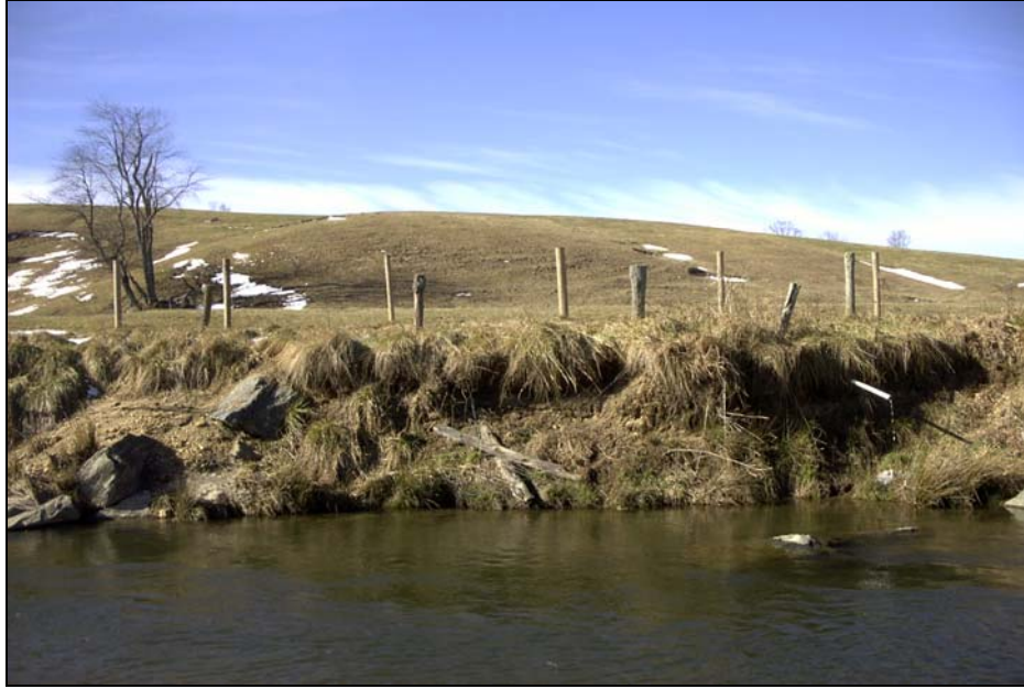
Brush Creek Photograph Station 9 270° from North
