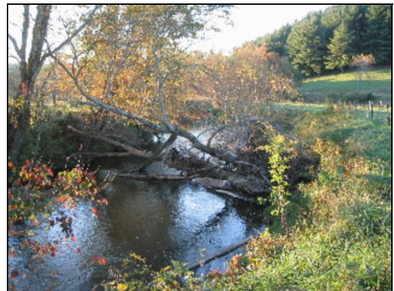
Issue Photo 2. Brush Creek near Station 5+00. Large Woody Debris in channel.
