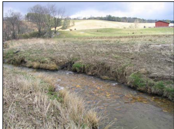
Issue Photo 4. Little Pine near station 6+00. Toe Scour along Right Bank
