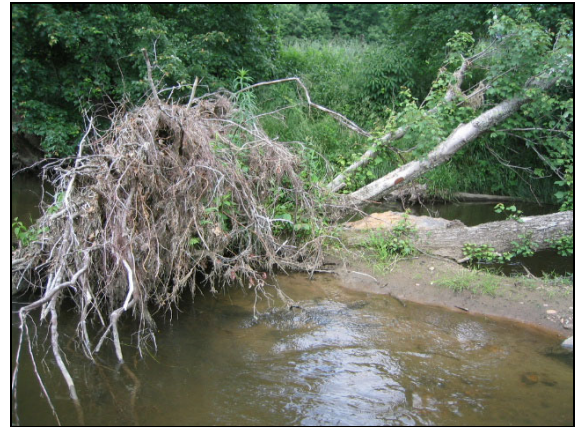
Issue Photo 2. Brush Creek near Station 0+50. Transverse bar at start of project.
