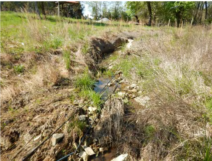
PHOTO POINT 35 T6 Reach 3 – upstream (4/7/2020)
