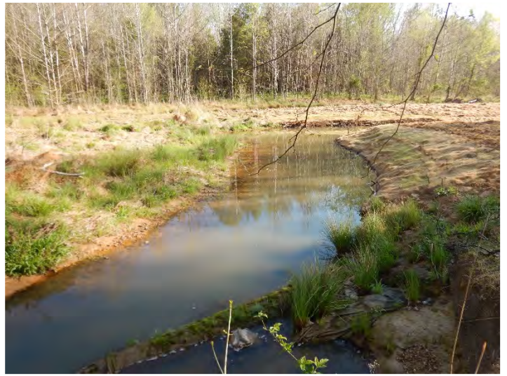
After - Repaired Localized Erosion (4/7/2020)
