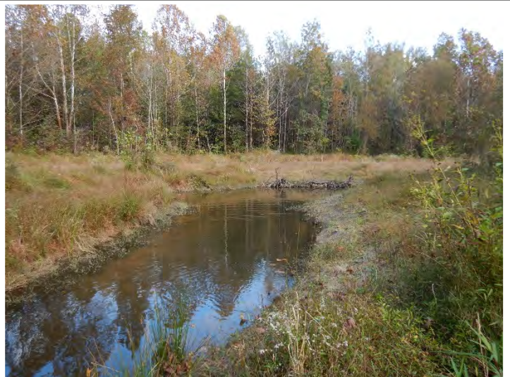
After - Repaired Localized Erosion (10/21/2020)
