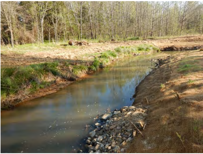
After - Repaired Localized Erosion (4/7/2020)
