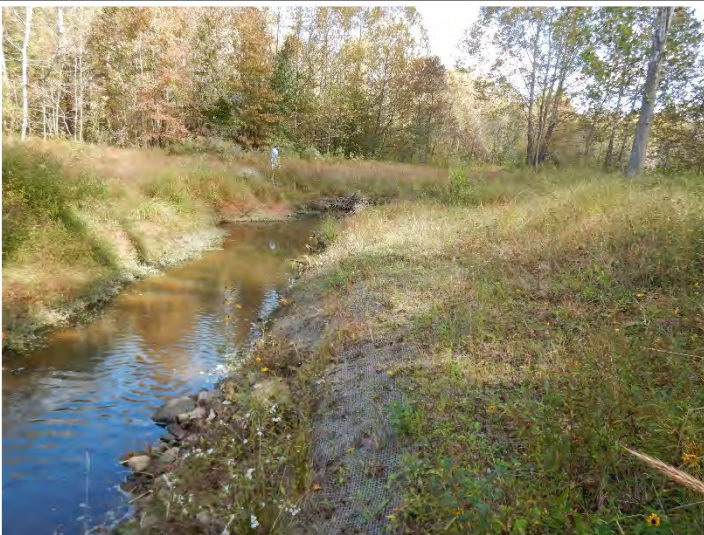
After - Repaired Localized Erosion (10/21/2020)
