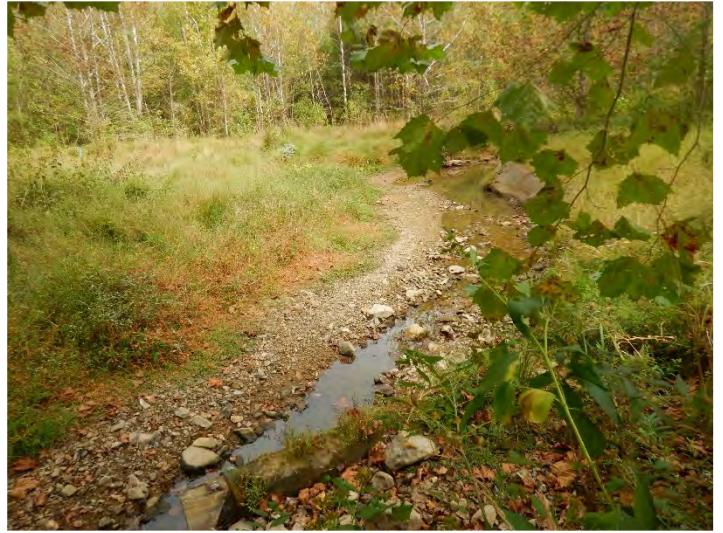
Before - Localized Erosion (10/9/2019)
