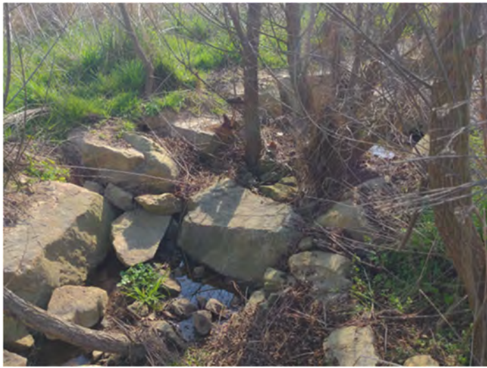
T4 STA 408+42 – 409+20 – Piping Rock Sills (3/24/2023)
