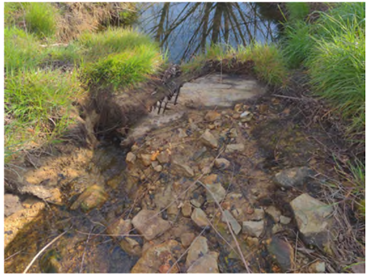
T3 R2 STA 314+40 - 314+70 – Piping Angled Log Riffle (3/24/2023)
