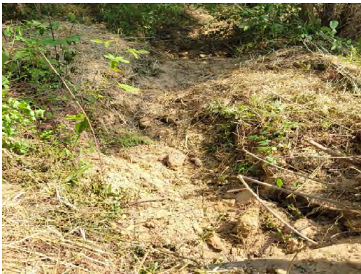
T6 R3 STA 517+80 – 518+20 – Repaired Area (8/22/2023)
