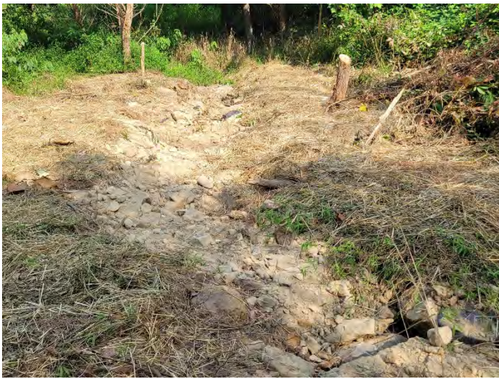
T4B R1 STA 451+40 – 451+70 – Repaired Area (8/22/2023)
