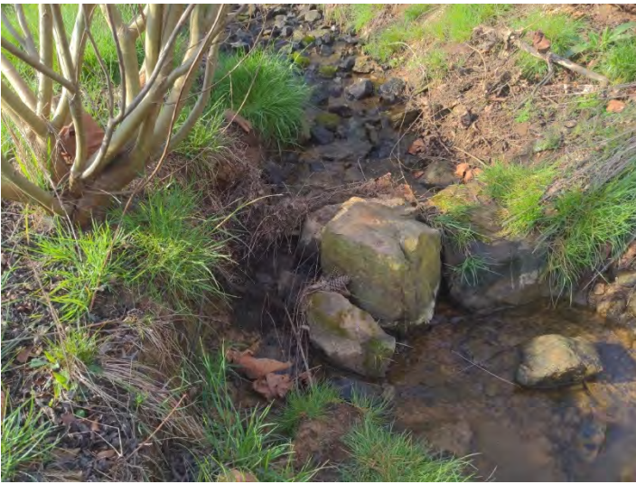
T3 R2 STA 314+20 - 314+30 – Piping Rock Sill (3/24/2023)
