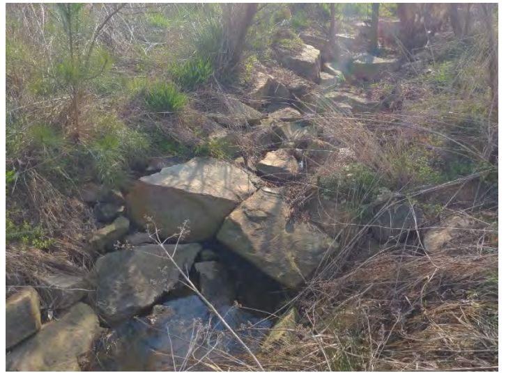
T4 STA 408+42 – 409+20 – Piping Rock Sills (3/24/2023)
