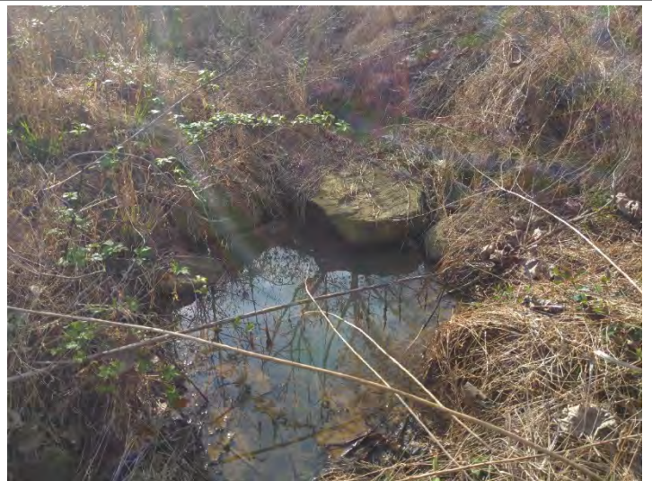
T4B R1 STA 451+40 – 451+70 – Piping Rock Sills (3/24/2023)
