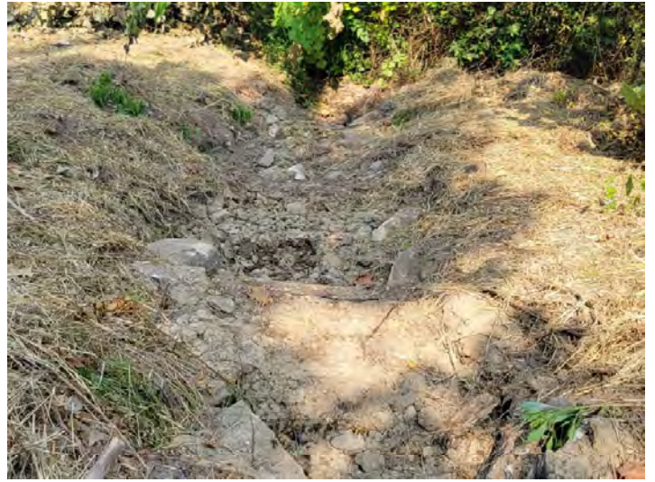
T4B R1 STA 453+00 – 453+50 – Repaired Area (8/22/2023)
