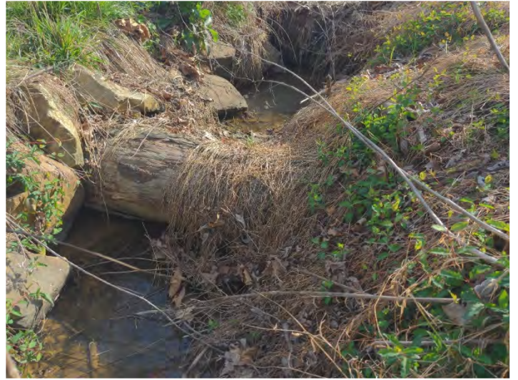
T4B R1 STA 453+00 – 453+50 – Piping Log and Rock Sills (3/24/2023)
