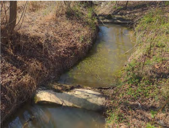
T6 R3 STA 517+80 – 518+20 – Piping Log Sills (3/24/2023)
