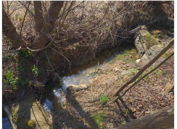
T6 R3 STA 517+80 – 518+20 – Piping Log Sills (3/24/2023)
