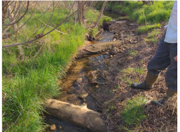
T3 R2 STA 314+40 - 314+70 – Piping Angled Log Riffle (3/24/2023)
