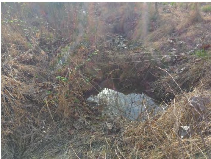
T4B R1 STA 451+40 – 451+70 – Piping Rock Sills (3/24/2023)
