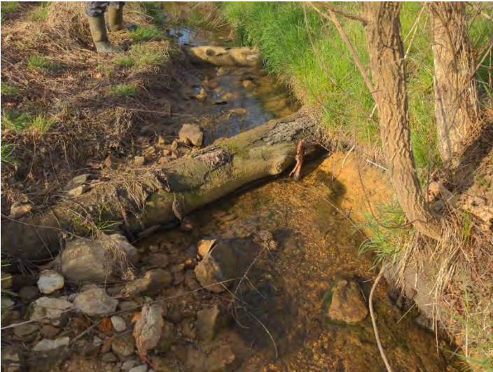
T3 R2 STA 314+40 - 314+70 – Piping Angled Log Riffle (3/24/2023)
