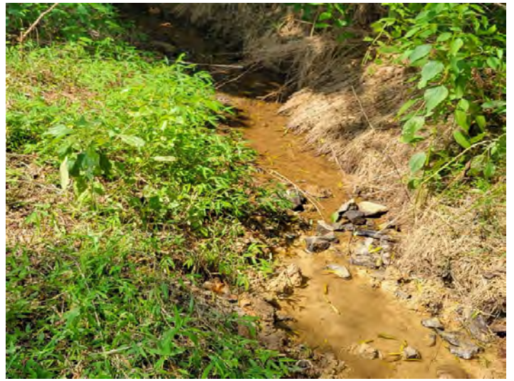
T3 R2 STA 314+20 – 314+30 – Repaired Area (8/22/2023)
