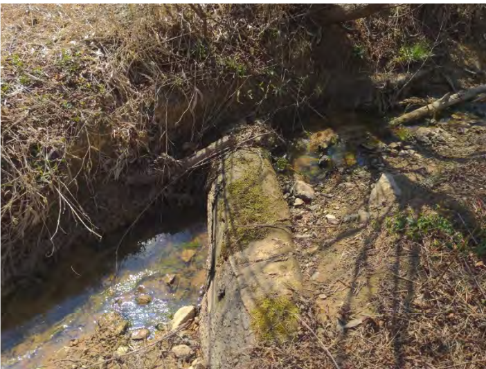
T6 R3 STA 517+80 – 518+20 – Piping Log Sills (3/24/2023)
