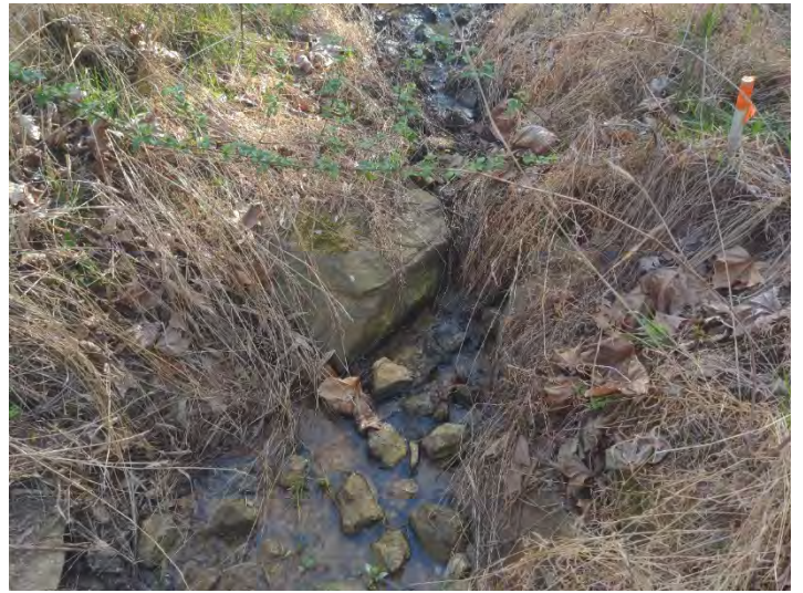
T4B R1 STA 451+40 – 451+70 – Piping Rock Sills (3/24/2023)
