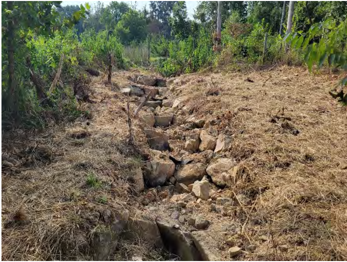
T4 STA 408+42 – 409+20 – Repaired Reach (8/22/2023)
