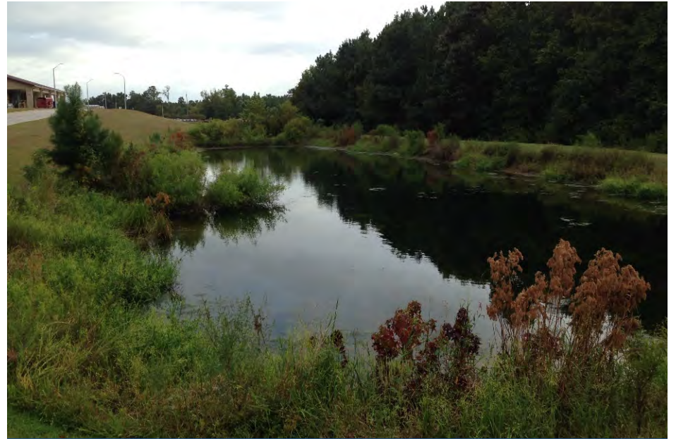
Stormwater BMP 2 at Corinth Holders High School
