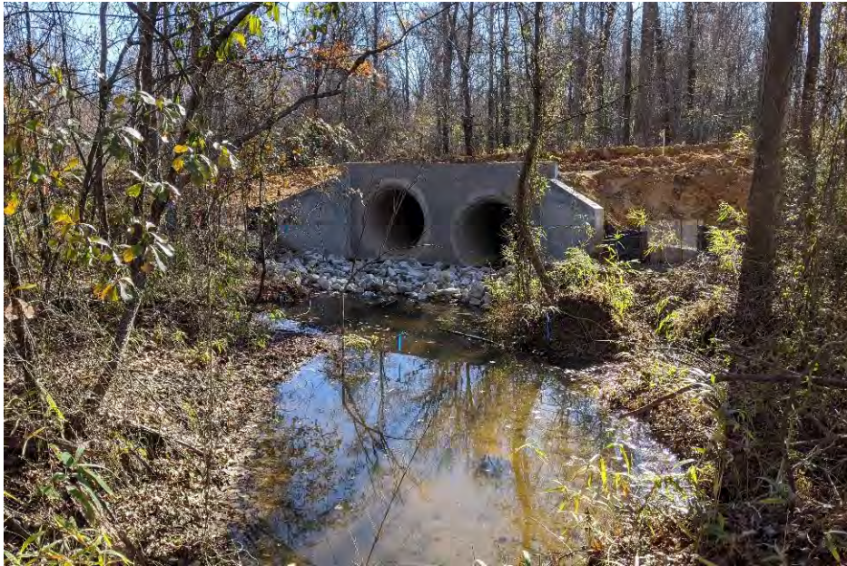
Reach MS-R2 – Upstream of newly installed culvert
