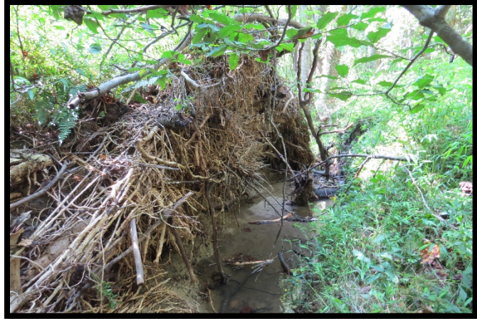
Photo illustrates active bank erosion and degraded wetland area along lower R5.
