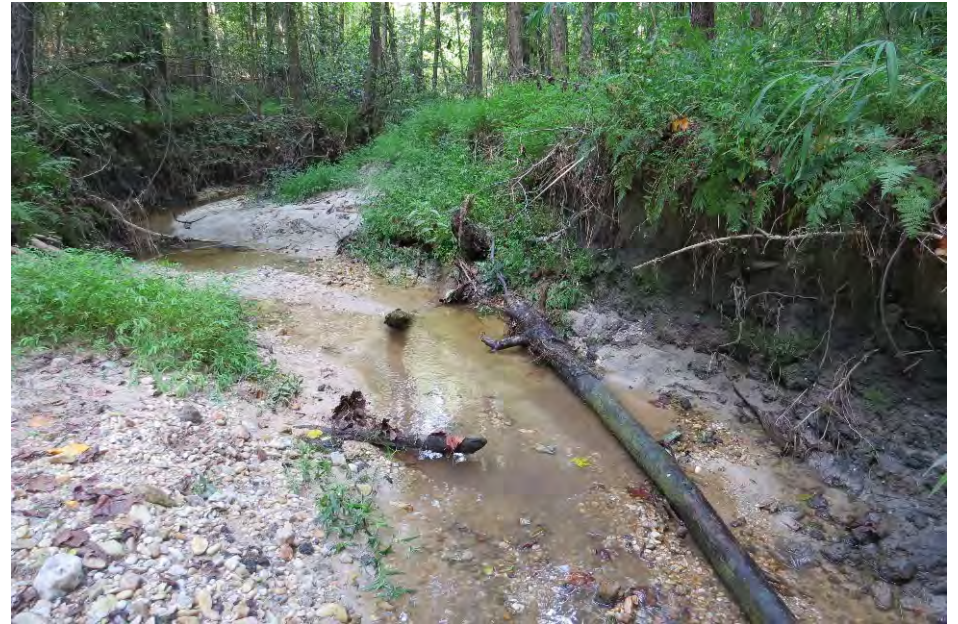
Reach MS-R1 – Stream incision and bank erosion
