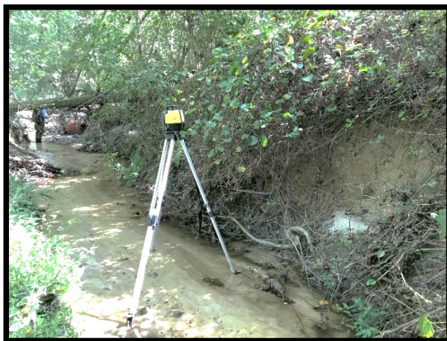
Looking downstream at lateral instability and stream bank erosion along MS-R2.
