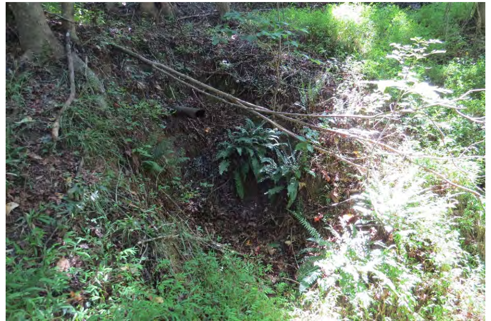
Reach R4 – Outfall pipe from historic farm pond
