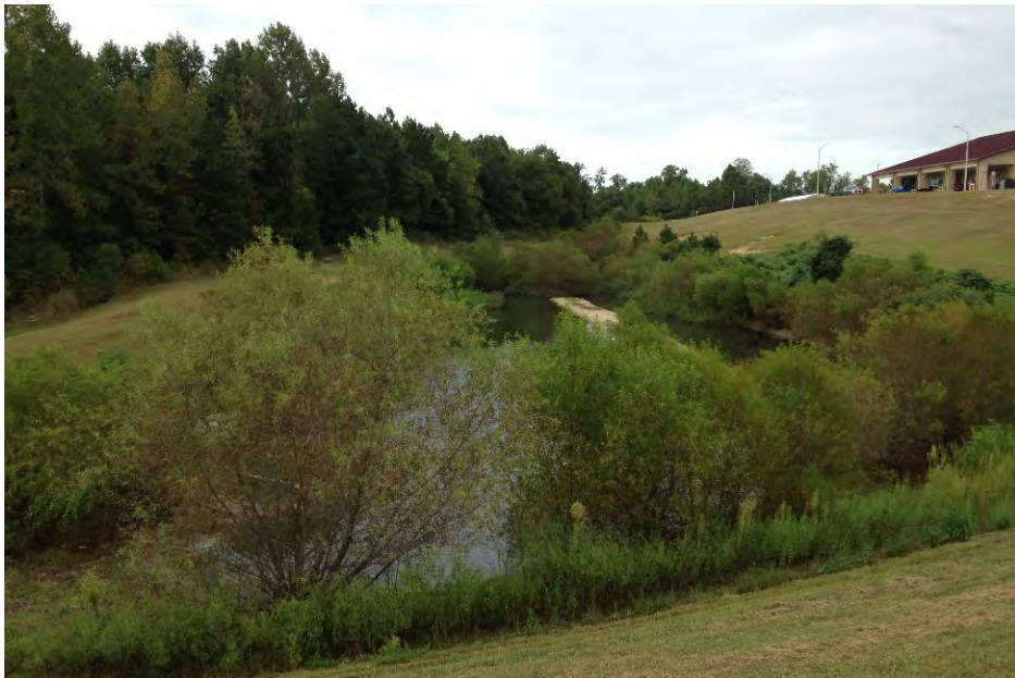
Stormwater BMP 1 at Corinth Holders High School
