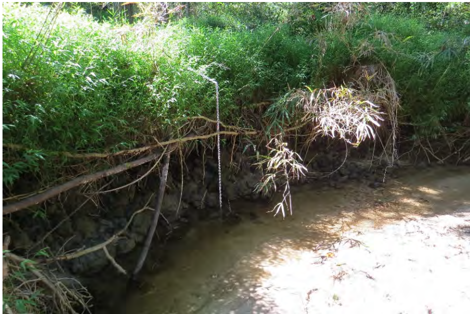
Reach MS-R2 – Stream incision and bank erosion
