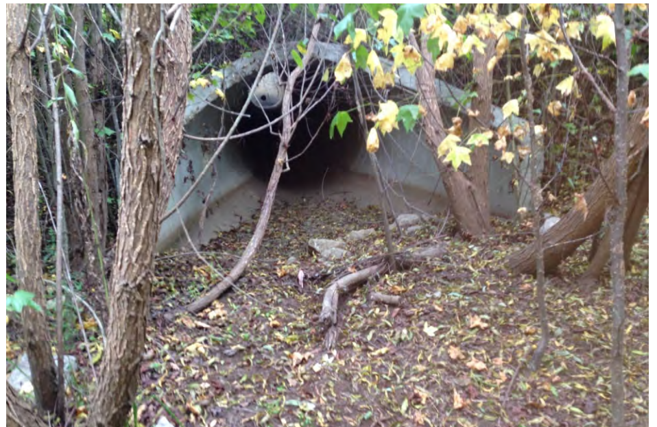
Stormwater outfall pipe of BMP 1
