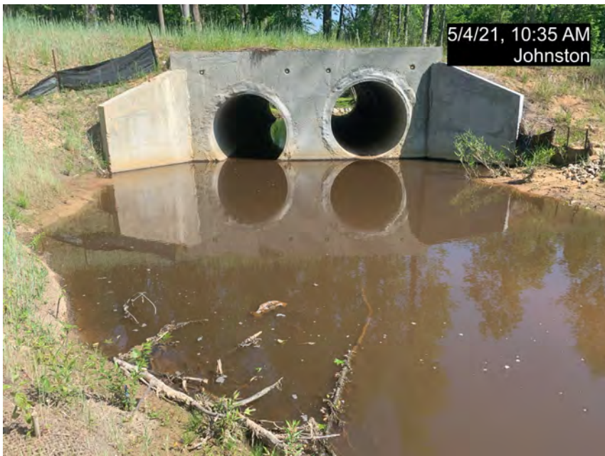
PS-2 – MS-R2 Culvert Crossing, Upstream (MY-00)
