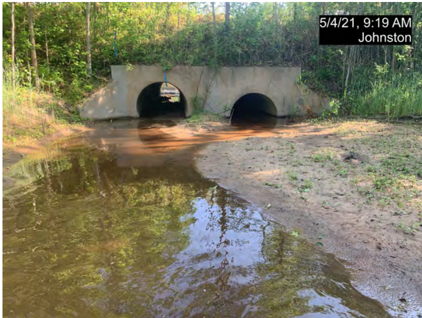
PS-1 – MS-R1 Culvert Crossing, Upstream (MY-00)
