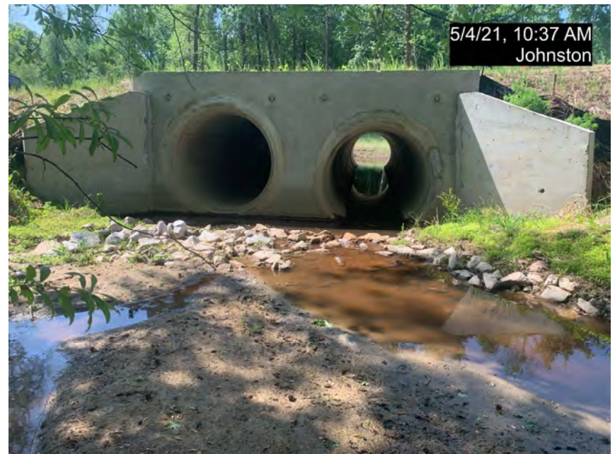
PS-2 – MS-R2 Culvert Crossing, Downstream (MY-00)
