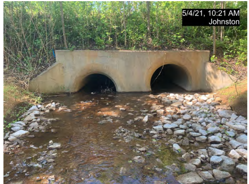
PS-1 – MS-R1 Culvert Crossing, Downstream (MY-00)
