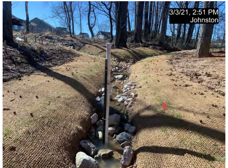
Flow Gauge (FG-2) – R6
