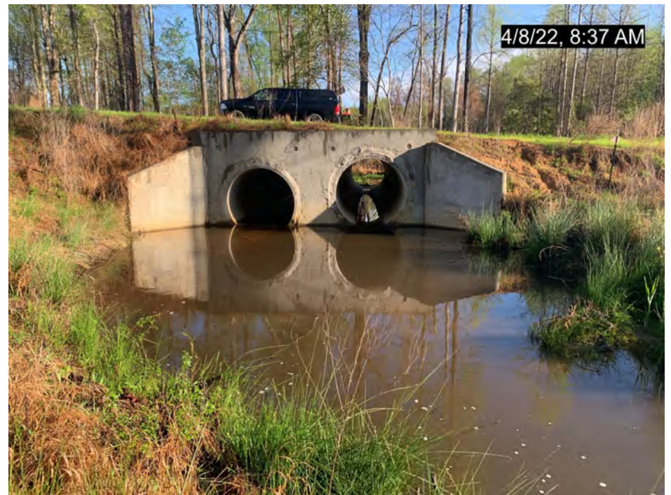
PS-2 – MS-R2 Culvert Crossing, Upstream (MY-02)
