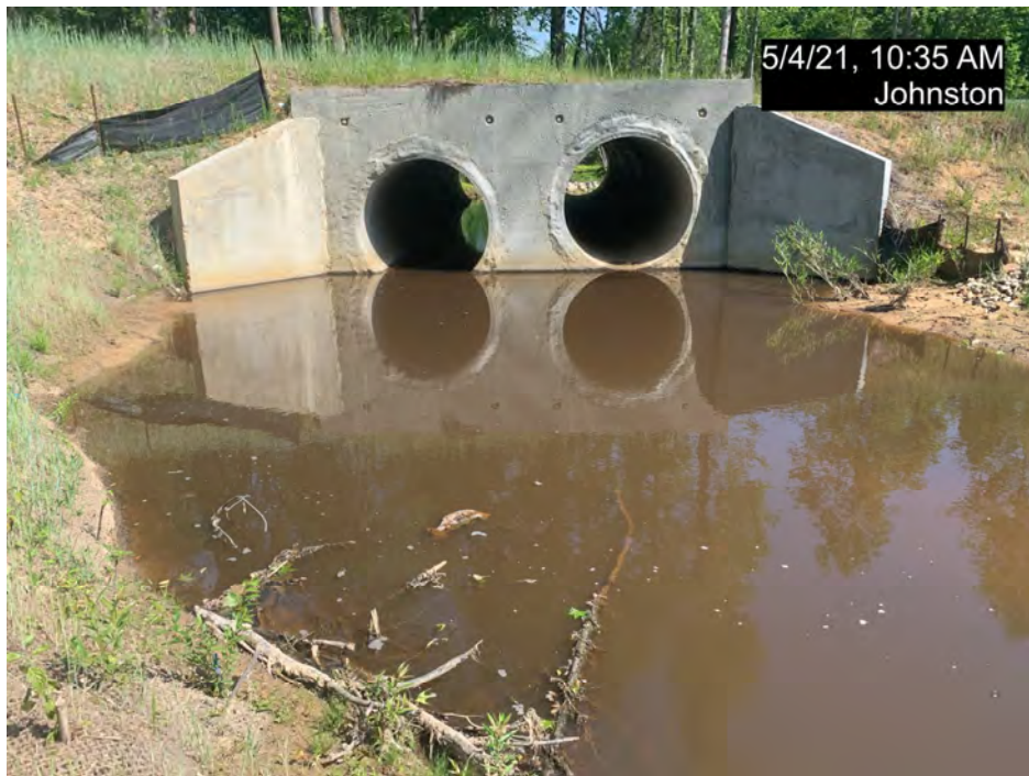
PS-2 – MS-R2 Culvert Crossing, Upstream (MY-00)
