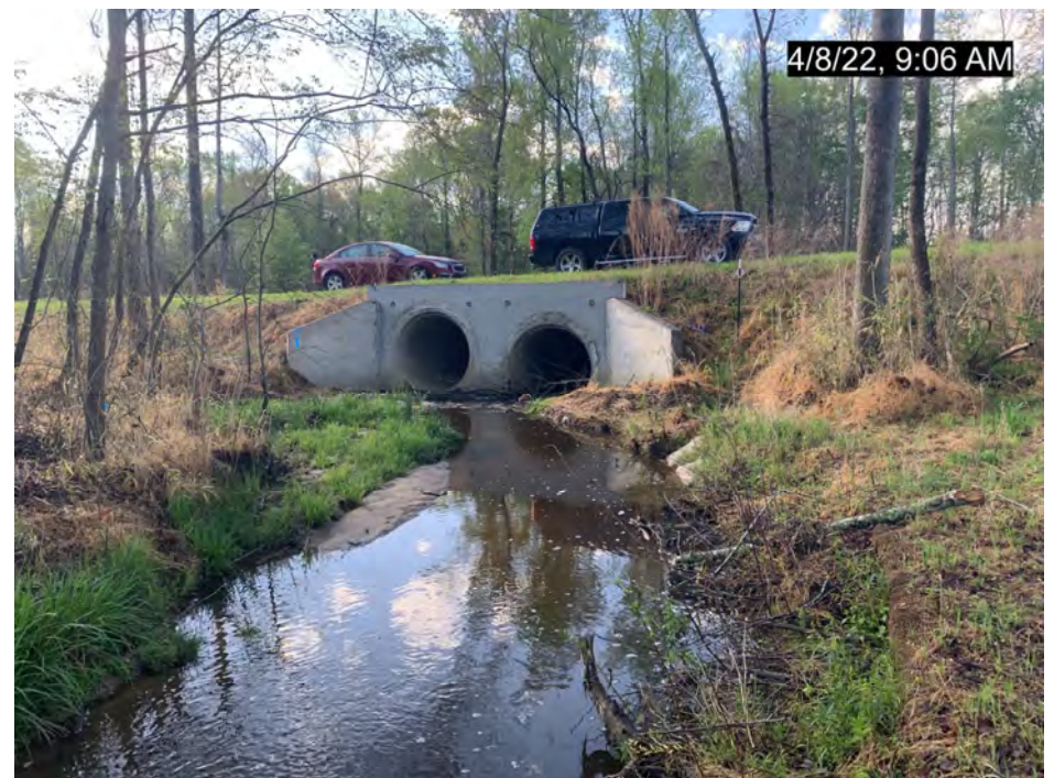
PS-2 – MS-R2 Culvert Crossing, Downstream (MY-02)
