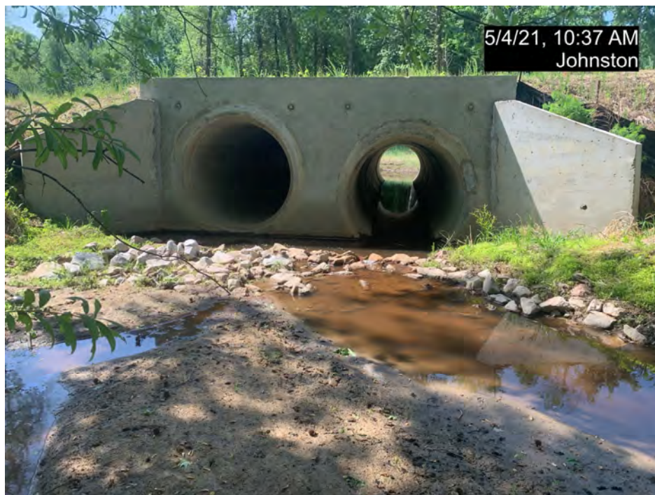
PS-2 – MS-R2 Culvert Crossing, Downstream (MY-00)
