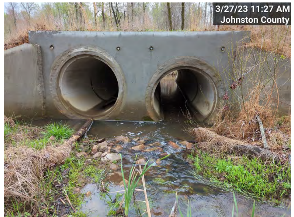
PS-2 – MS-R2 Culvert Crossing, Downstream (MY-03)
