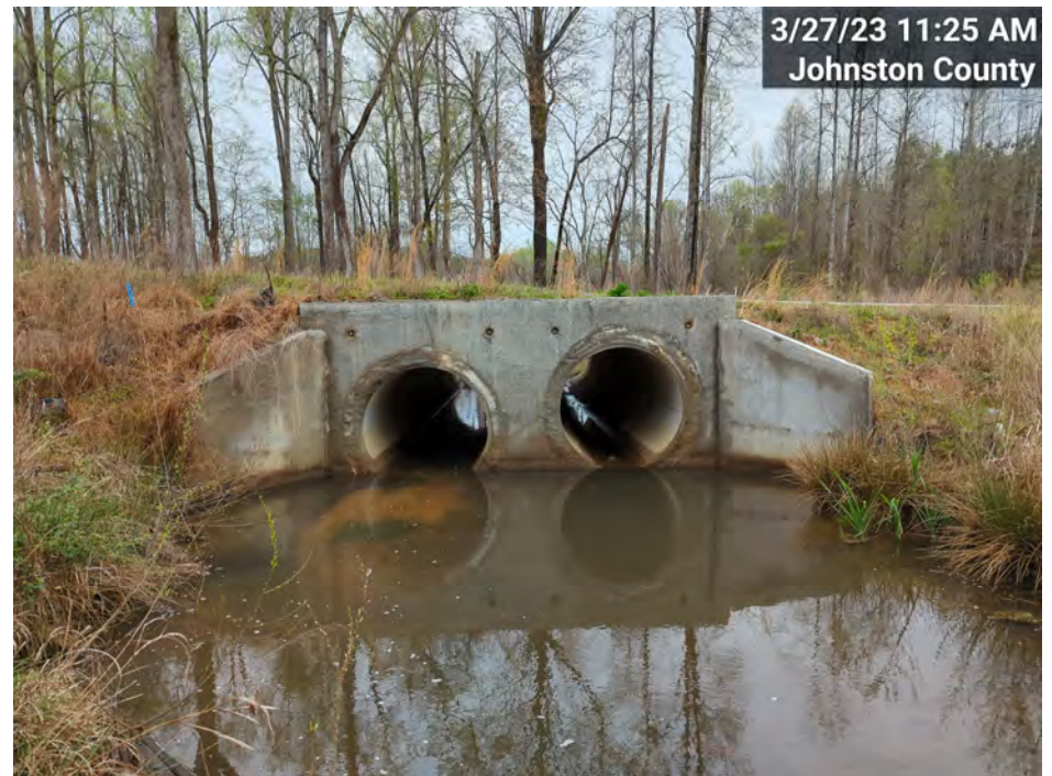
PS-2 – MS-R2 Culvert Crossing, Upstream (MY-03)
