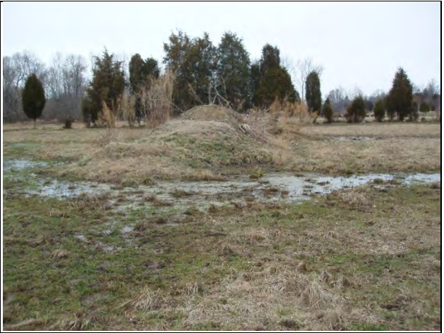
Spoil remaining from the pond construction. 3/2/2010
