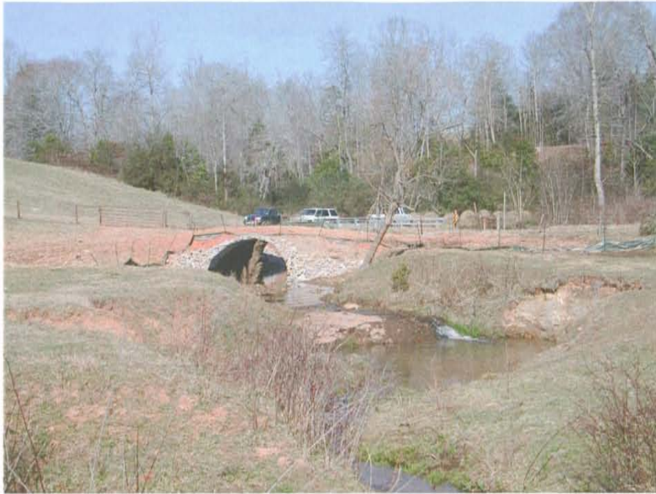
Picture 11. Existing bridge to be replaced.
