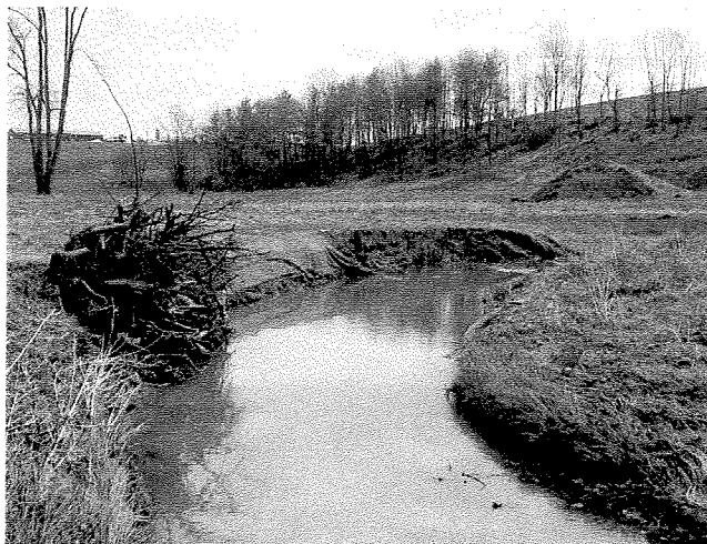
Lack of vegetation to hold the bank together.
