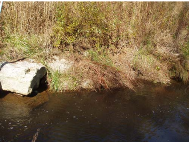
PA27 facing left bank
