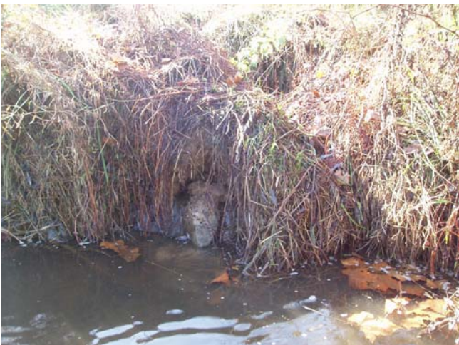
PA21 facing right bank
