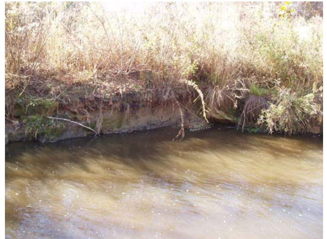
PA38 facing right bank
