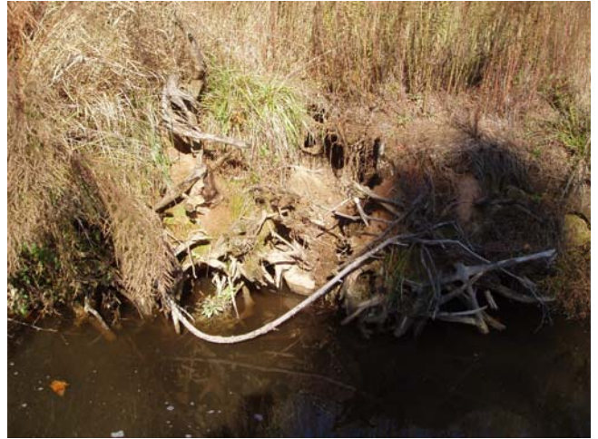
PA24 facing left bank
