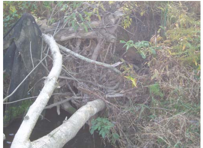
PA8 facing right bank
