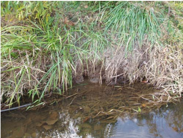
PA7 facing right bank
