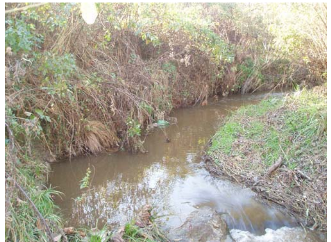
UTPA18 facing upstream
