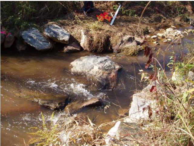
PA37 facing upstream at junction with UT
