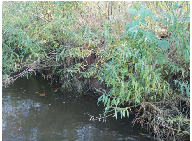
PA22 facing left bank
