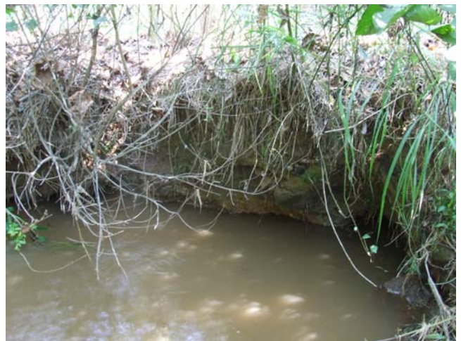
UTPA22 facing left bank
