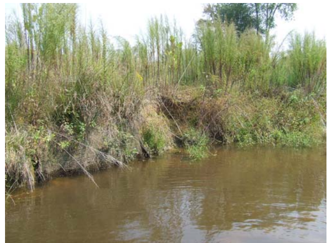
PA10 facing downstream
