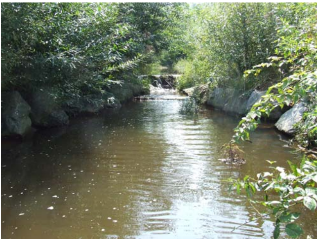
PA19 facing downstream
