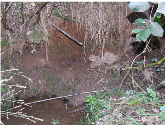
UTPA7 facing left bank
