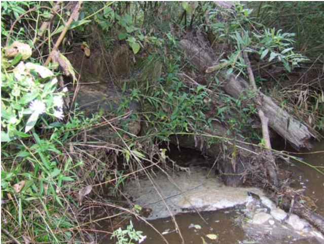
UTPA5 facing downstream
