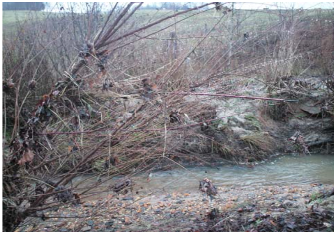
Facing Left Bank
