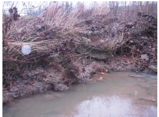
PA41 facing left bank
