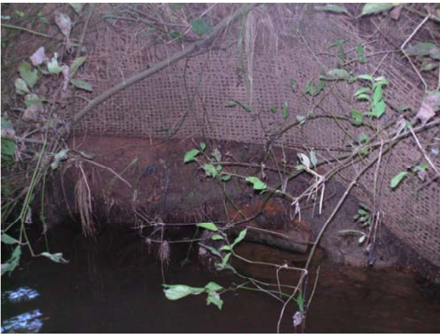
UTVPA3 facing right bank (9/4/08)
