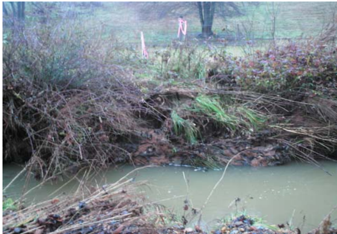
Facing Left Bank
