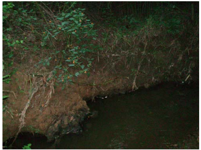
UTVPA4 facing left bank, upstream (9/4/08)
