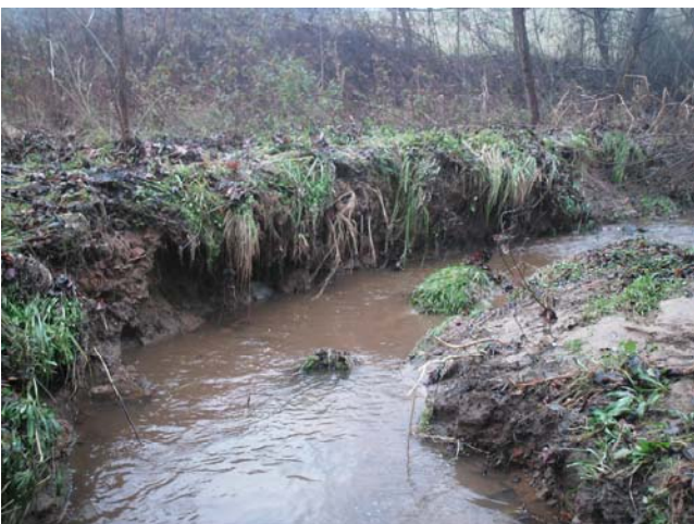
UTPA17 facing downstream
