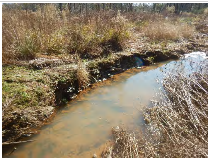
Before – Localized Toe Erosion (11/17/2022)
