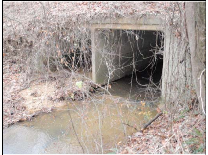
Box culvert under River Siloam Rd
